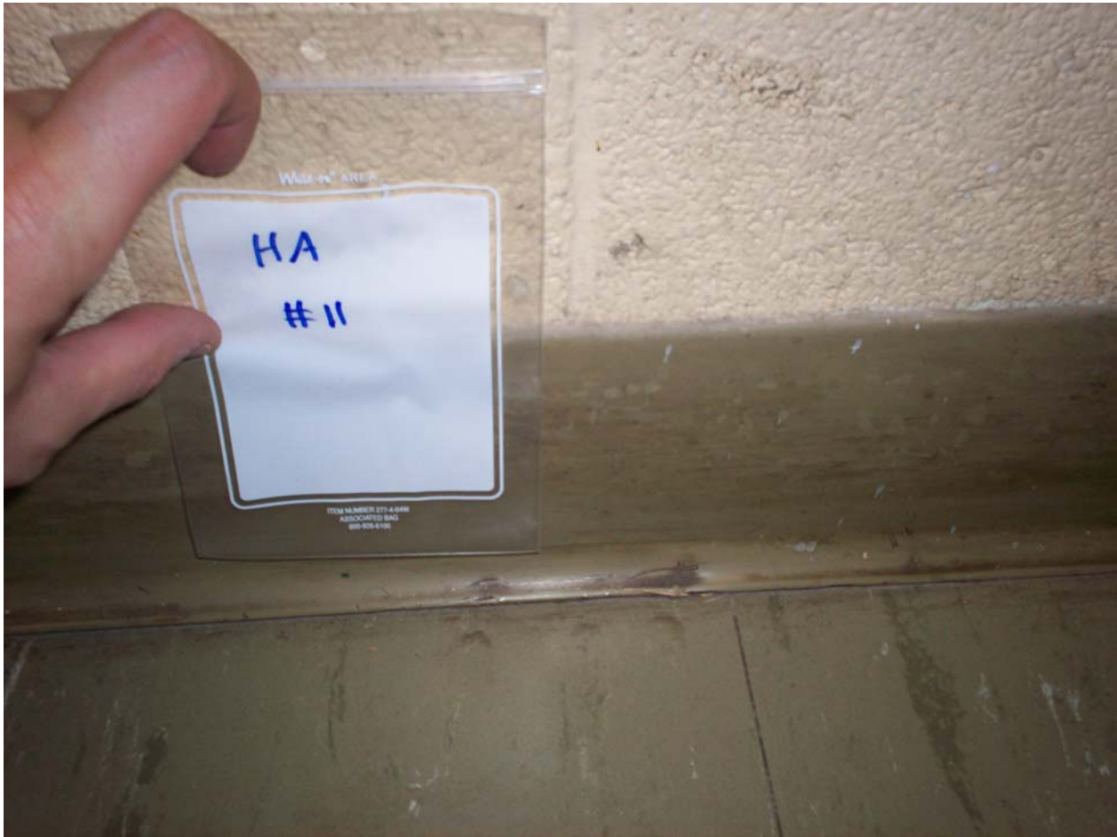
HA #11 – Non asbestos containing 4” green cove molding and associated mastic
