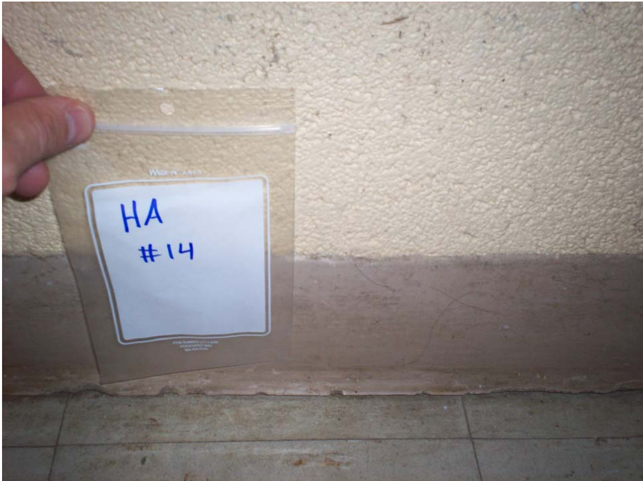
HA #14 – Non asbestos containing 4” tan cove molding and associated mastic
