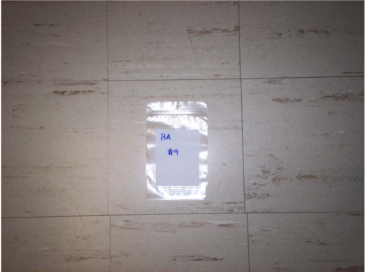
HA #9 – Asbestos containing 9” x 9” cream floor tile with white and brown streaks and associated non asbestos containing mastic
