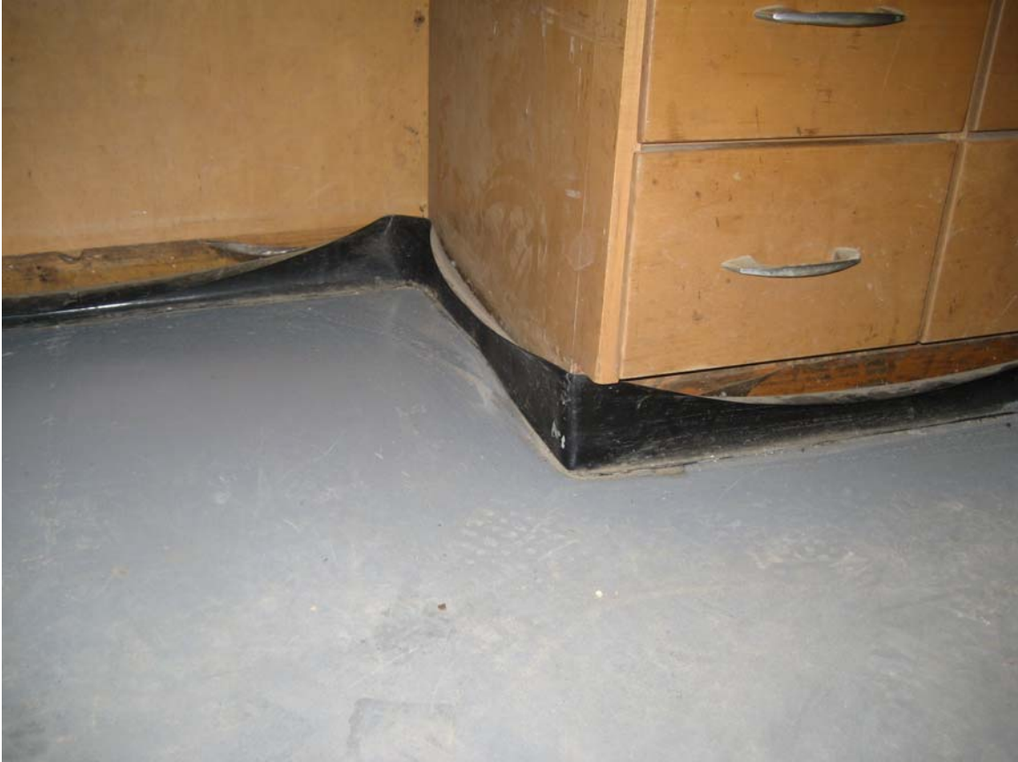
HA #4 – Non asbestos containing 4” black cove molding and associated mastic
