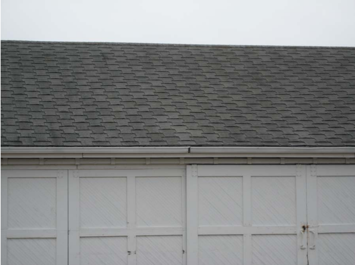
HA #2 – Non-asbestos containing gray shingles and associated products
