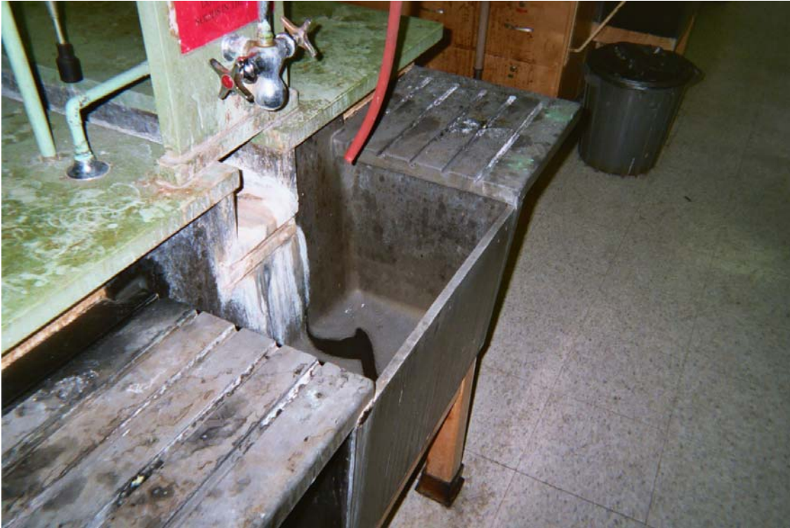
Photo 8 – Non-asbestos containing black lab sink and table tops
