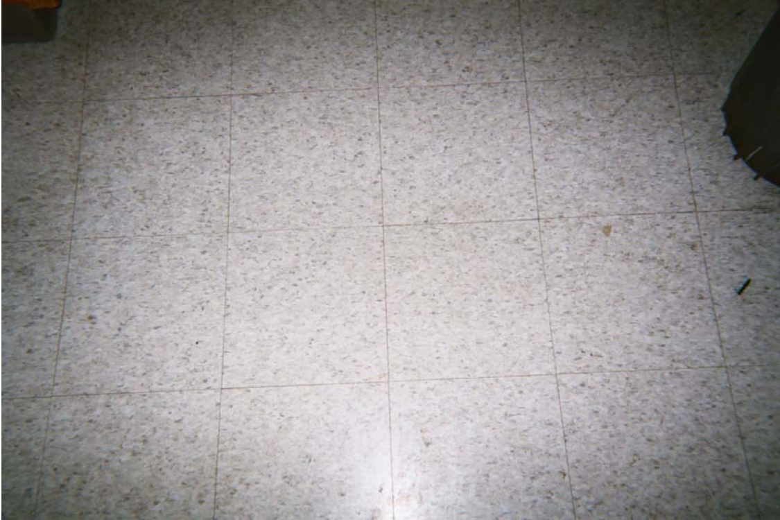
Photo 10 – Non-asbestos containing 12” x 12” cream marble pattern floor tile and associated mastic
