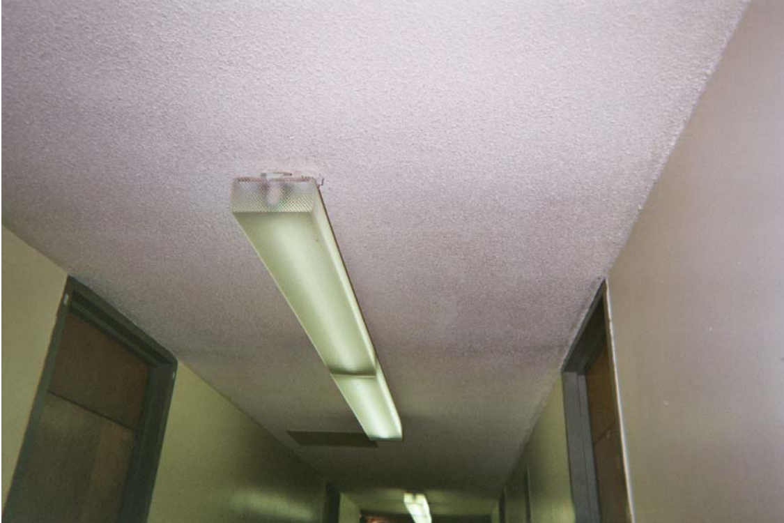
Photo 14 – Non asbestos-containing spray-in acoustical plaster
