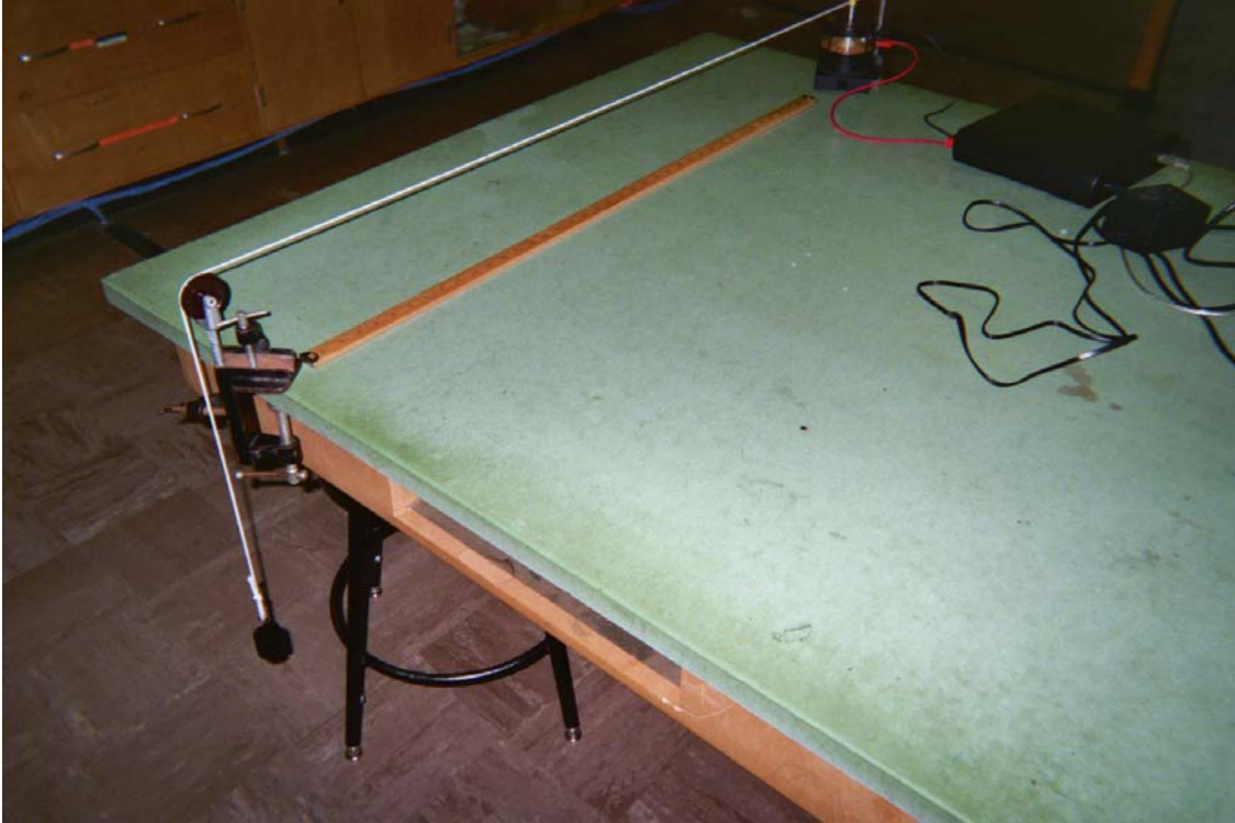
Photo 7 – Asbestos-containing green lab table
