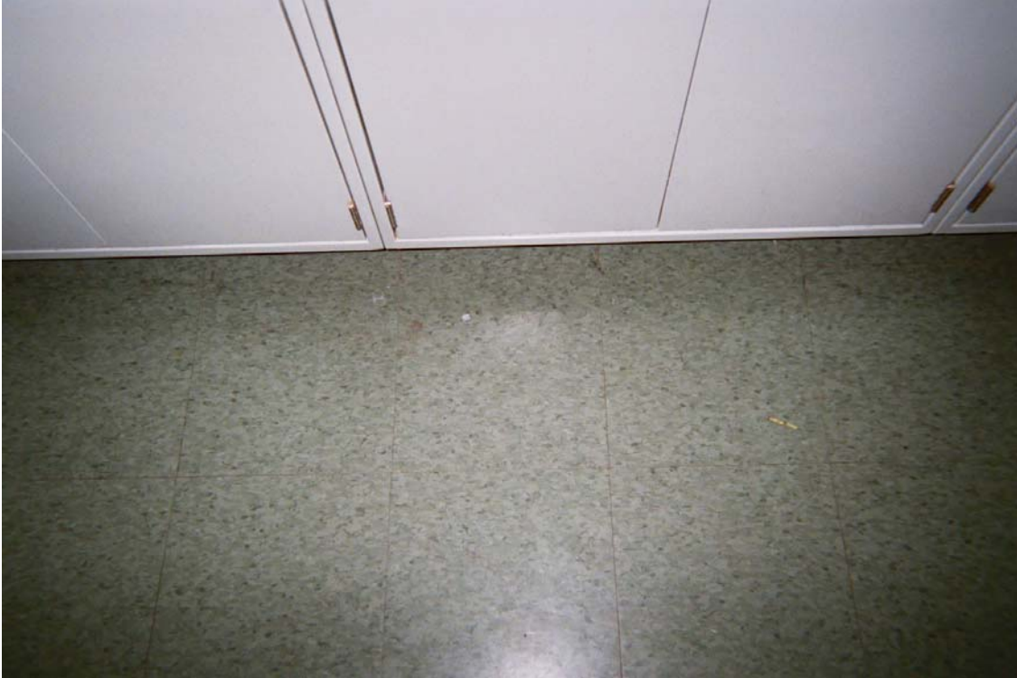
Photo 9 – Non-asbestos containing 12” x 12” green marble pattern floor tile and associated mastic
