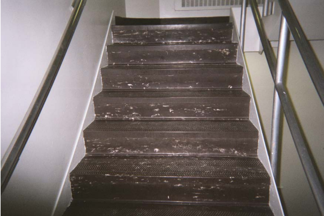
Photo 15 – Non asbestos-containing 2' x 2' brown linoleum and stair tread with cream swirls and associated mastic
