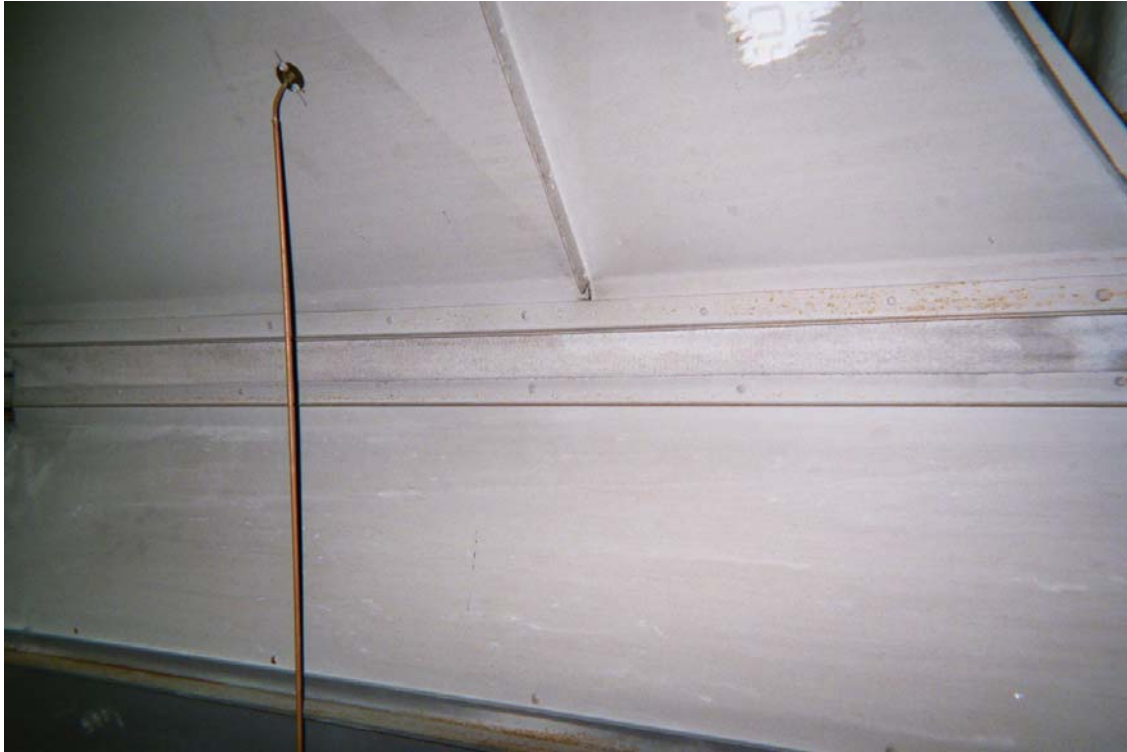
Photo 3 – Asbestos-containing ventilation duct expansion cloth
