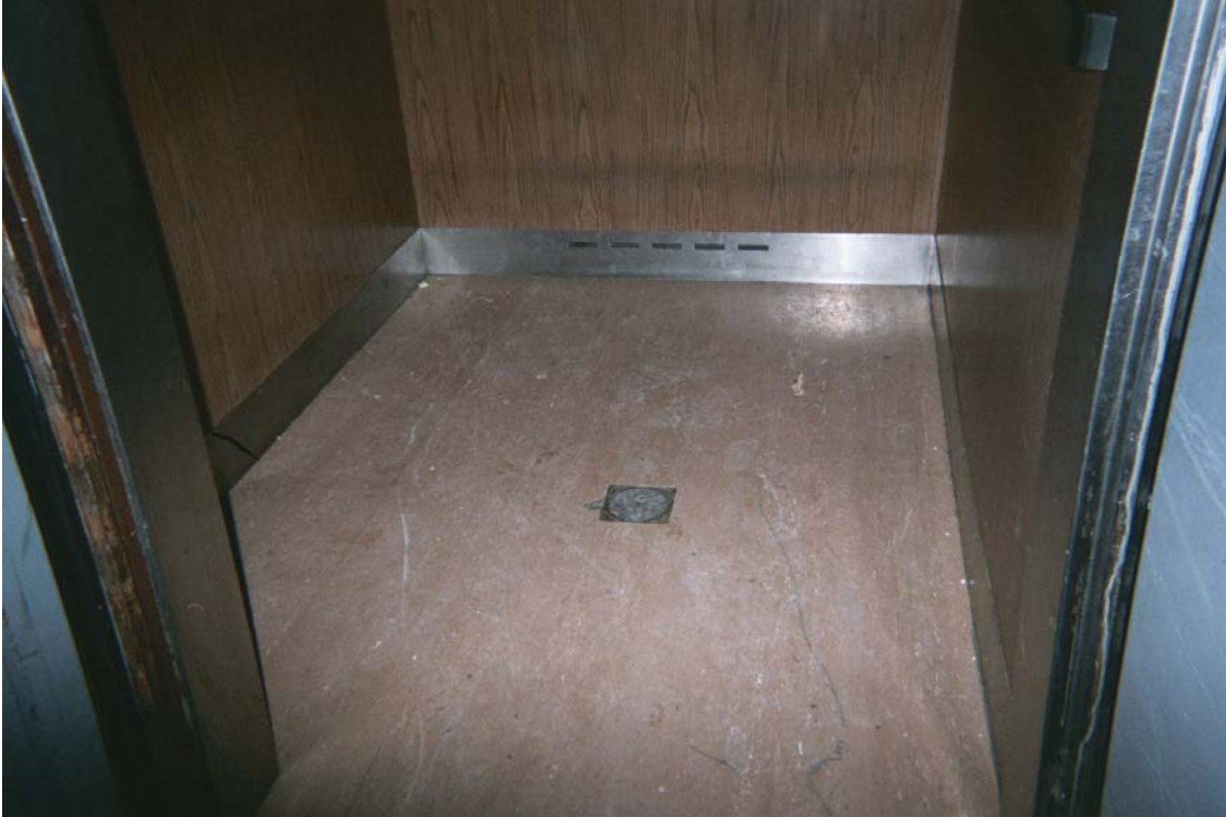
Photo 17 – Non asbestos-containing tan linoleum with cream streaks and associated mastic
