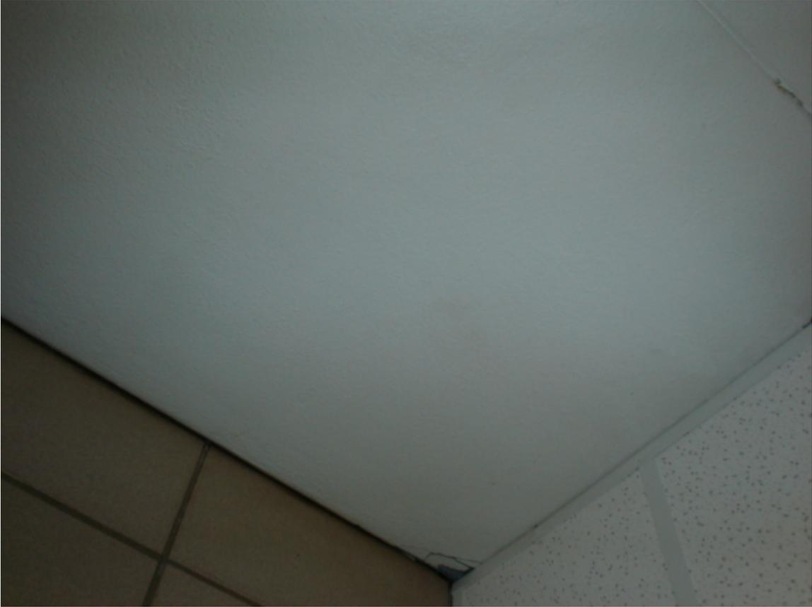
HA #1 – Non asbestos-containing ceiling plaster
