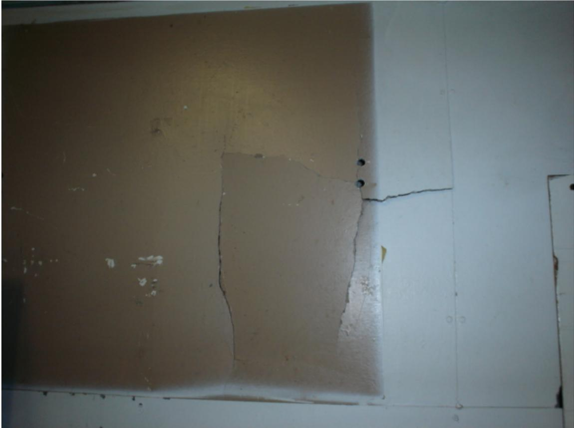
HA #15 – Significantly damaged asbestos-containing transite paneling
