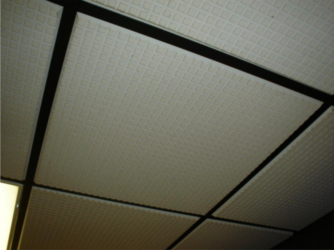
HA #12 – Non asbestos-containing 2' x 2' white drop-in ceiling tile
