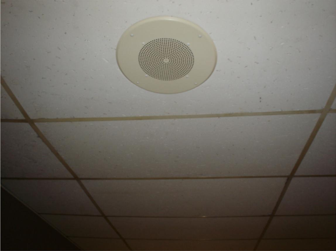
HA #19 – Non asbestos-containing 2' x 4' white lay-in ceiling tile with pin holes and fissures
