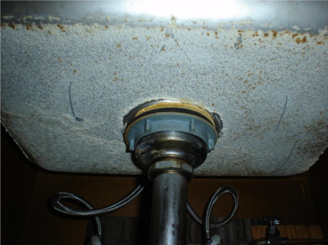
HA #17 – Asbestos-containing white sink undercoating
