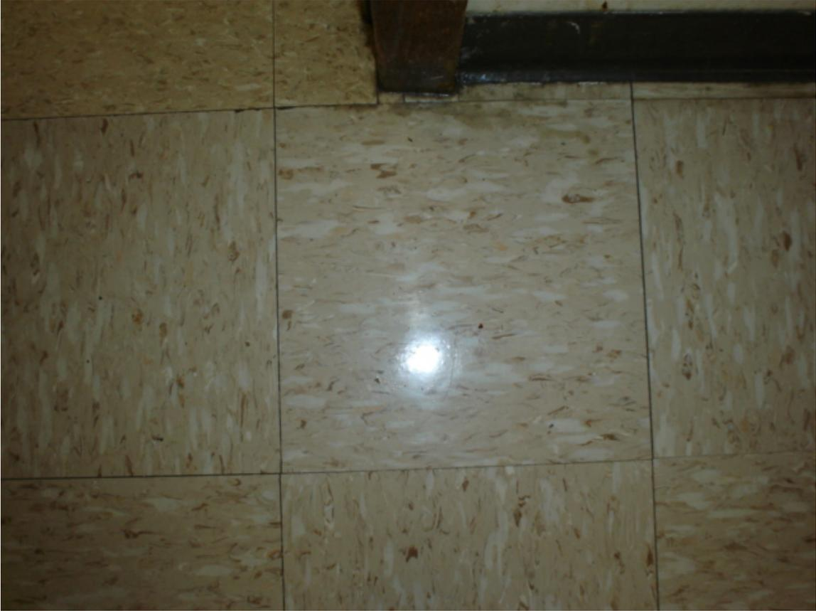
HA #16 – Non asbestos-containing 12" x 12" tan floor tile with cream and brown specks and associated mastic
