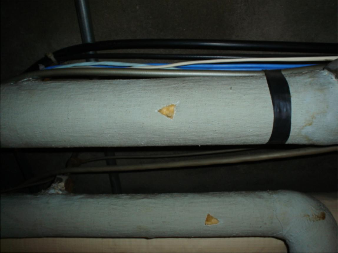
HA #13 – Non asbestos-containing canvas wrap on fiberglass pipe straight insulation
