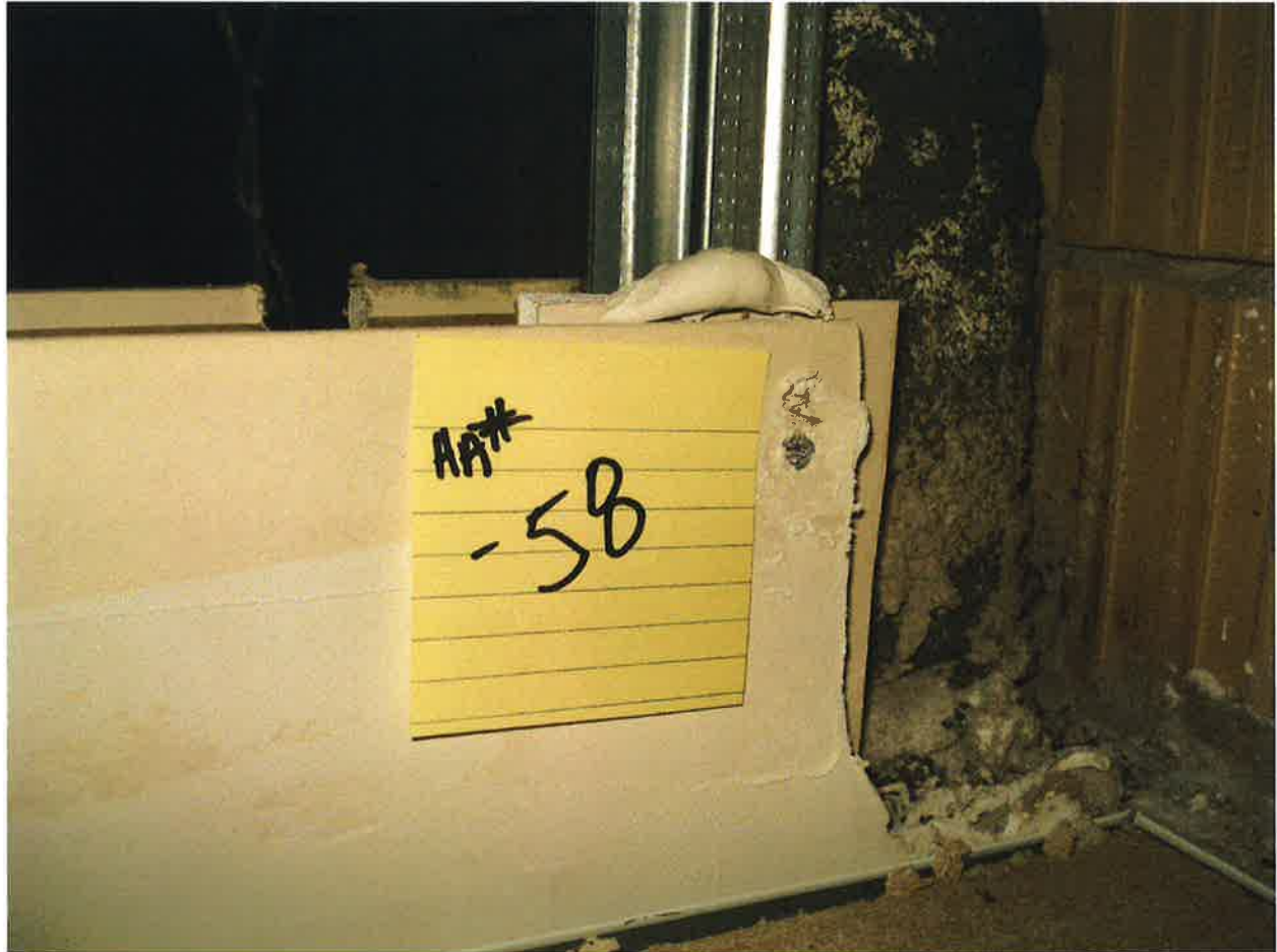
HA #58 – Non asbestos containing drywall joint compound
