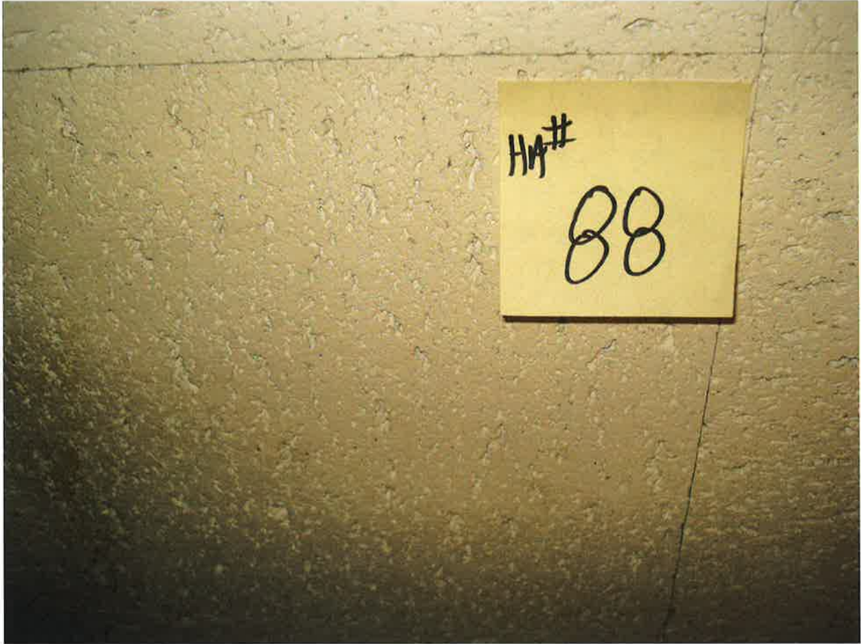
HA #88 – Non asbestos containing 12” x 12” white ceiling tile with fissures and associated glue pods
