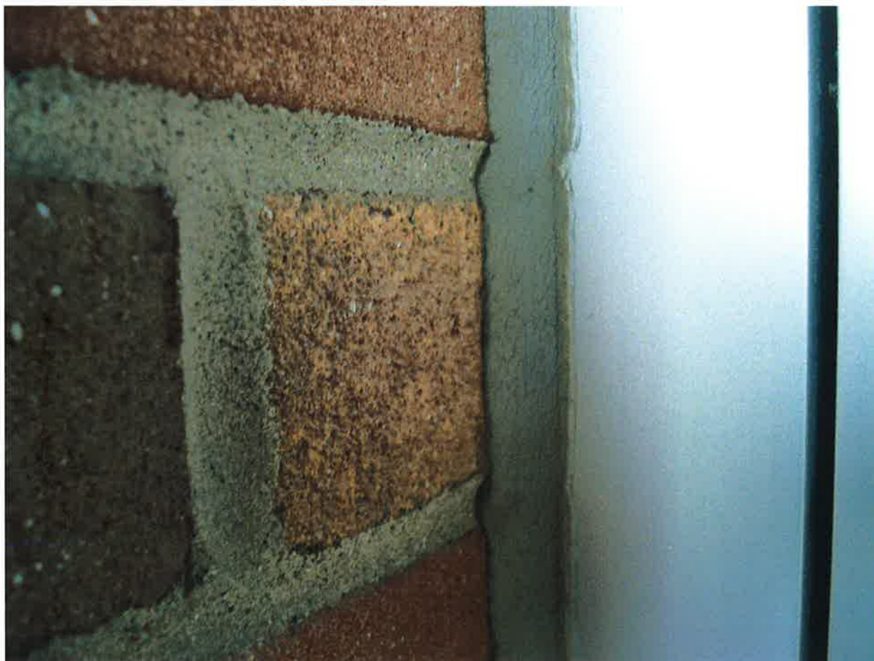
HA #34 – Non asbestos containing gray window and door frame caulk compound
