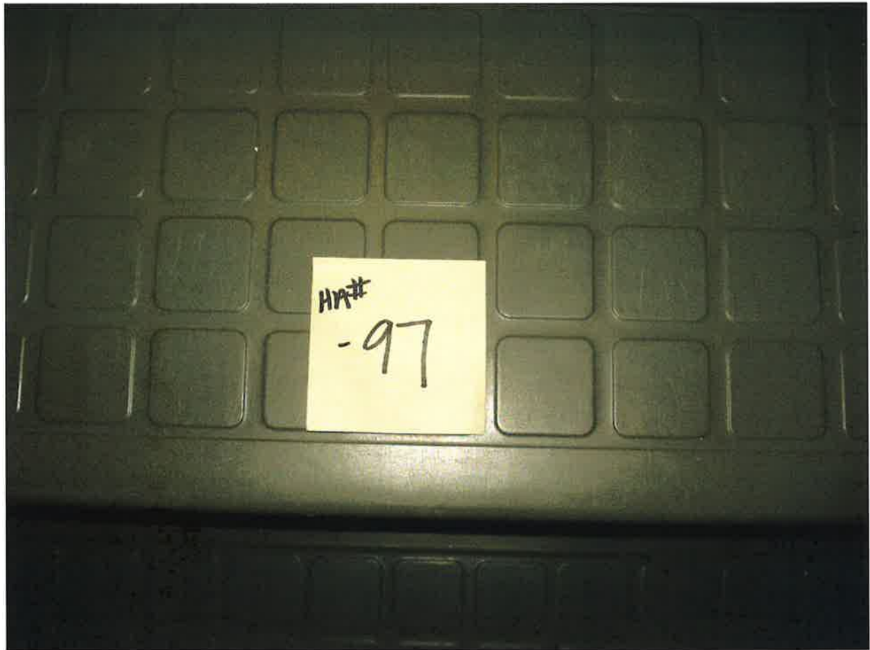
HA #97 – Non asbestos containing gray stair tread and associated mastic
