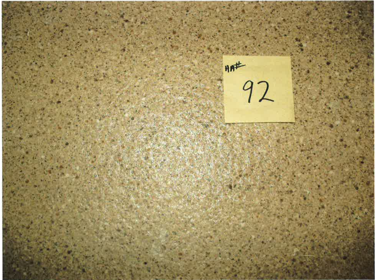
HA #92 – Assumed asbestos containing tan linoleum with brown and white specks and associated mastic
