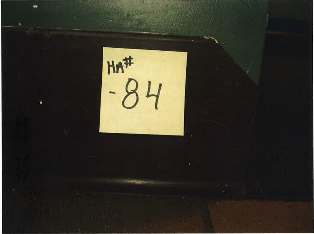
HA #84 – Non asbestos containing 6” brown baseboard and associated mastic
