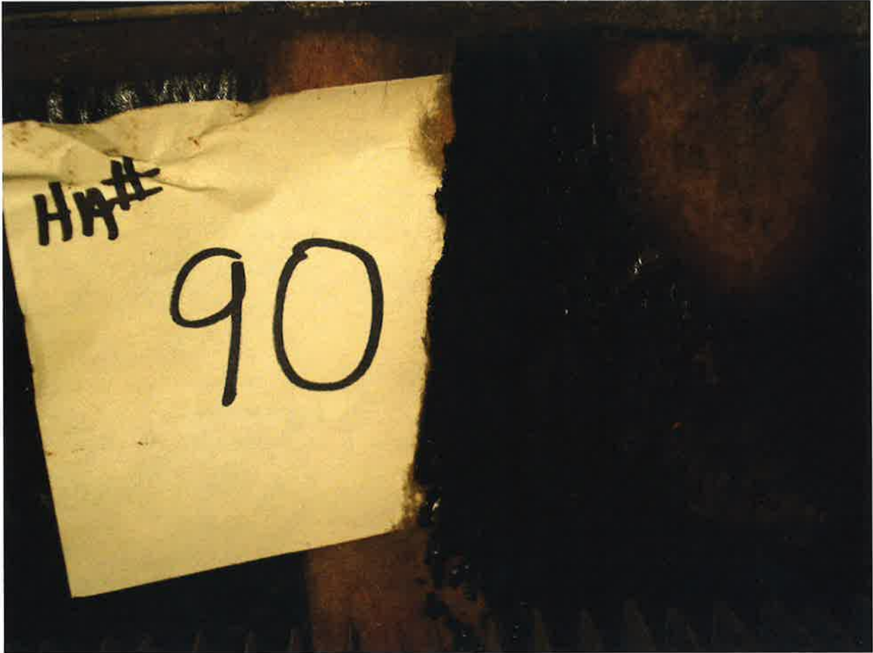
HA #90 – Non asbestos containing black tar paper on fiberglass insulation squares
