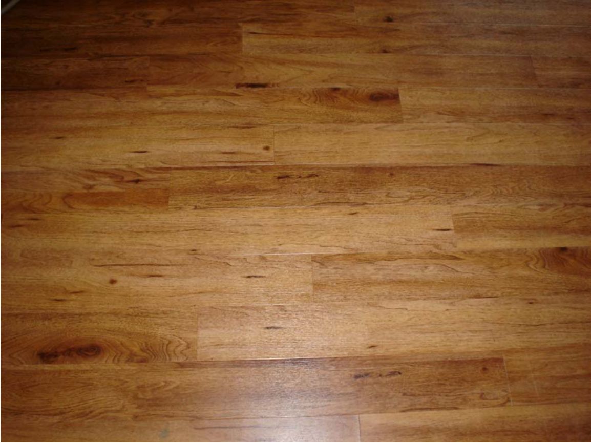
Photo 10 – Non asbestos-containing vinyl wood grain flooring and associated mastic
