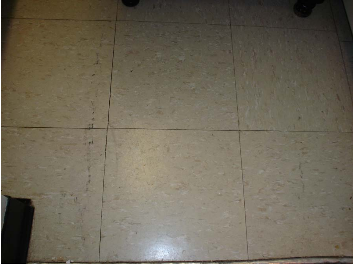
Photo 4 – Non asbestos-containing 12” x 12” cream floor tile with white and tan streaks and associated mastic
