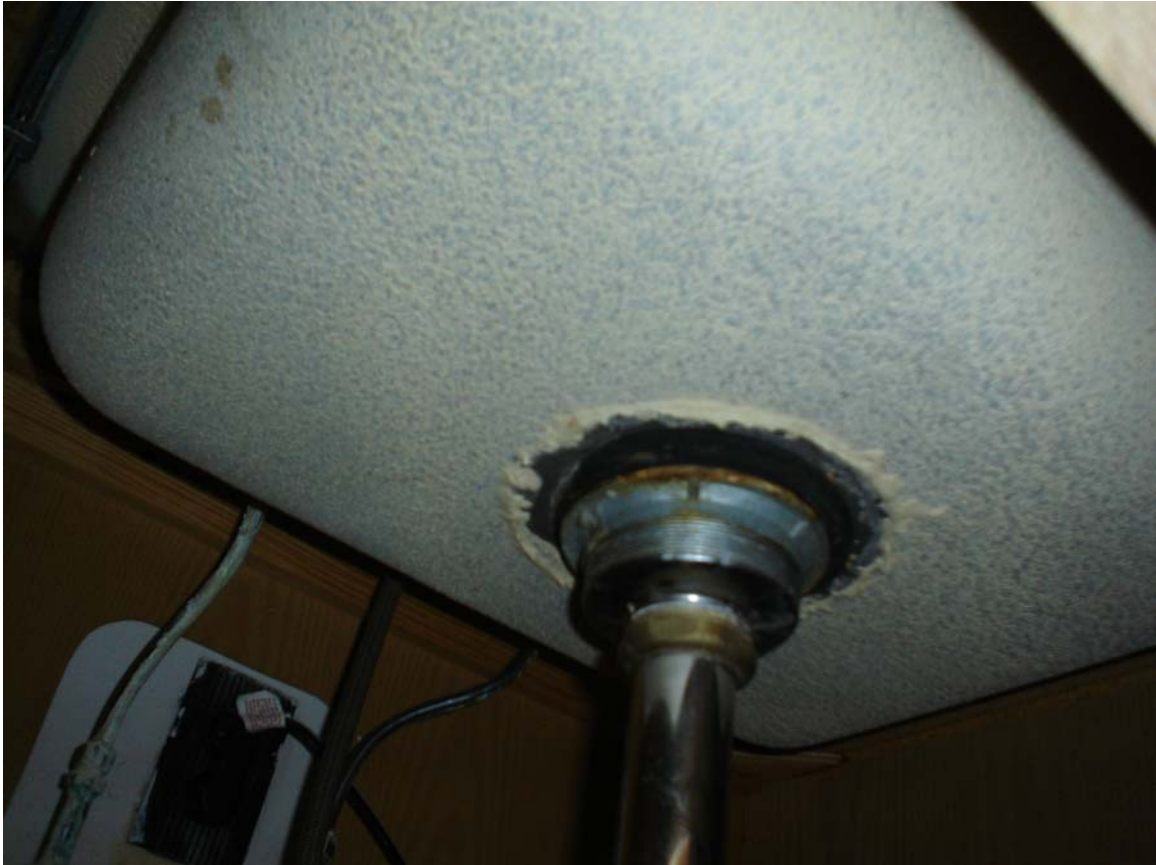
Photo 5 – Non asbestos-containing white sink undercoating
