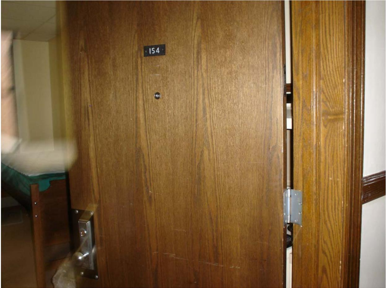
Assumed asbestos-containing fire door and frame
