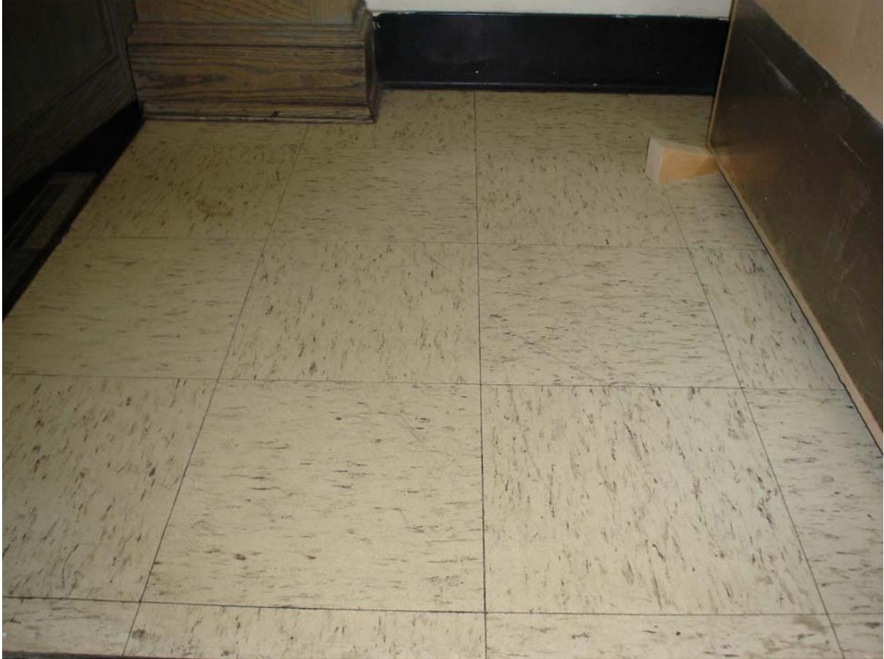
Non-asbestos containing 12" x 12" cream floor tile with tan and rust streaks
