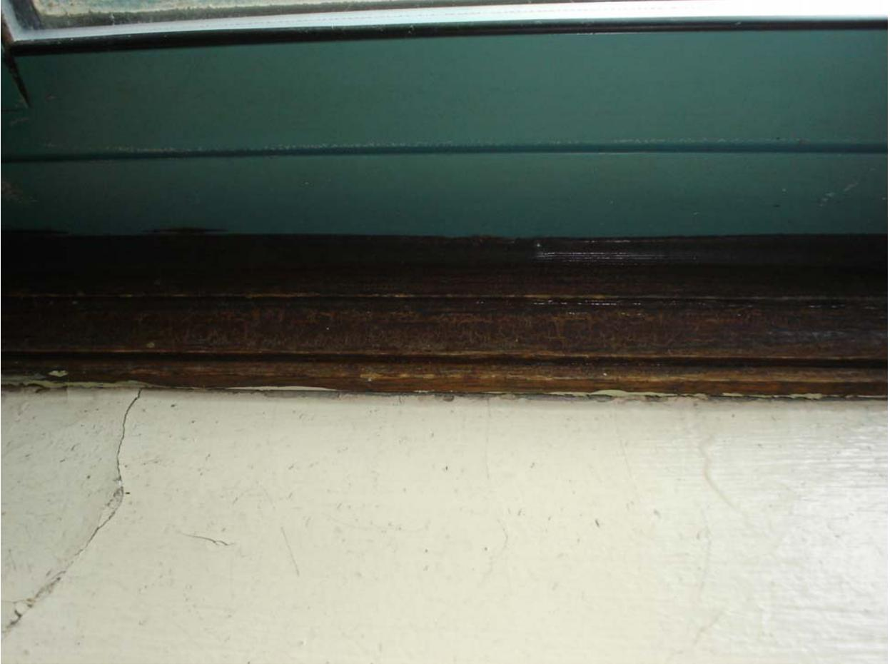
Assumed asbestos-containing window and door frame caulk compound
