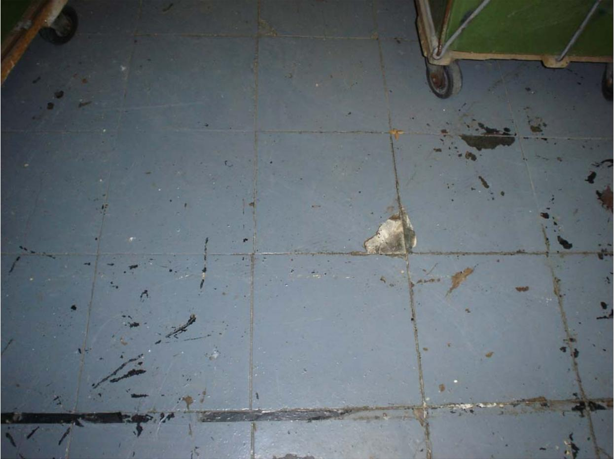
Asbestos-containing 12" x 12" brown floor tile and associated mastic
