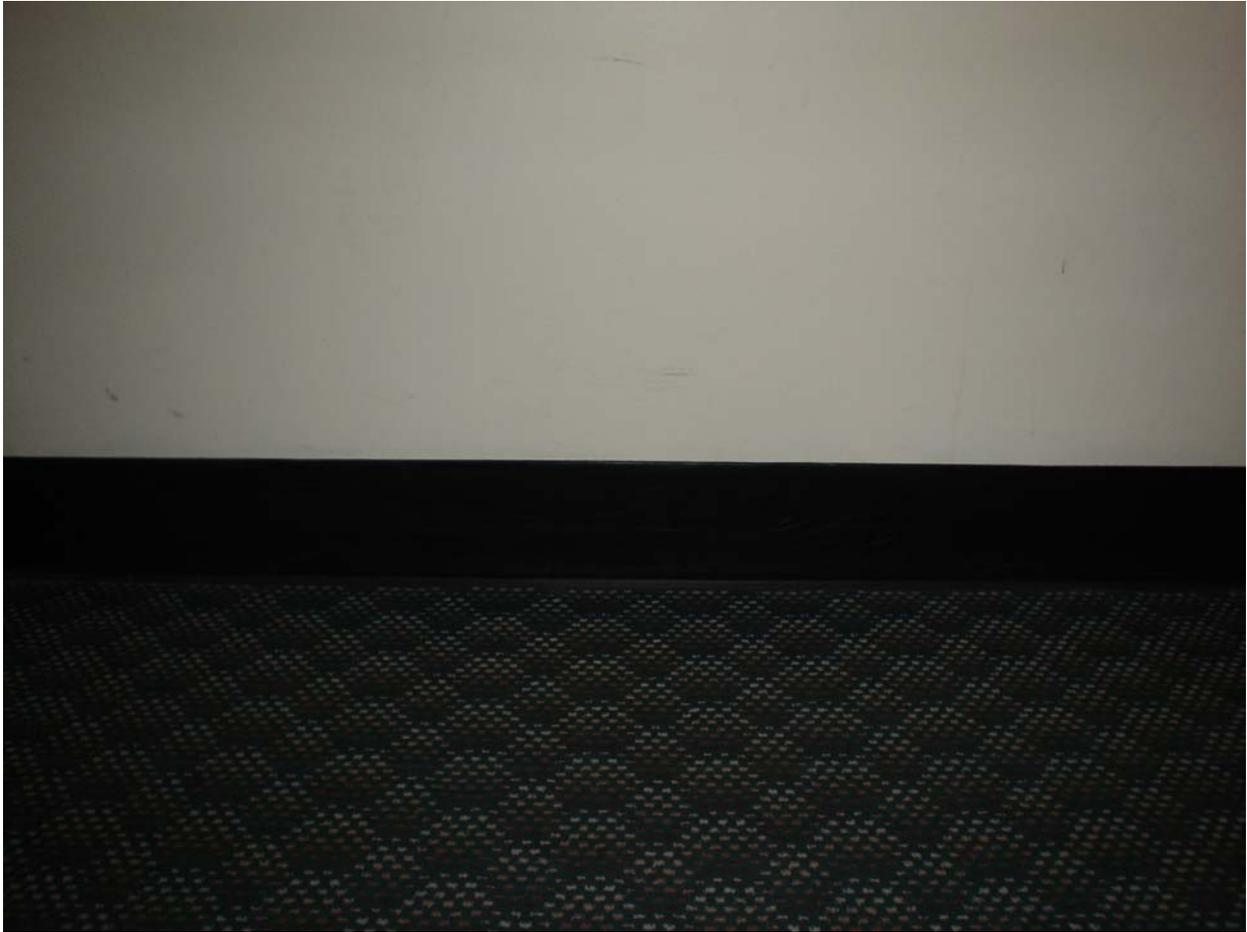
Non-asbestos containing 6" black cove molding and associated mastic
