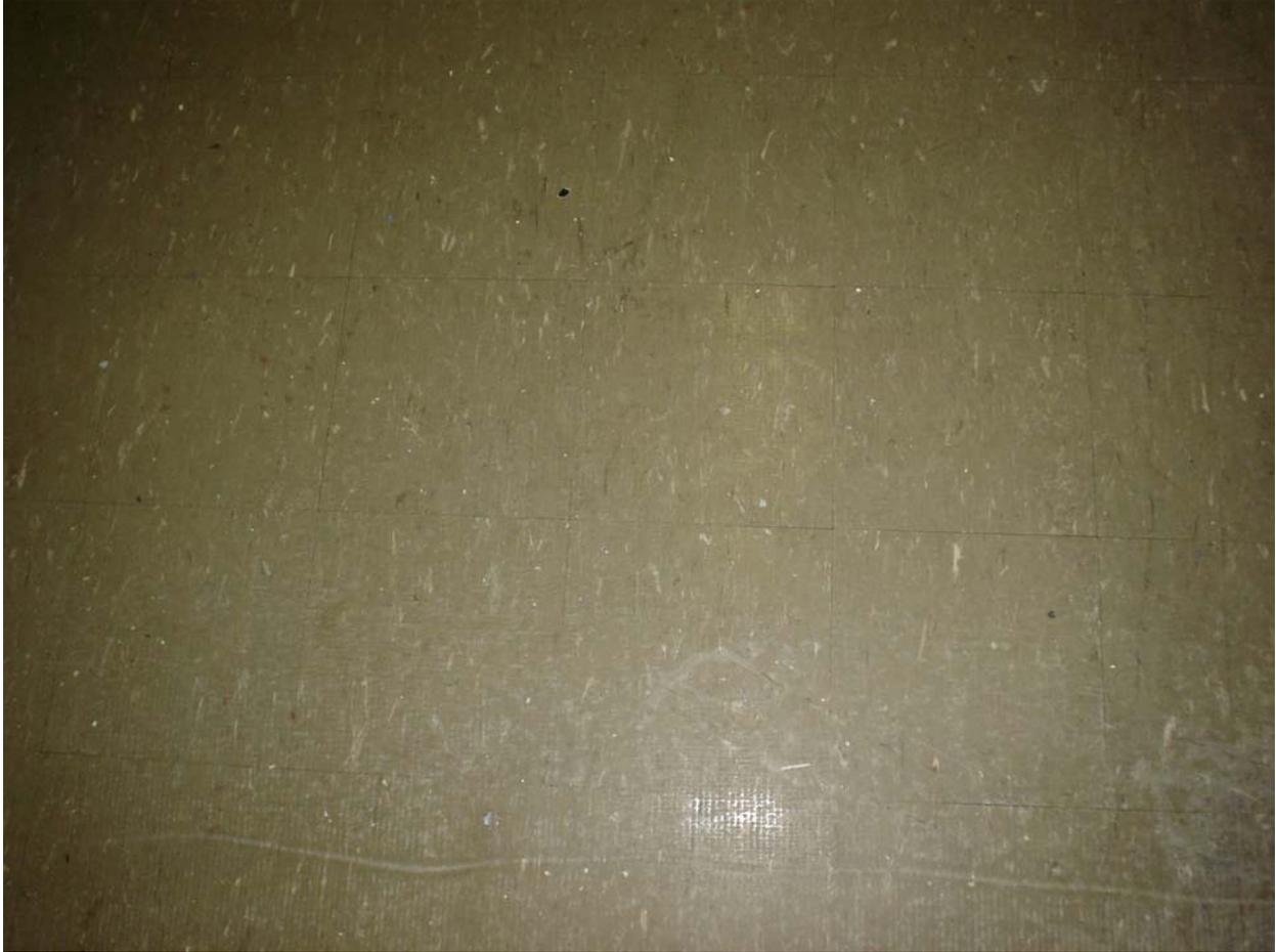
Asbestos-containing 9" x 9" army green floor tile with cream streaks
