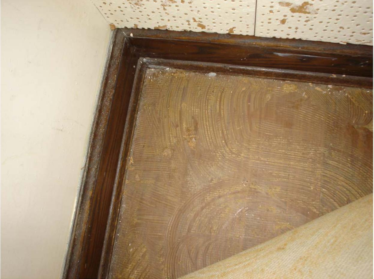
Non-asbestos containing brown floor covering and associated mastic
