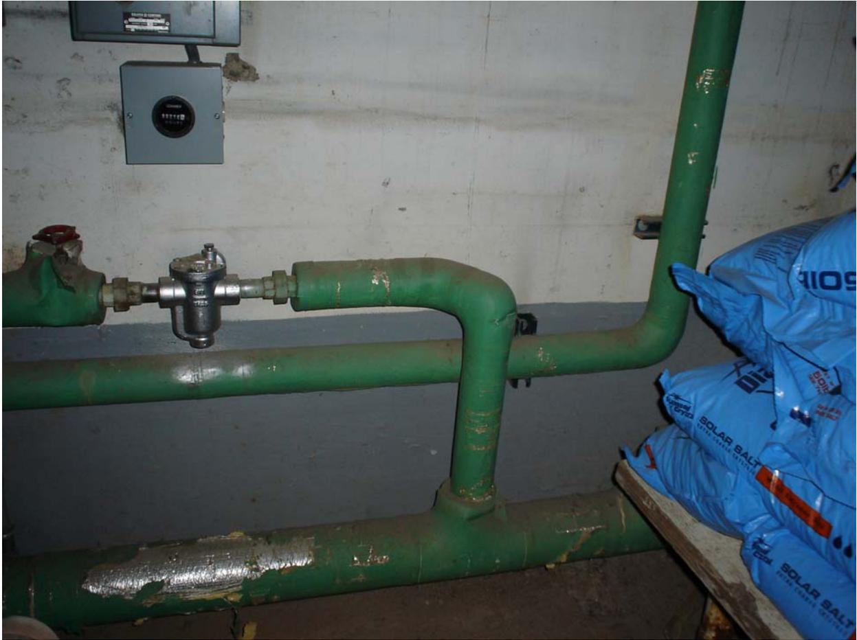
Asbestos-containing steam/condensate supply & return pipe straight insulation
