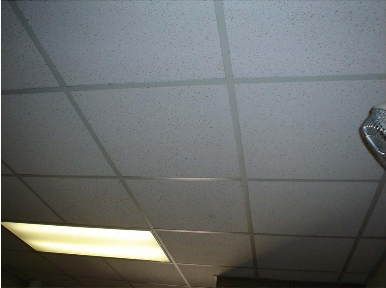
Non-asbestos containing 2' x 2' white lay-in ceiling tile with fissures
