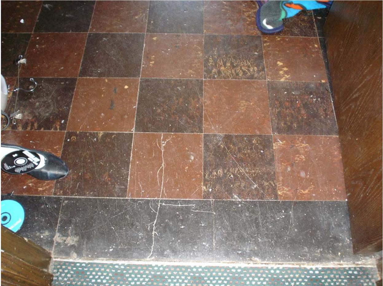
Asbestos-containing 9" x 9" brown floor tile with cream and rust streaks
