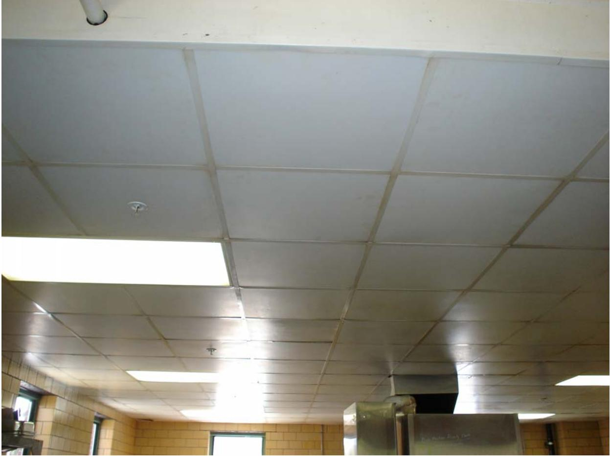
Non-asbestos containing white lay-in ceiling tile with pin holes
