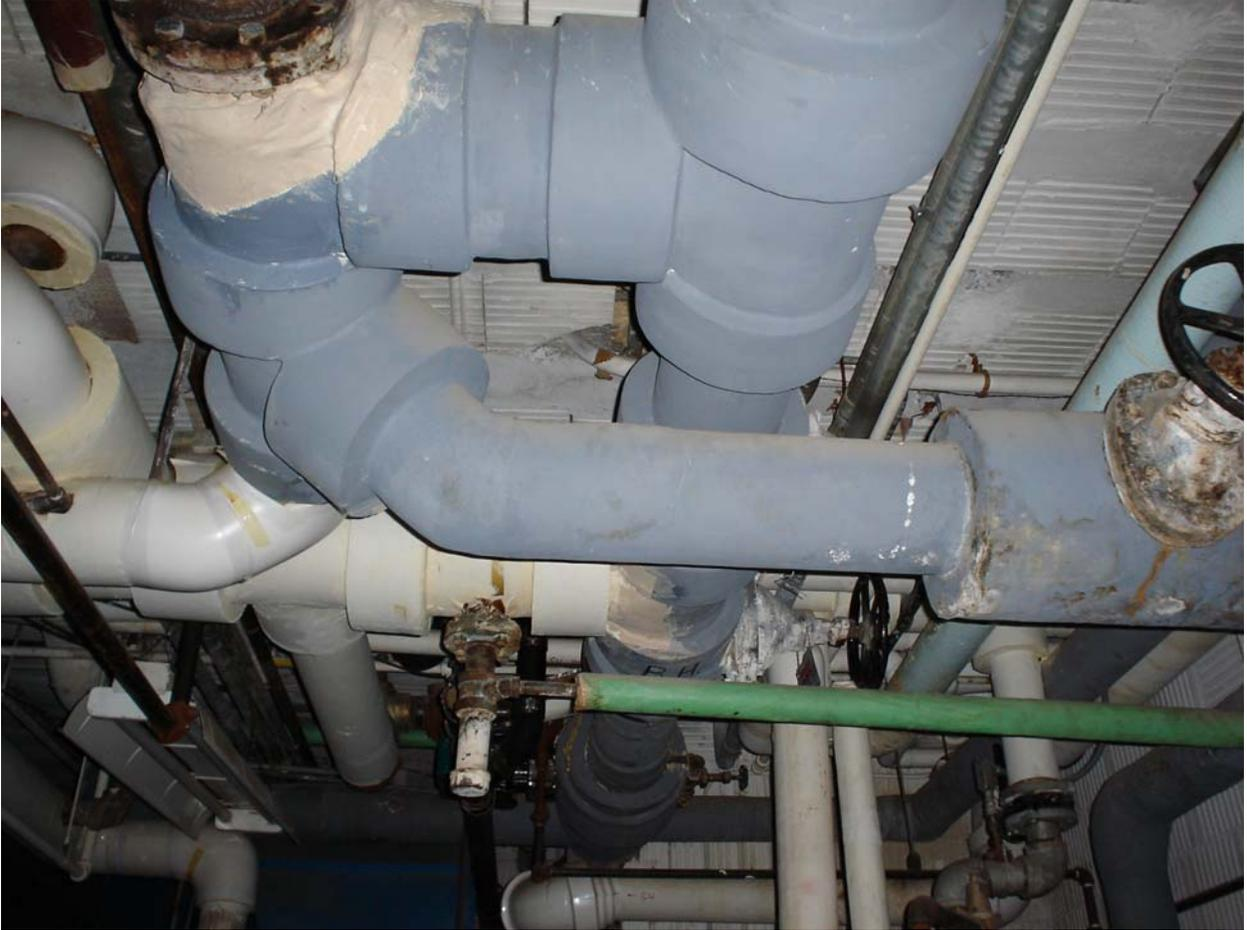
Asbestos-containing steam/condensate supply & return pipe joint insulation
