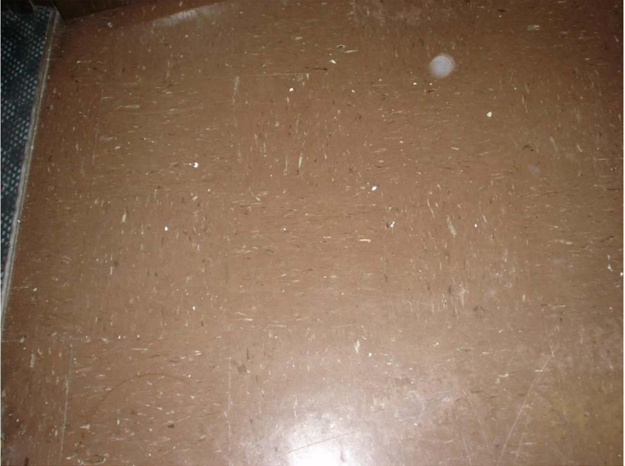
Asbestos-containing 12" x 12" chocolate brown floor tile with cream streaks and associated mastic
