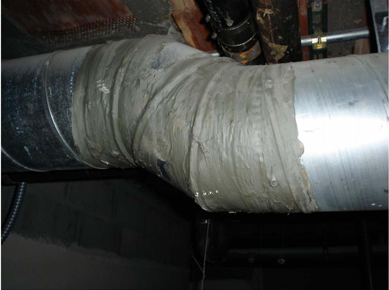
Non-asbestos containing gray duct caulk compound
