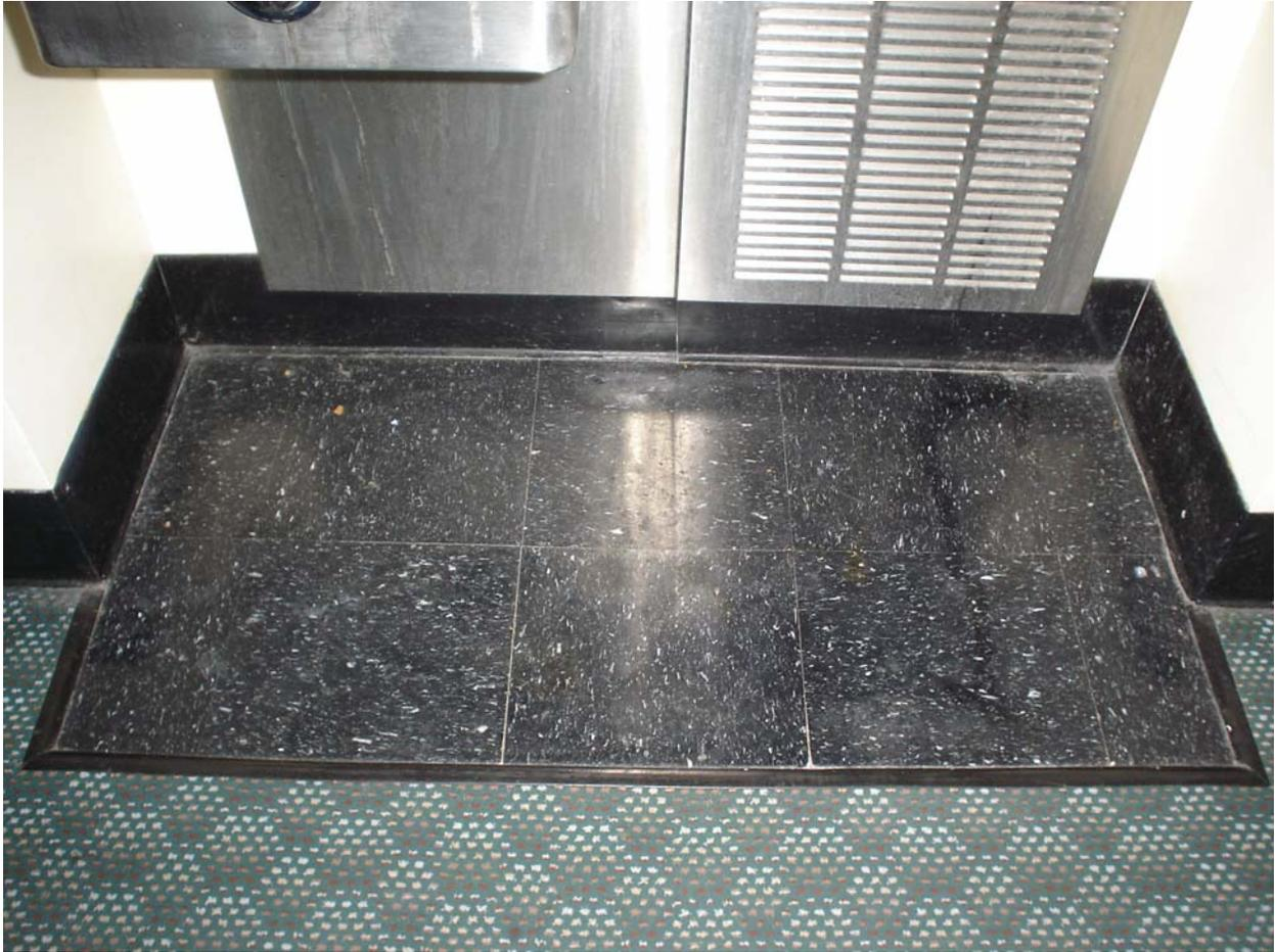
Non-asbestos containing 12" x 12" black floor tile with white specks and associated mastic
