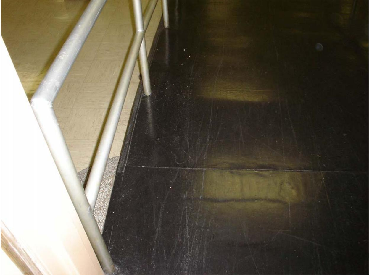
Non-asbestos containing 12" x 12" gray floor tile with cream streaks (painted black) and associated mastic
