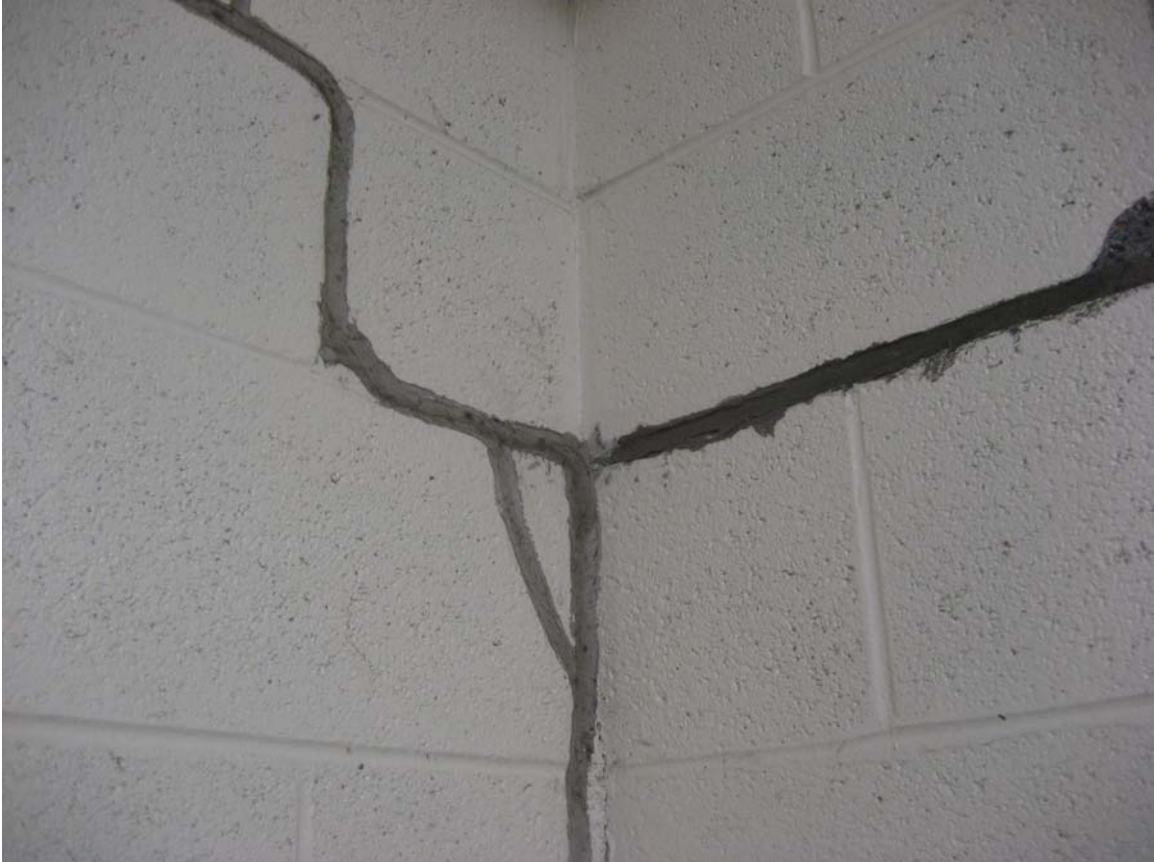
HA #5 – Non asbestos containing Grey Building Caulk
