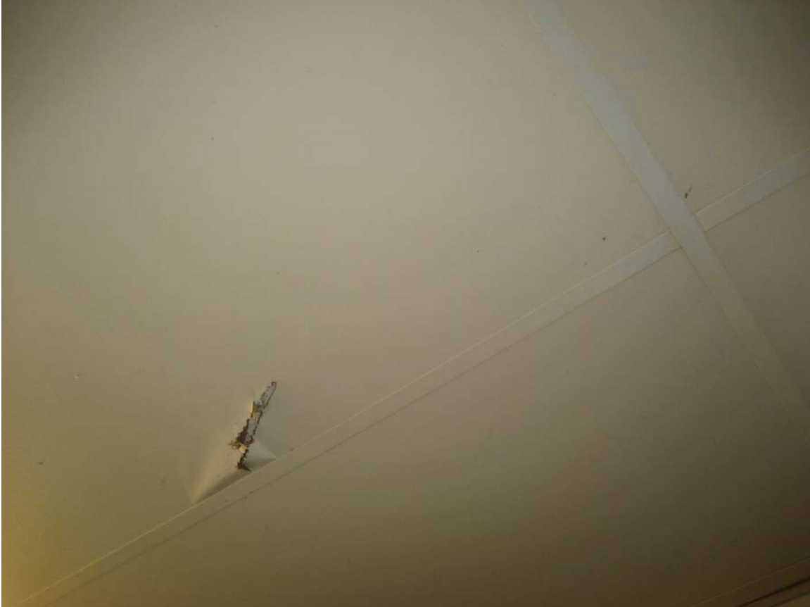
HA #8 – Non asbestos containing 2' x 4' white smooth lay in ceiling tile
