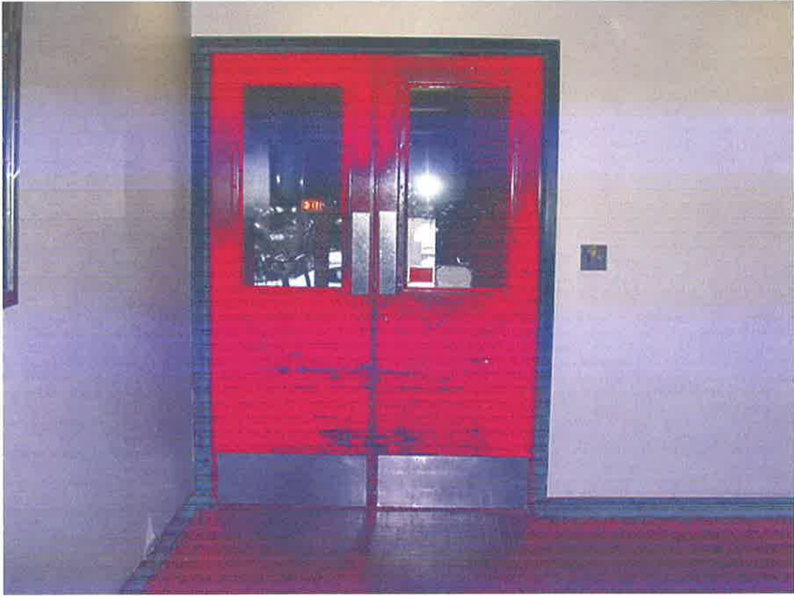
Photo 18 – Fire door, southwest landing to 1 st floor entrance
