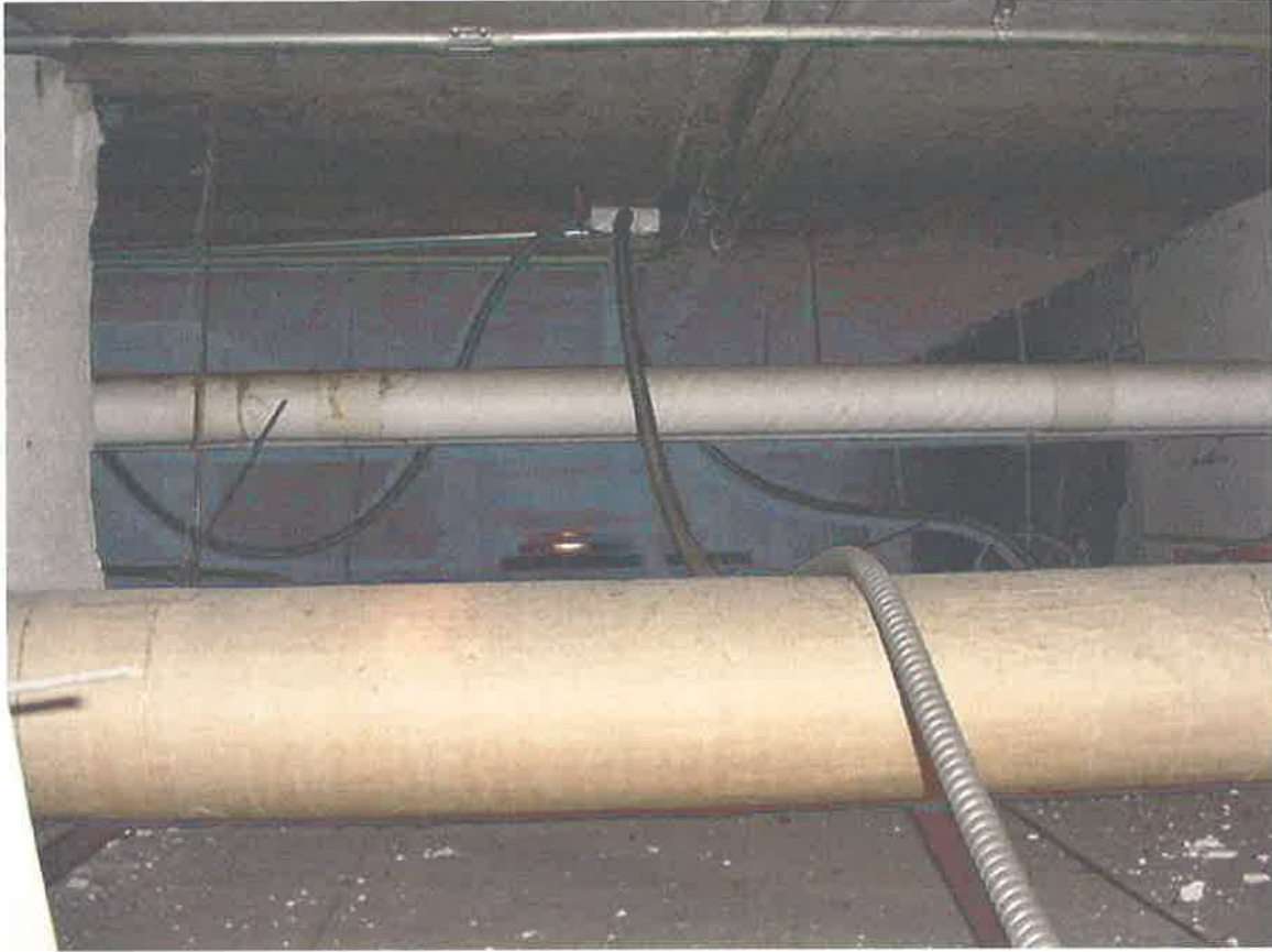
Photo 30 – 5 th floor, ceiling plenum access area, facing east from southwest corner
