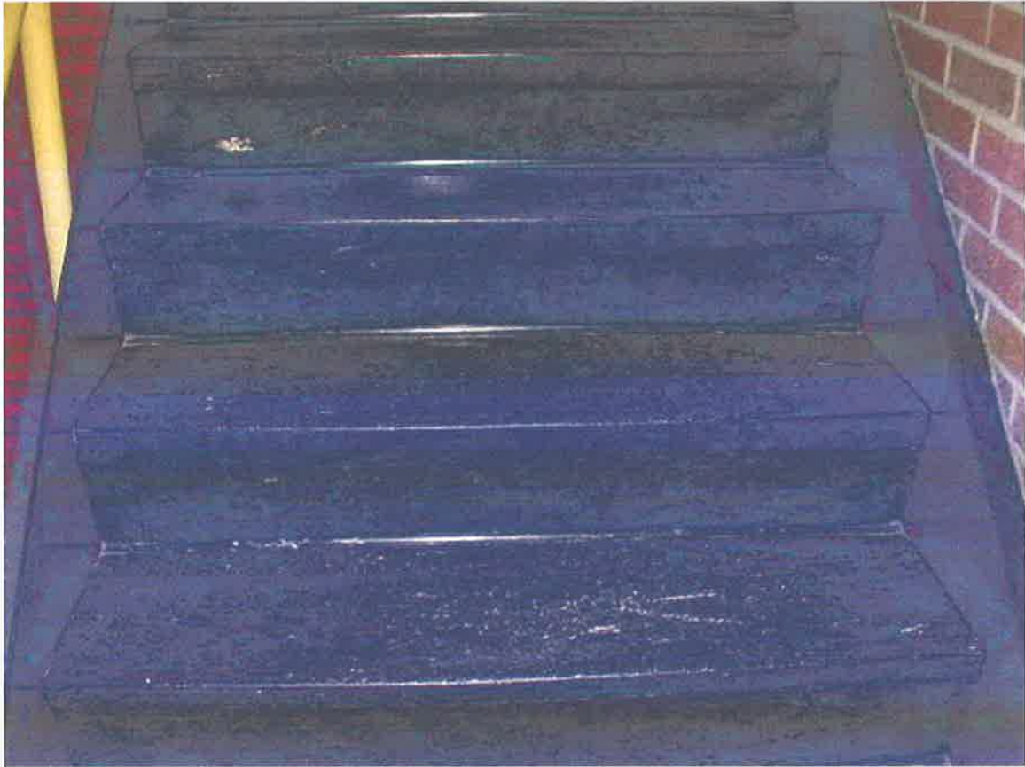
Photo 24 – Black vinyl stair tread with white streaks, southwest stairwell
