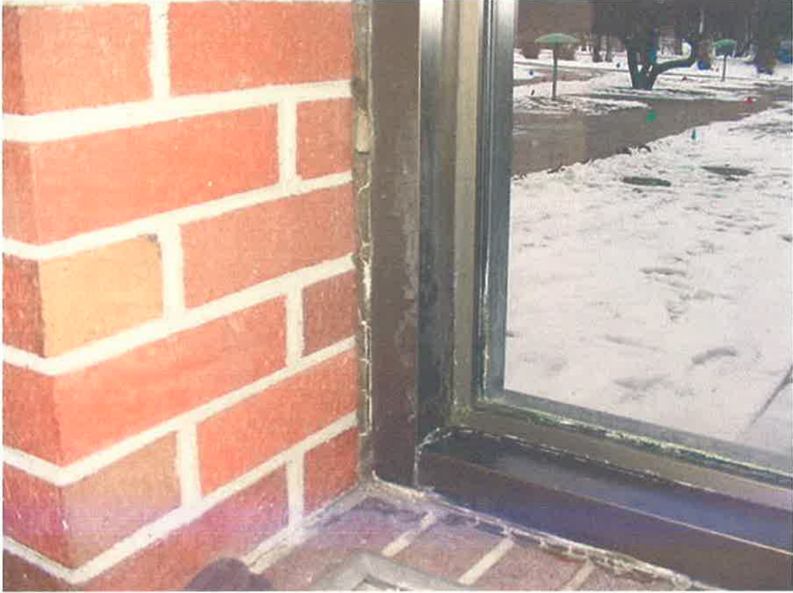
Photo 25 – Window caulk (inside), northeast landing of 1 st floor, facing south
