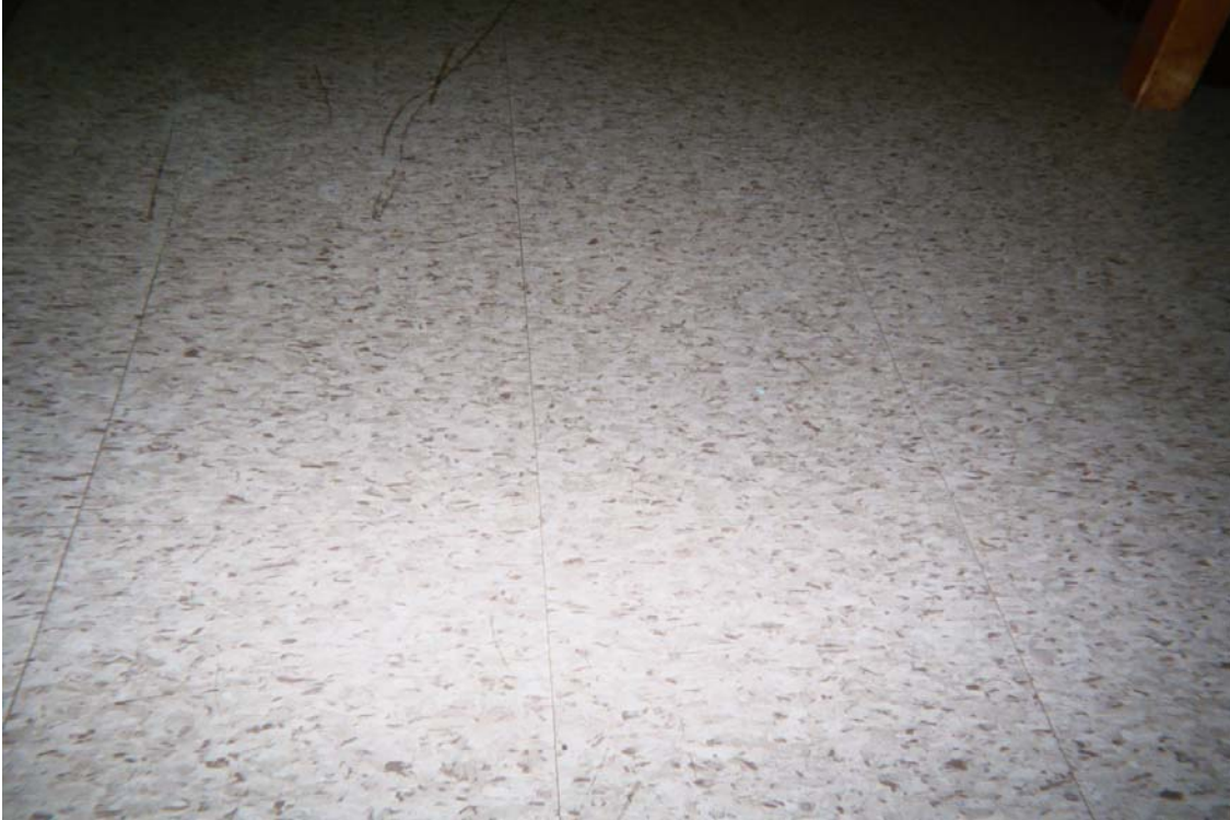
Non asbestos-containing 12" x 12" tan and brown marble floor tile and associated mastic
