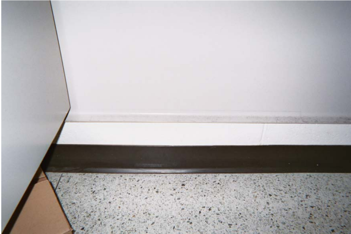
Non asbestos-containing 4" brown cove molding and associated mastic
