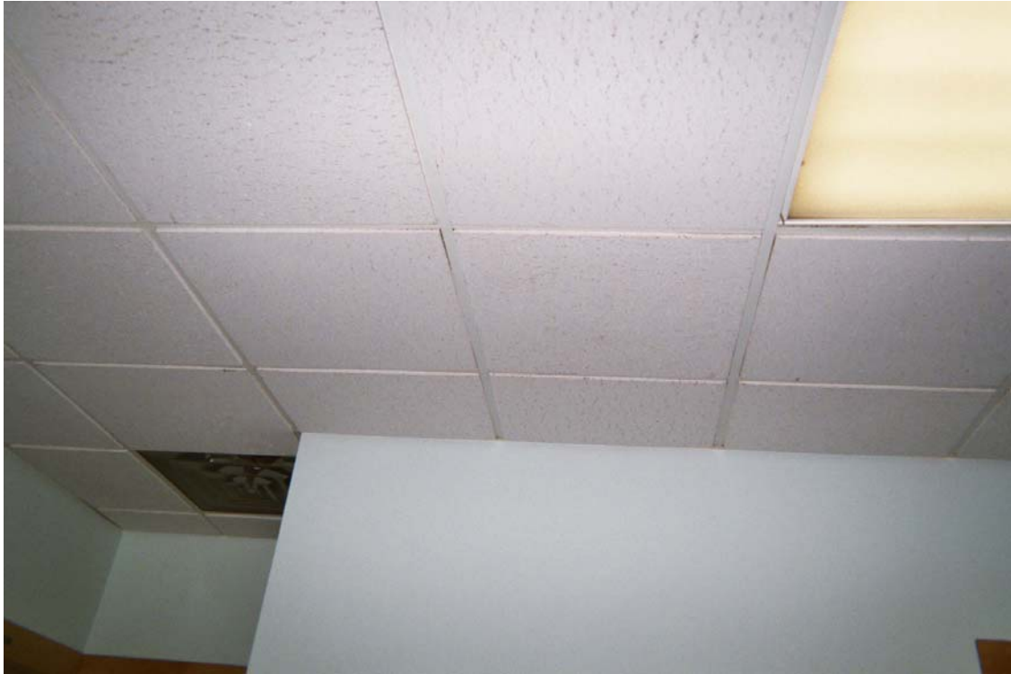
Non asbestos-containing 2' x 2' white drop-in ceiling tile with rough texture
