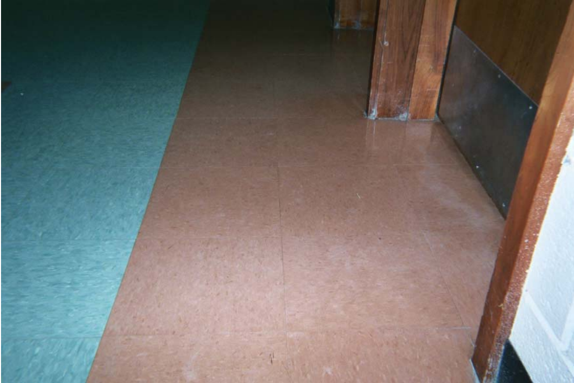
Non asbestos-containing 12" x 12" orange marble pattern floor tile and associated mastic
