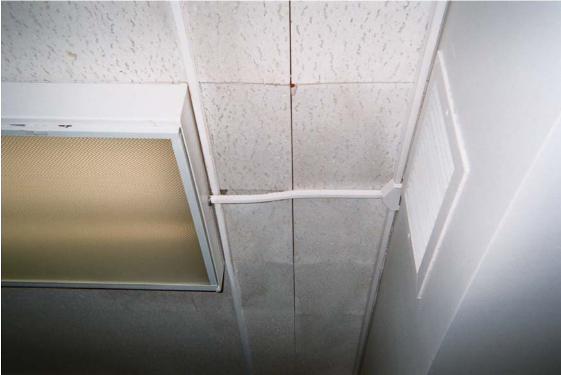
Non asbestos-containing 12" x 12" white ceiling tile with pin holes and fissures and associated glue pods
