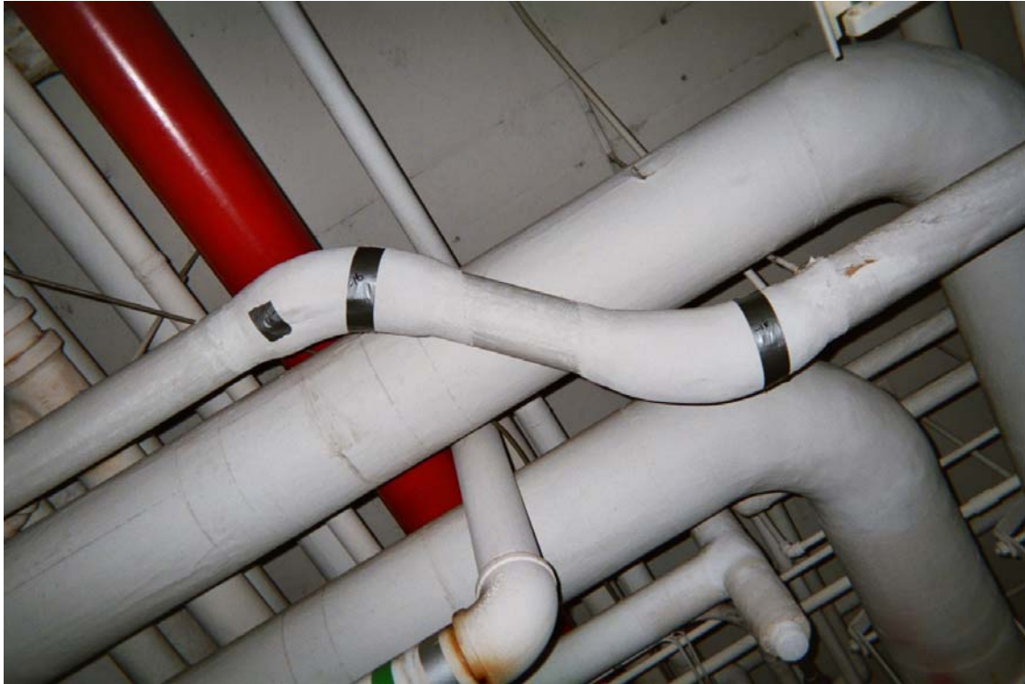
Asbestos-containing wastewater pipe joint/hanger insulation
