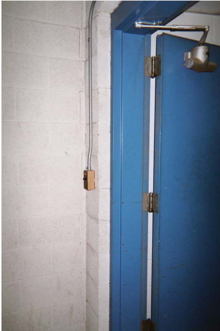
Assumed asbestos-containing fire door and frame
