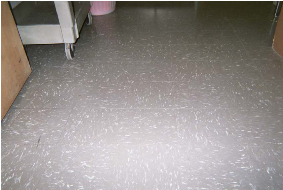
Asbestos-containing 9" x 9" gray floor tile with white streaks and associated mastic
