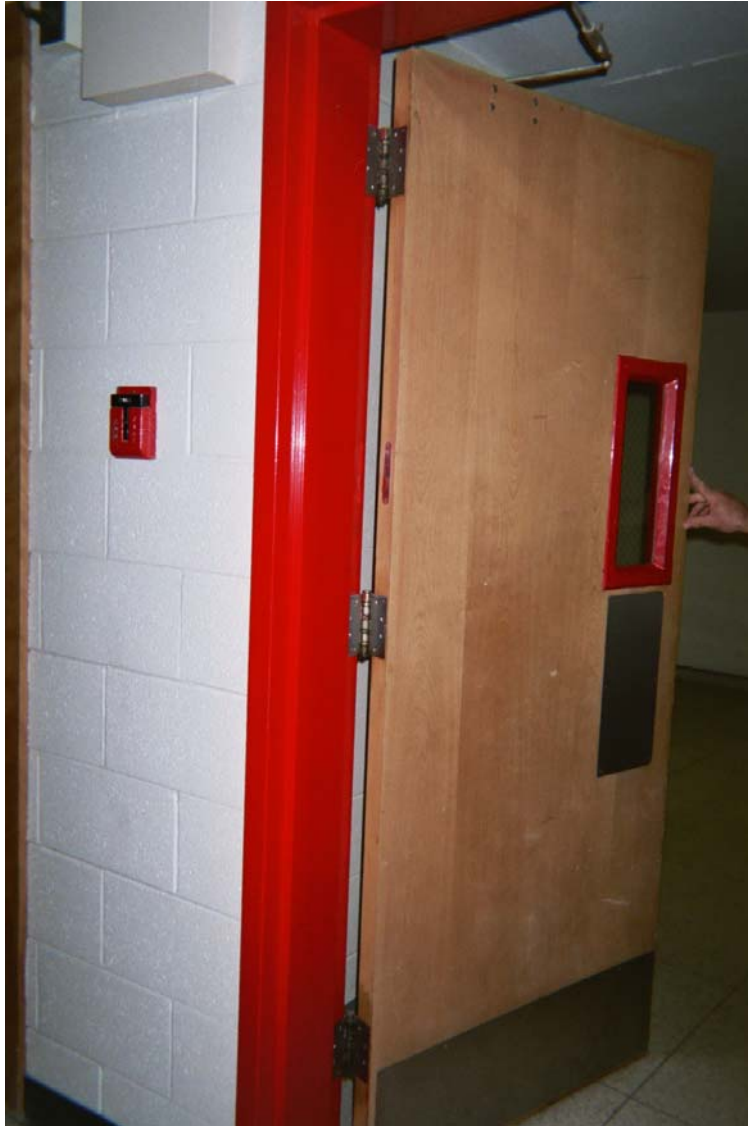
Assumed asbestos-containing fire door and frame
