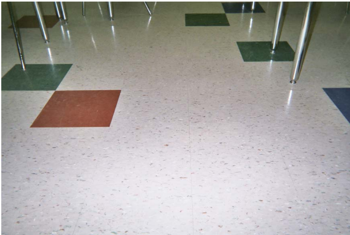
Non asbestos-containing 12" x 12' tan floor tile with multi-colored specks and associated mastic
