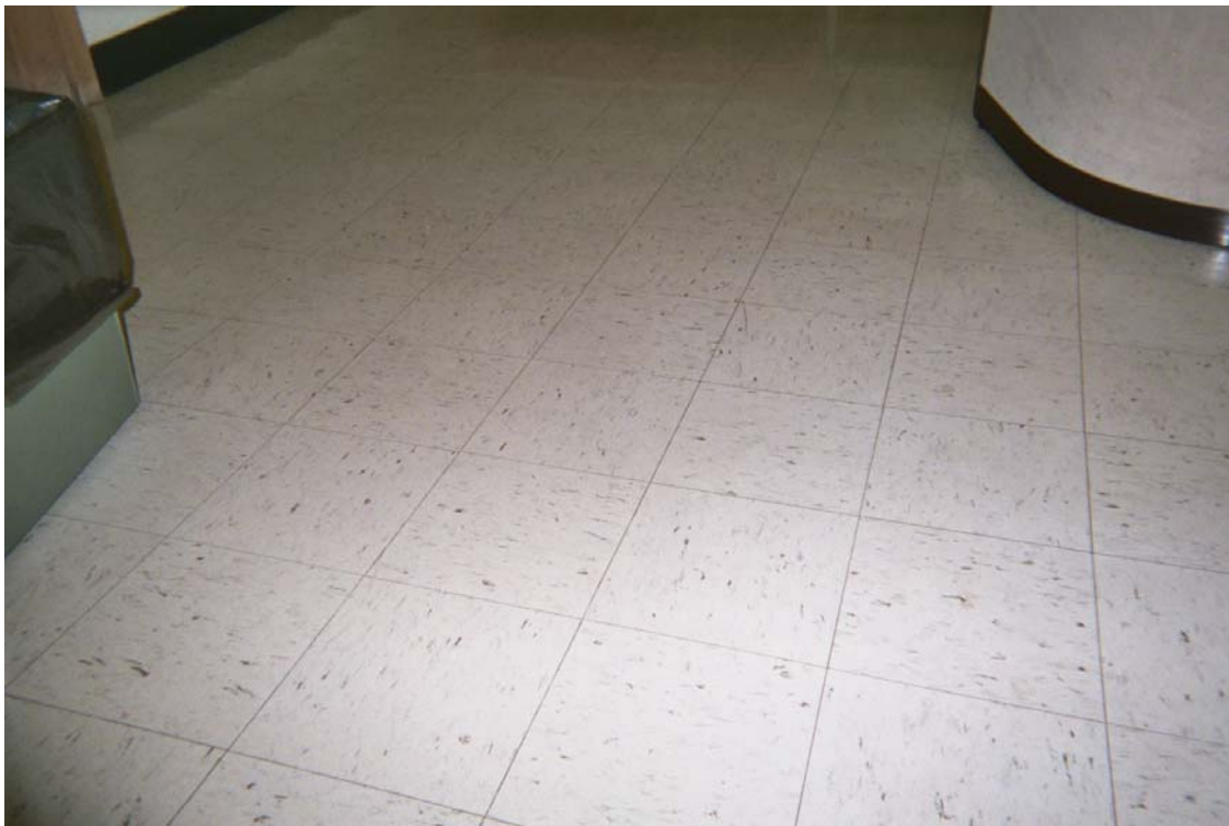
Asbestos-containing 9" x 9" white floor tile with gray streaks and associated mastic
