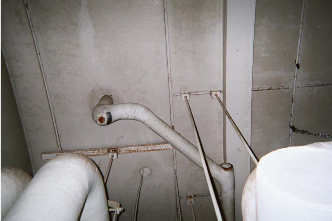
Asbestos-containing drain line pipe joint/hanger insulation on fiberglass
