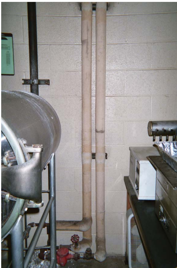
Asbestos-containing steam/condensate pipe straight insulation
