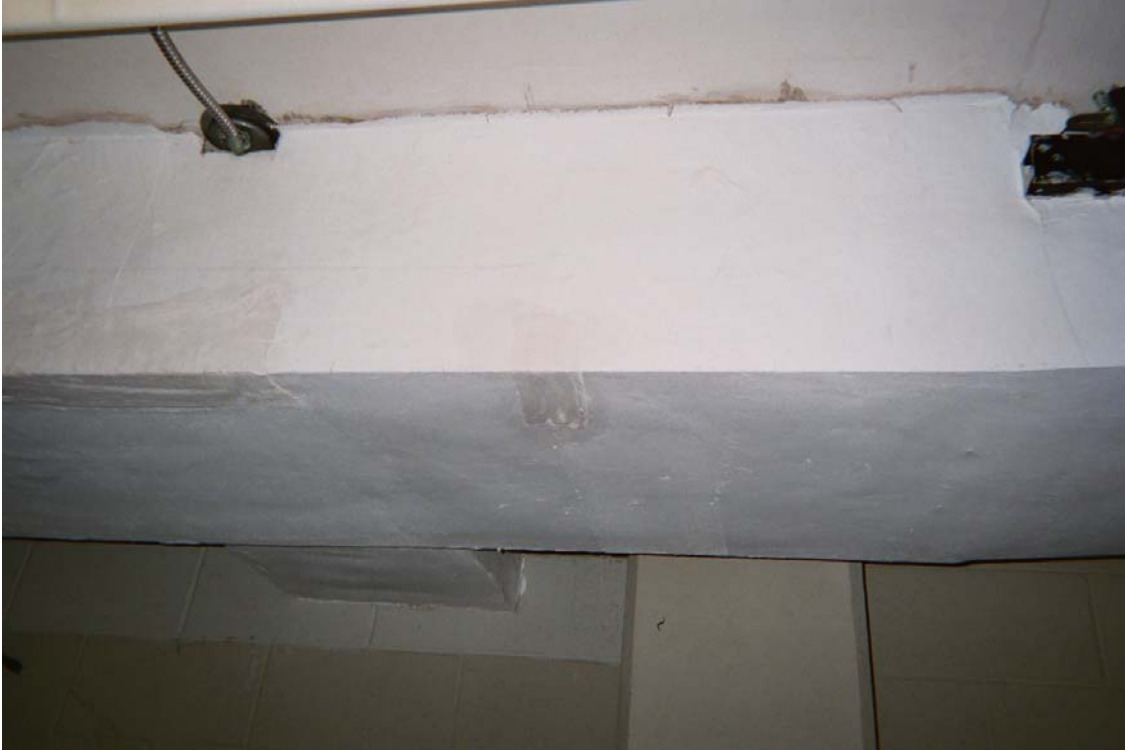
Asbestos-containing duct wrap insulation
