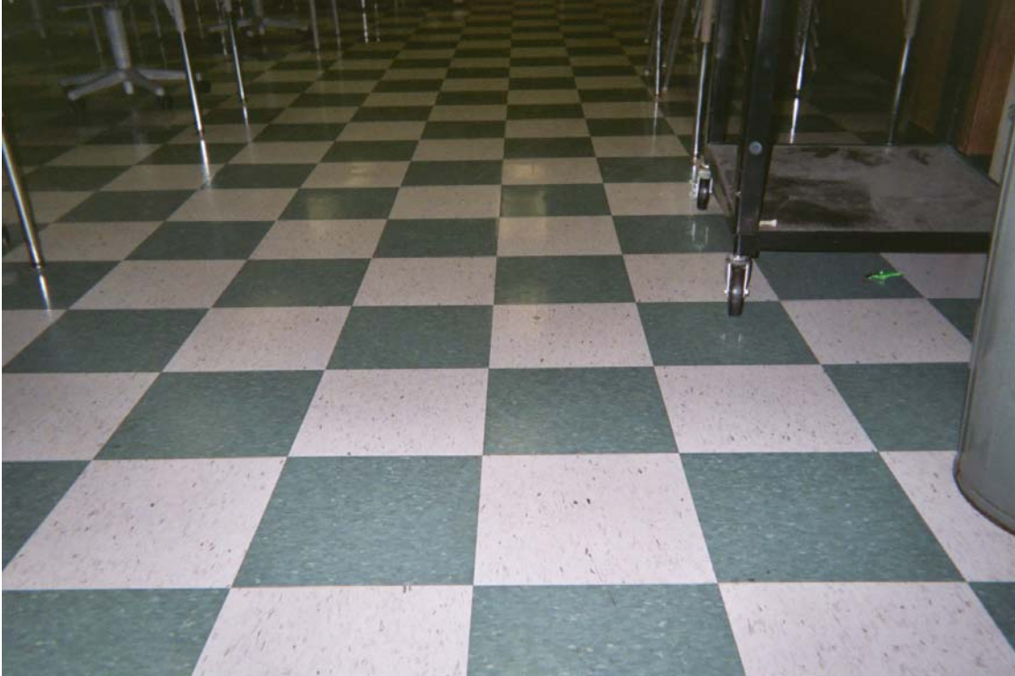
Non asbestos-containing 12" x 12" dark green marble pattern floor tile and associated mastic
