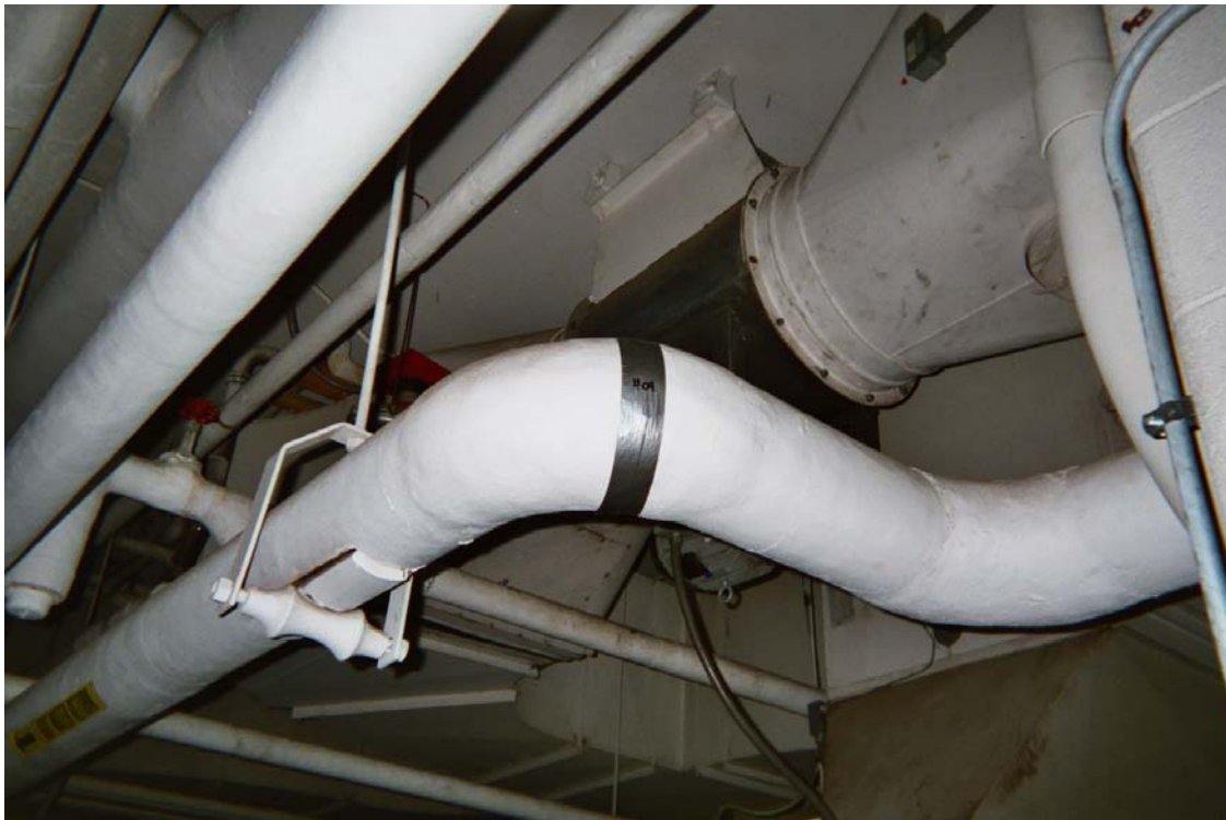
Asbestos-containing domestic water pipe joint and hanger insulation on fiberglass straight
