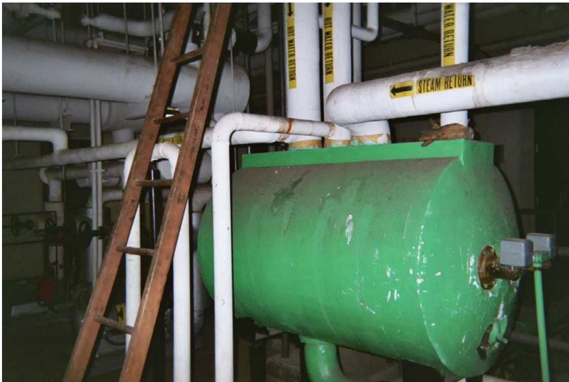
Asbestos-containing hot water holding tank insulation
