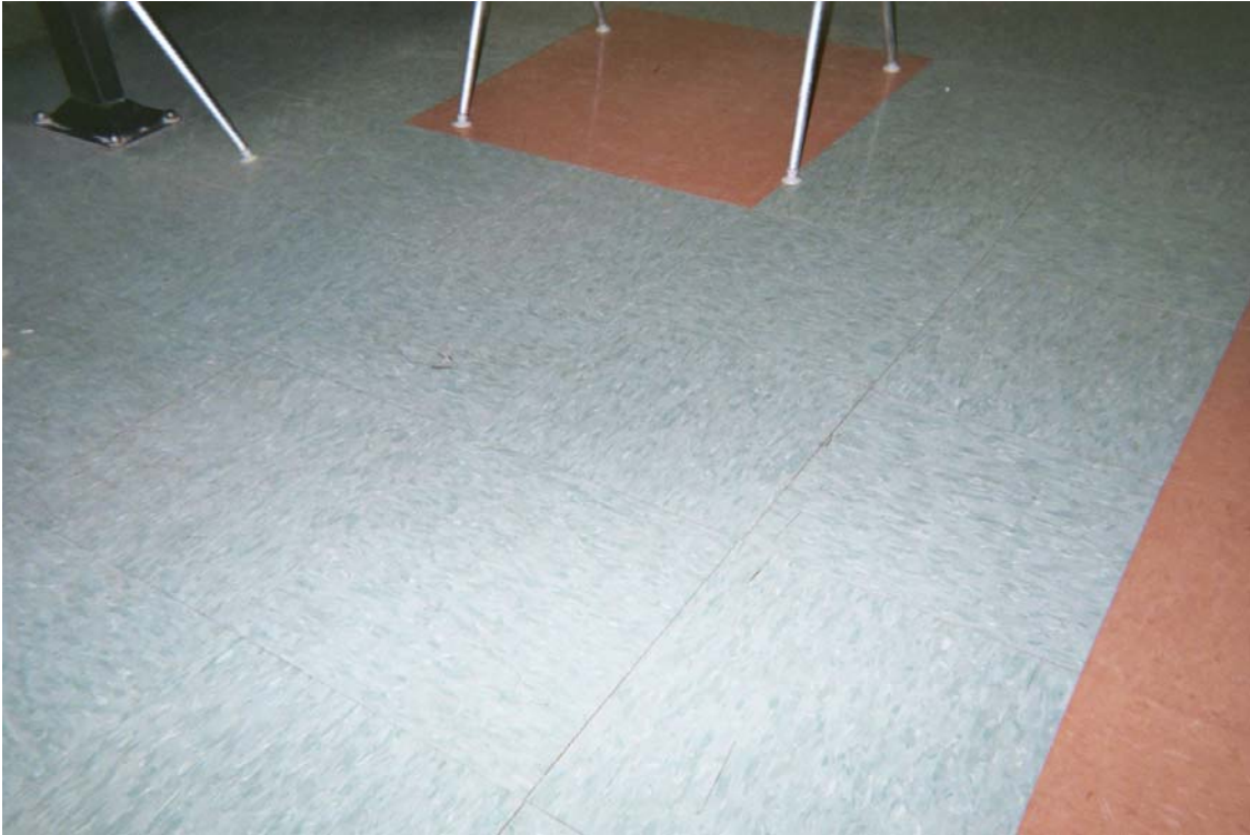
Non asbestos-containing 12" x 12" light green marble pattern floor tile and associated mastic
