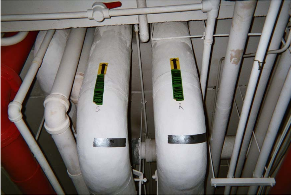
Asbestos-containing chilled water pipe joint/hanger insulation on fiberglass straight
