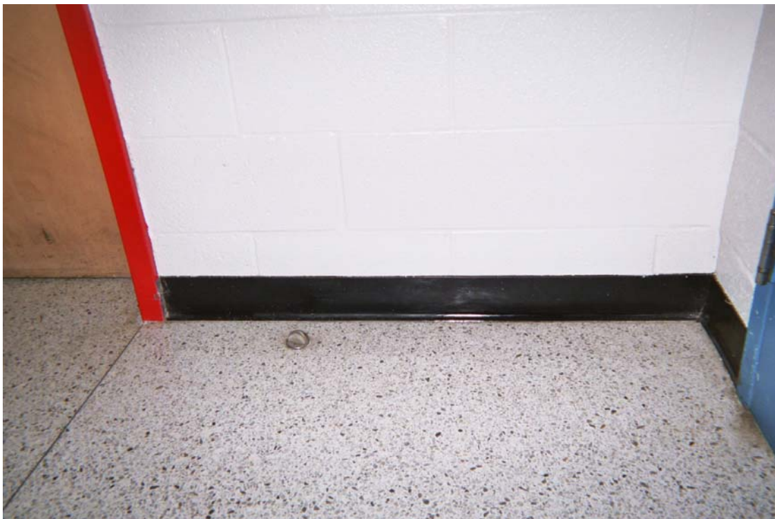
Non asbestos-containing 4" black cove molding and associated mastic
