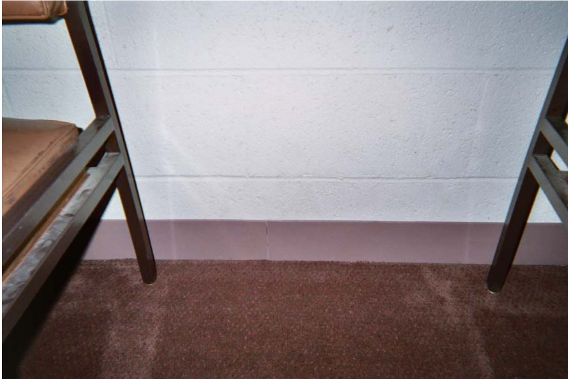
Non asbestos-containing 4" mauve cove molding and associated mastic
