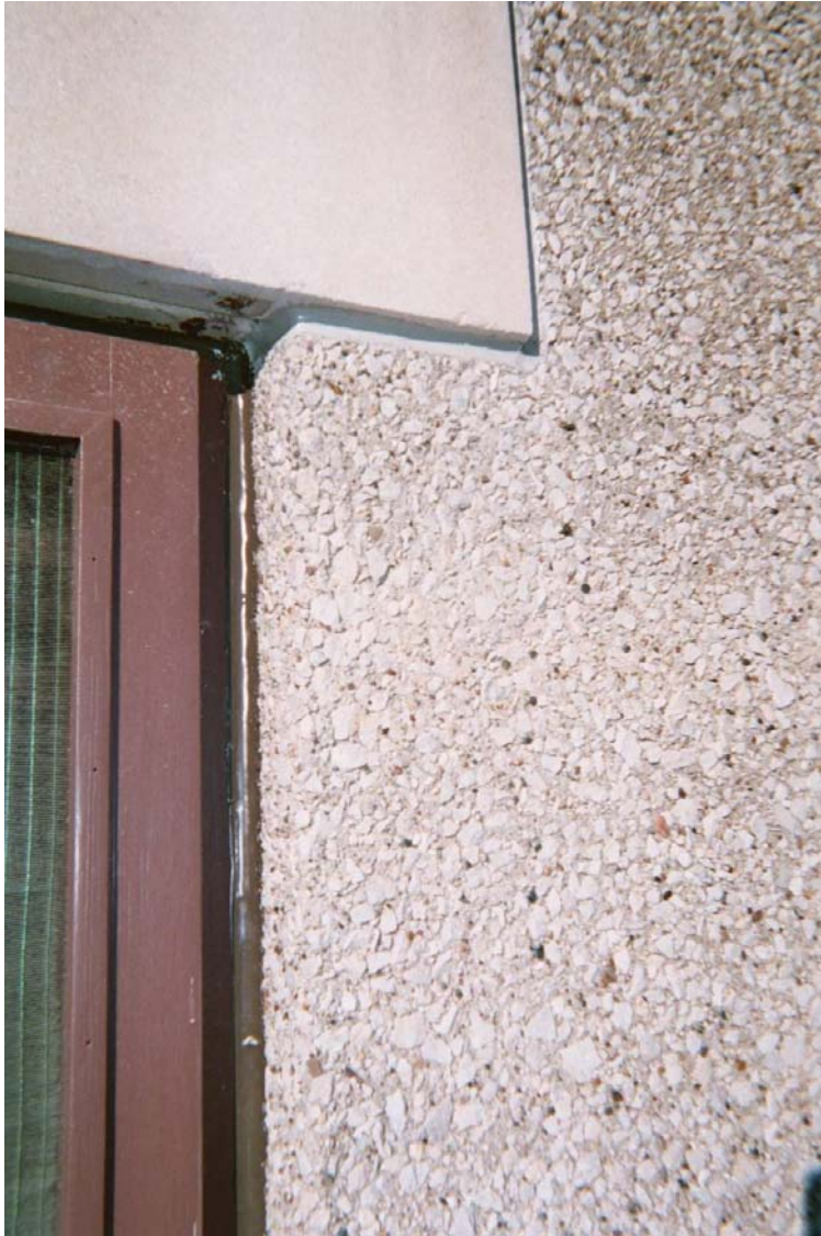
Assumed asbestos-containing gray exterior window and door frame caulk
