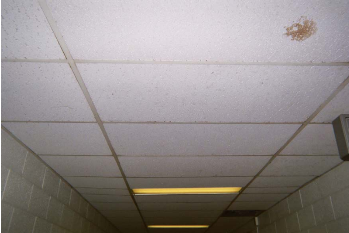
Non asbestos-containing 2' x 4' white lay-in ceiling tile with pin holes and fissures
