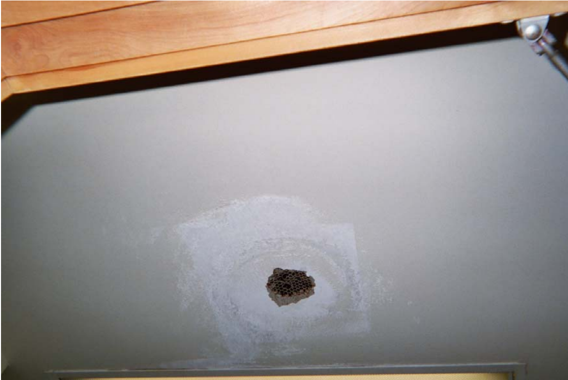
Non asbestos-containing plaster
