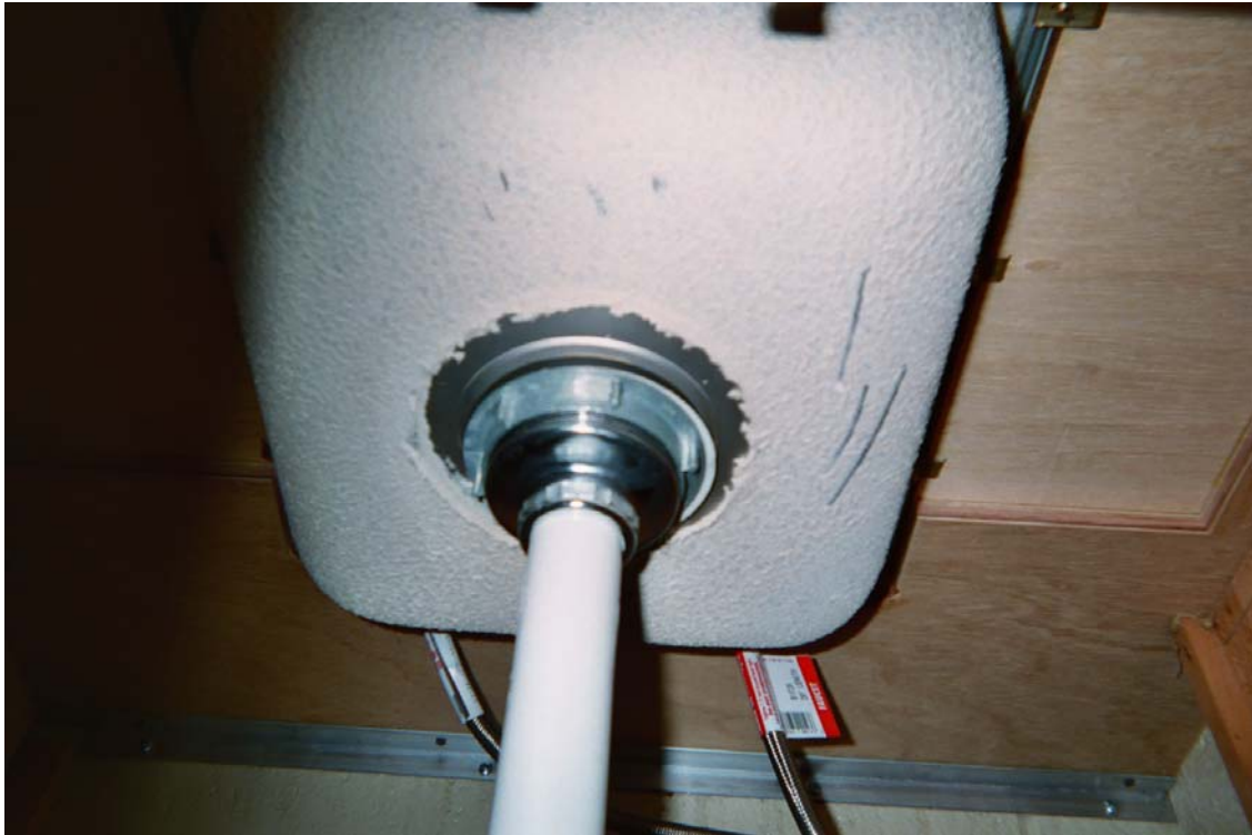
Non asbestos-containing white sink undercoating
