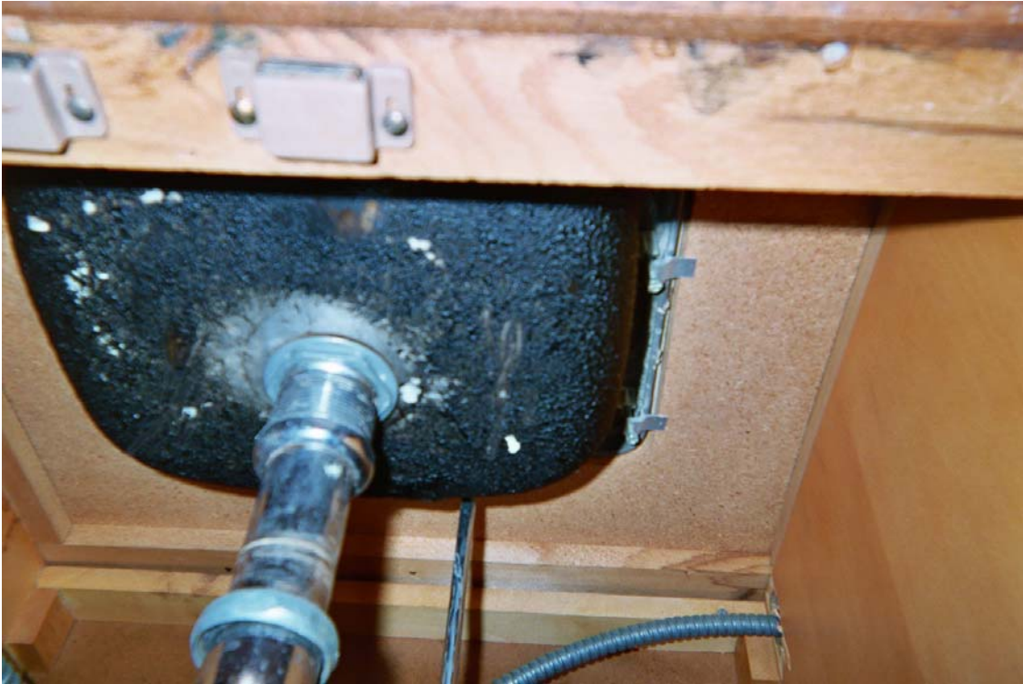
Asbestos-containing black sink undercoating
