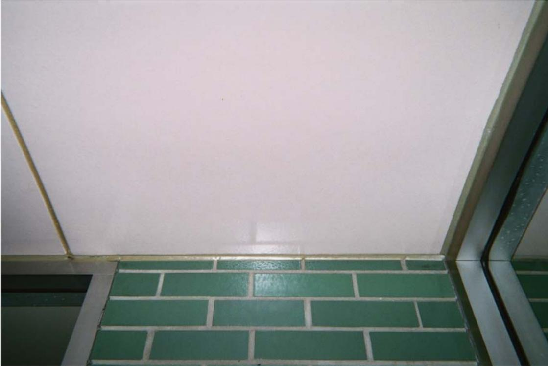
Photo 7 – Assumed asbestos-containing green building caulk compound
