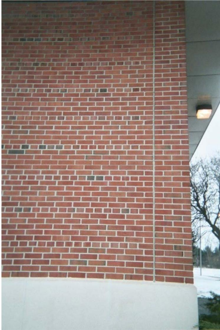
Photo 1 – Assumed asbestos-containing gray building caulk compound
