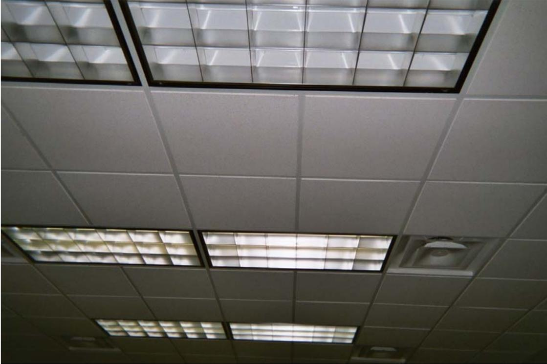
Photo 14 – Non asbestos-containing 2' x 2' white drop-in ceiling tile with pin holes and fissures
