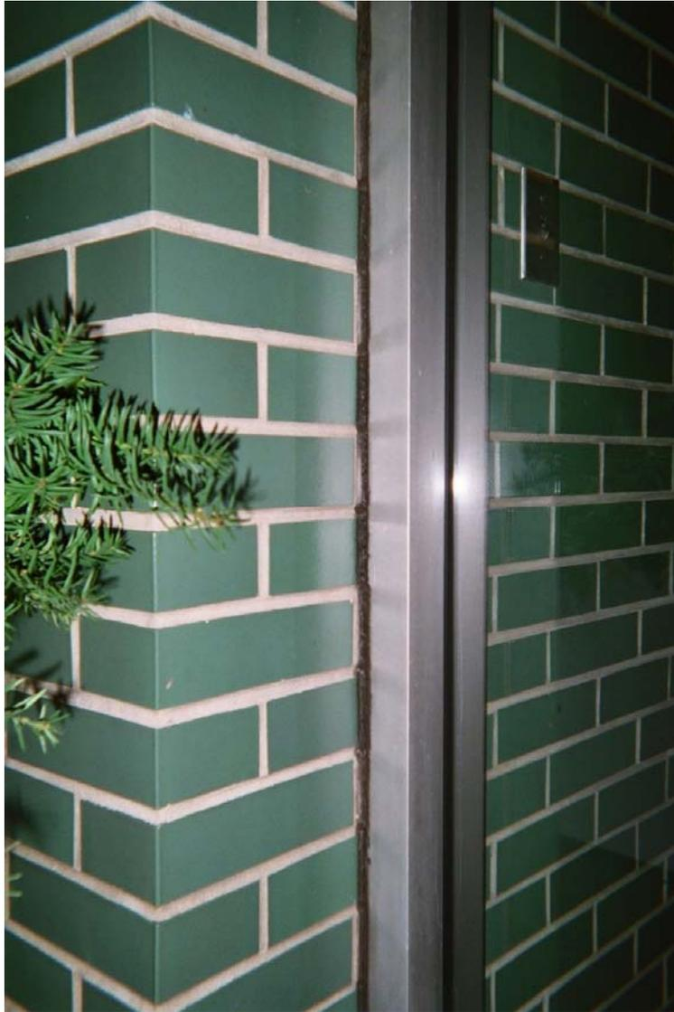
Photo 6 – Assumed asbestos-containing black building caulk compound
