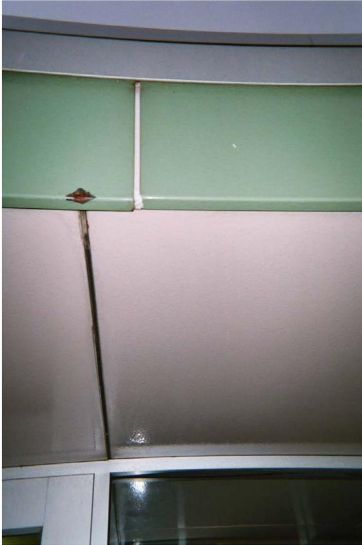
Photo 5 – Assumed asbestos-containing white and black exterior building caulk compound
