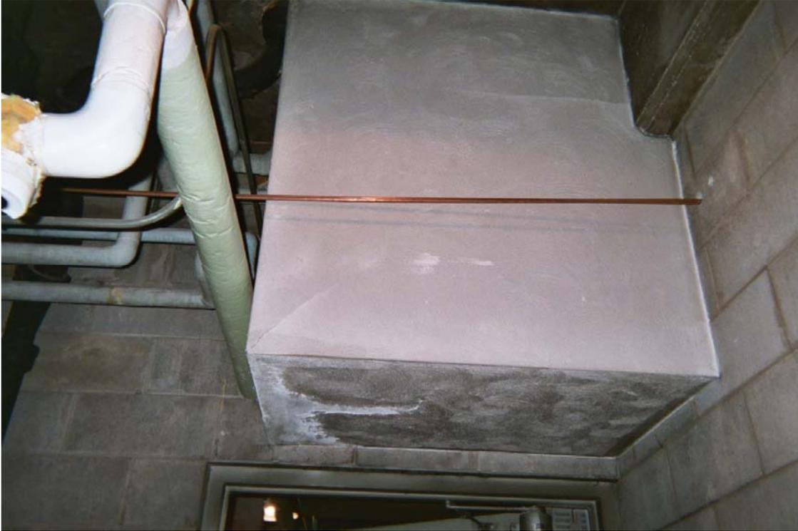
Photo 19 – Non asbestos-containing plaster over ventilation ductwork
