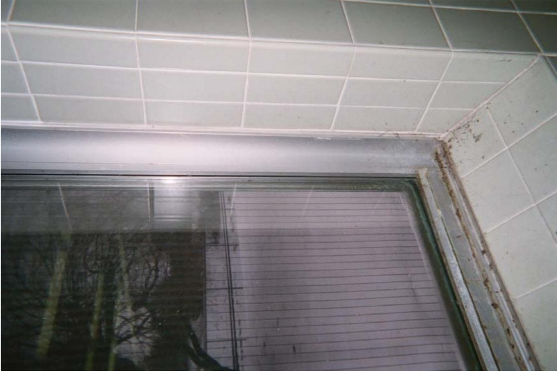
Photo 18 – Non asbestos-containing white interior window frame caulk compound
