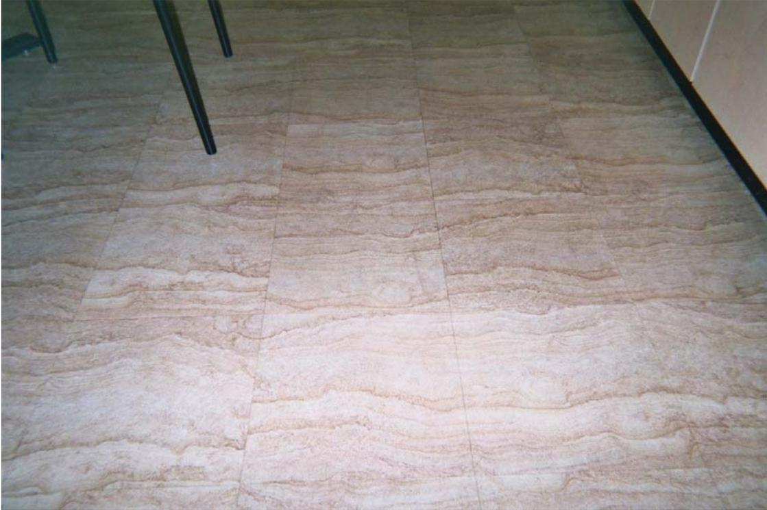
Photo 10 – Non asbestos-containing 12” x 12” cream floor tile with rust streaks and associated mastic
