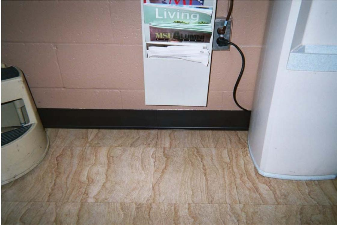
Photo 9 – Non asbestos-containing 4” black cove molding
