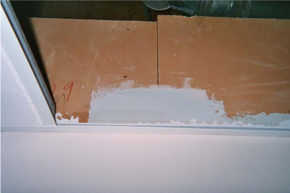
Photo 12 – Asbestos-containing drywall joint compound
