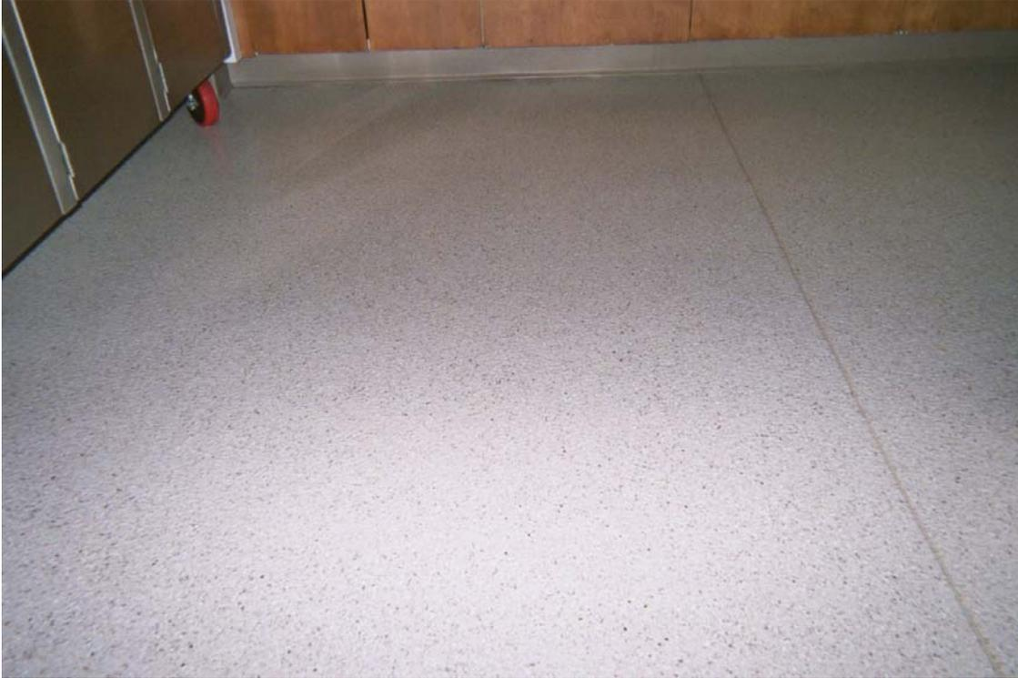
Photo 8 – Non asbestos-containing cream and vinyl flooring
