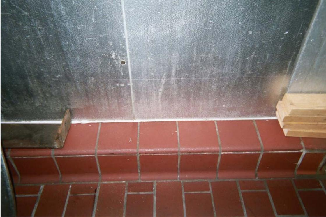
Photo 17 – Non asbestos-containing white refrigeration caulk compound
