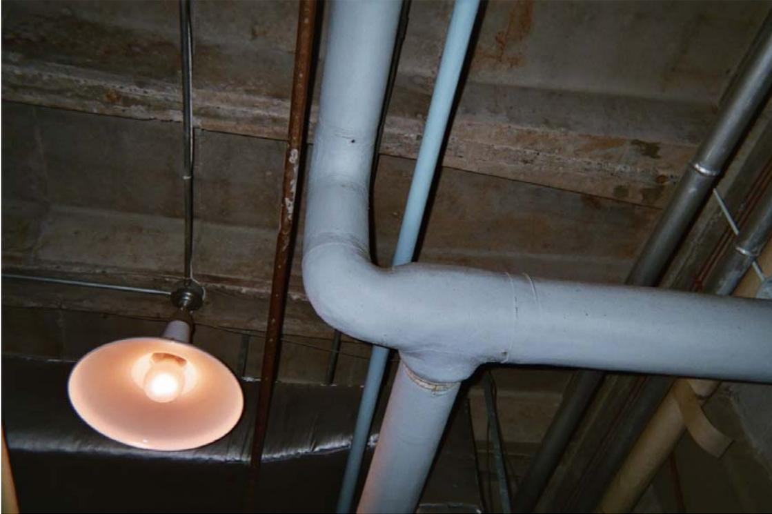
Photo 22 – Asbestos-containing domestic water pipe joint insulation
