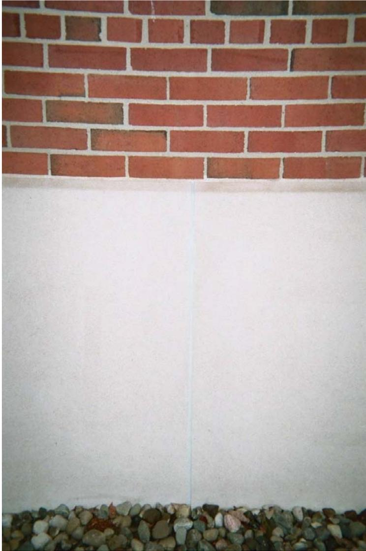
Photo 3 – Assumed asbestos-containing gray building caulk compound
