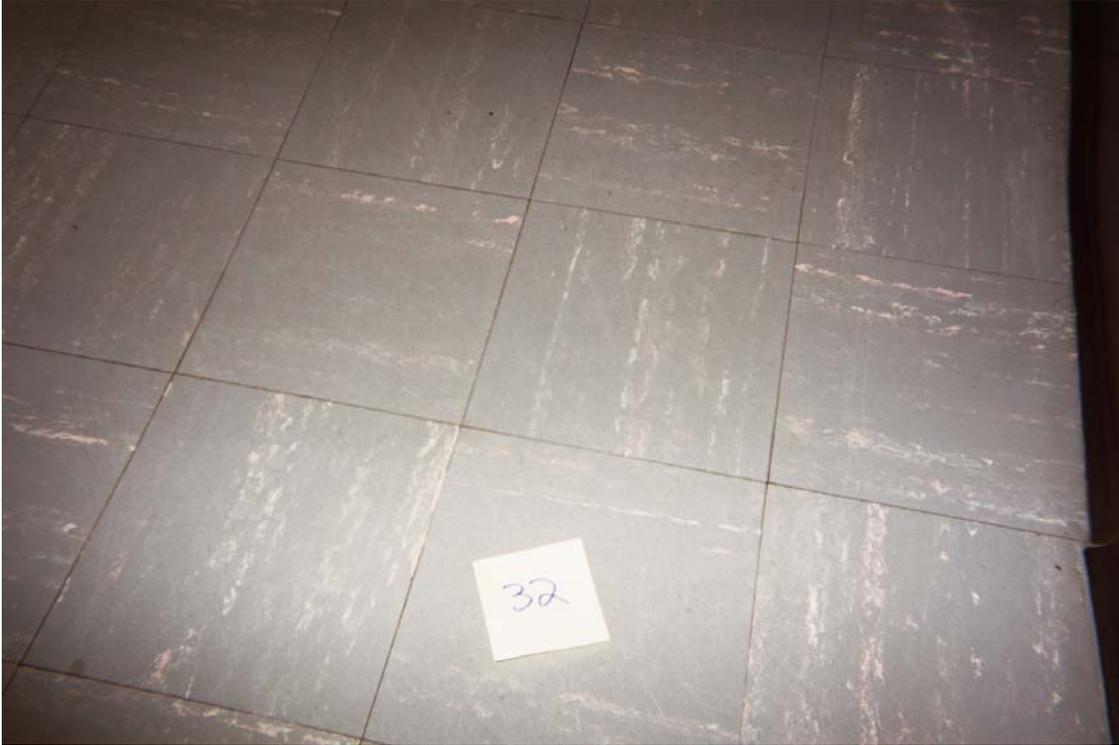
HA #33 – Asbestos-containing 9” x 9” gray floor tile with pink and cream streaks and non asbestos containing associated mastic
