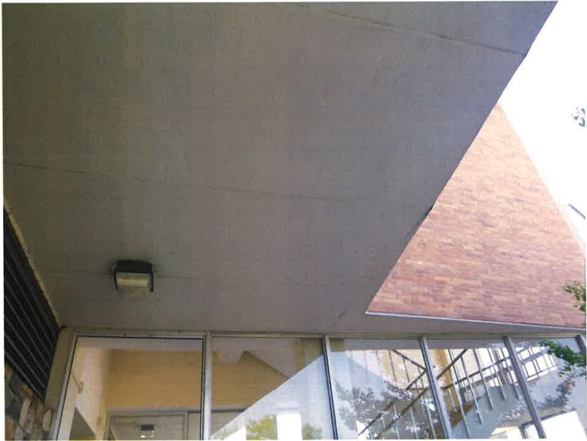
Chemistry Building HA 146 Exterior Concrete Overhang Non-Asbestos
