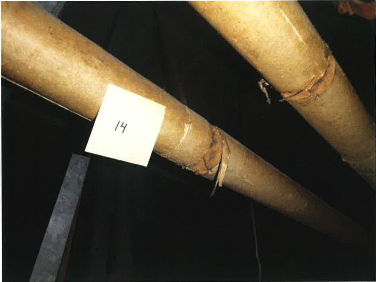
Chemistry Building HA 14 Fiberglass Pipe Insulation - Old Non-Asbestos
