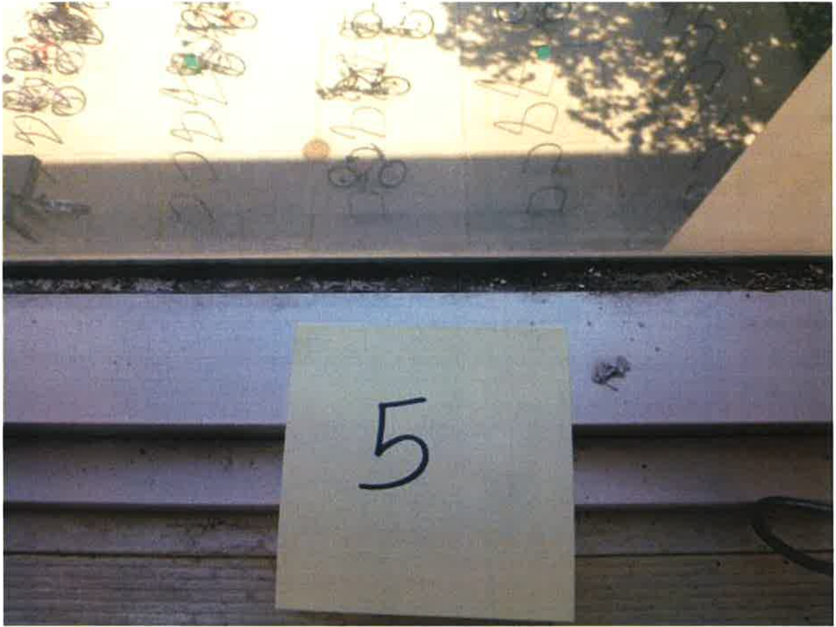
Chemistry Building HA 5 Window Glaze - Old Gray Non-Asbestos
