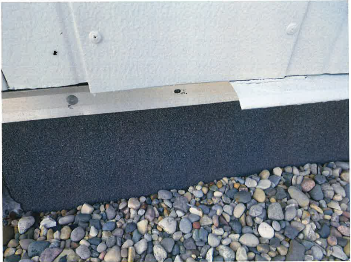
Chemistry Building HA 148 Exterior Penthouse Flashing Non-Asbestos
