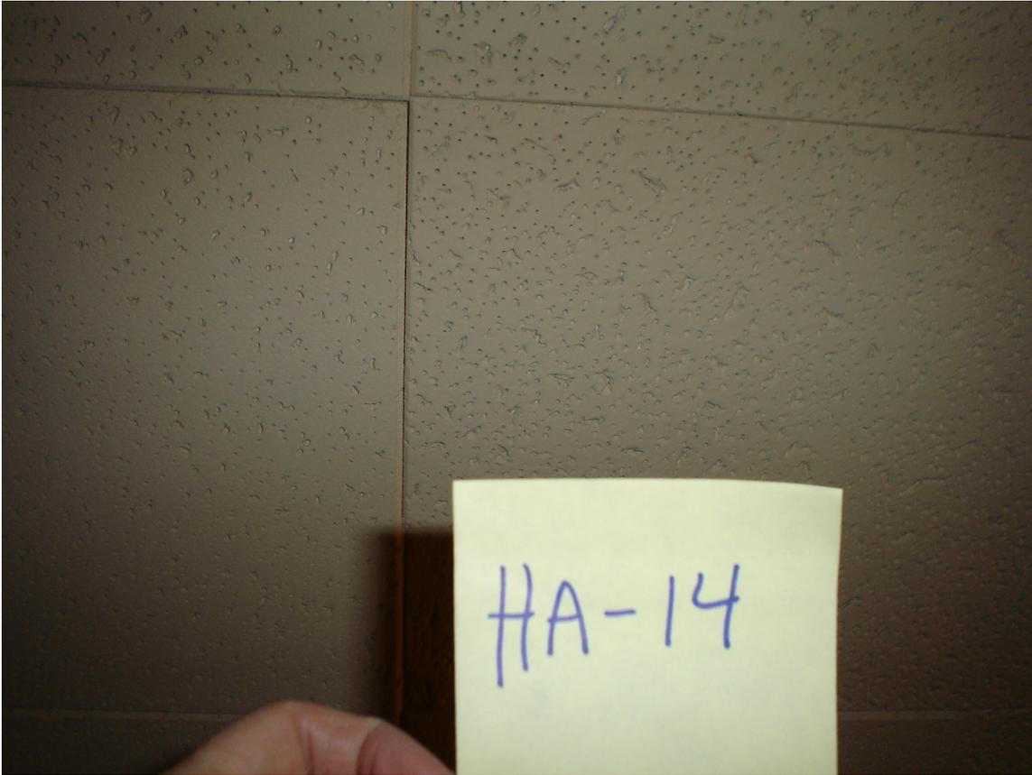
HA #14 – Non asbestos containing 12” x 12” light brown textured glued-on ceiling tile and associated glue pods
