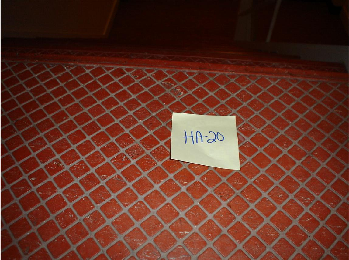
HA #20 – Asbestos containing red stair tread and associated non asbestos containing mastic
