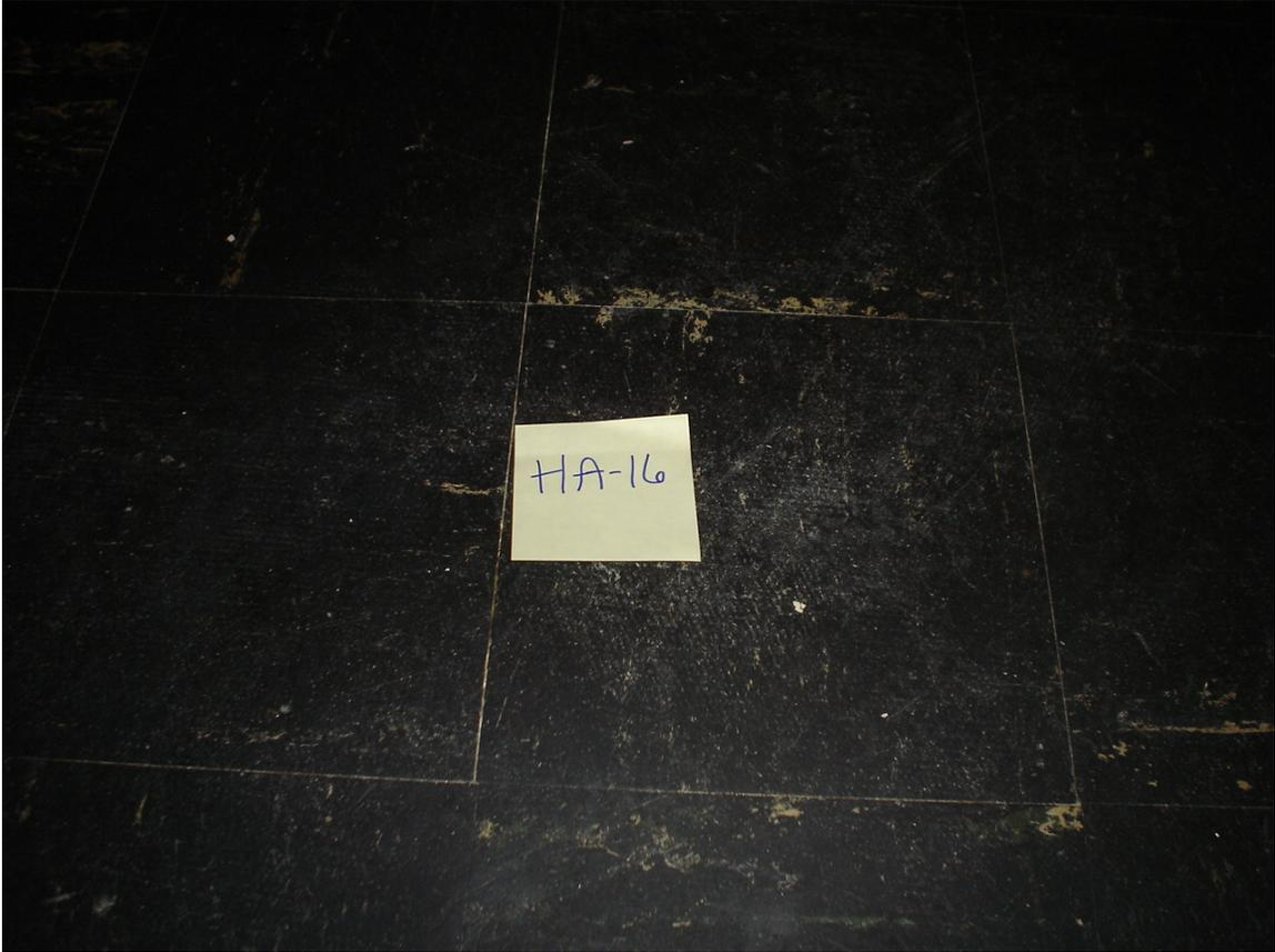
HA #16 – Asbestos containing 9” x 9” black floor tile with white streaks and associated non asbestos containing mastic
