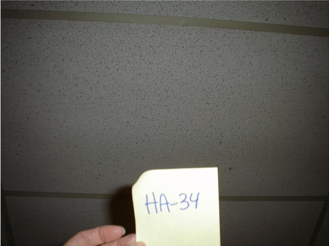
HA #34 – Non asbestos containing 2' x 4' white drop in ceiling tile
