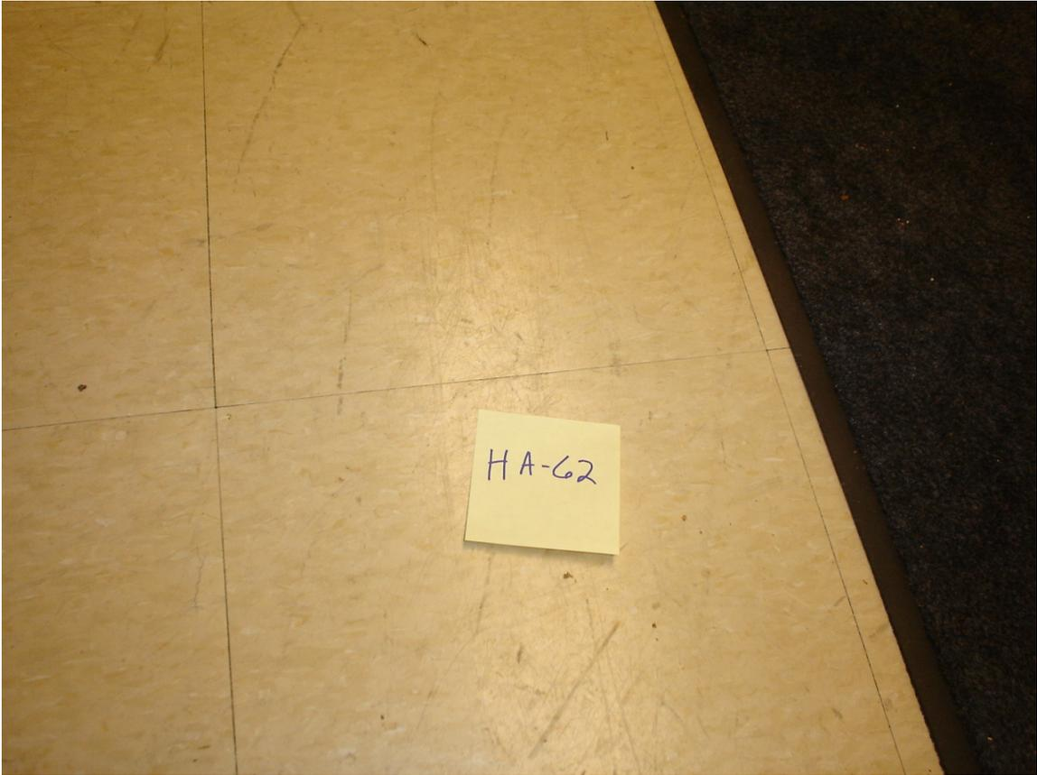
HA #62 – Non asbestos containing 12” x 12” white floor tile with brown and white streaks and associated asbestos containing mastic
