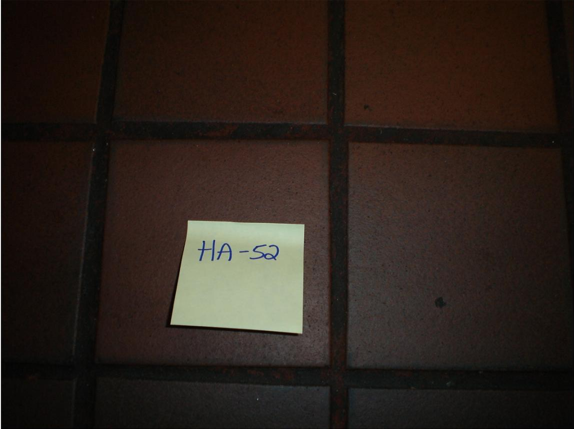
HA #52 – Non asbestos containing red ceramic floor
