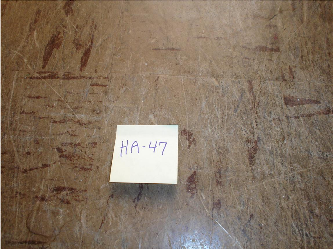
HA #47 – Asbestos containing 9” x 9” brown floor tile with brown and white streaks and associated non asbestos containing mastic
