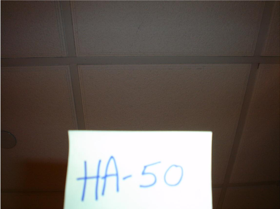
HA #50 – Non asbestos containing 2' x 2' white drop in ceiling tile with pin holes
