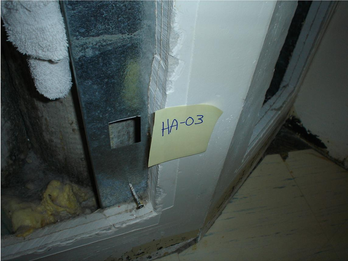
HA #3 – Non asbestos containing drywall with plaster skim coat
