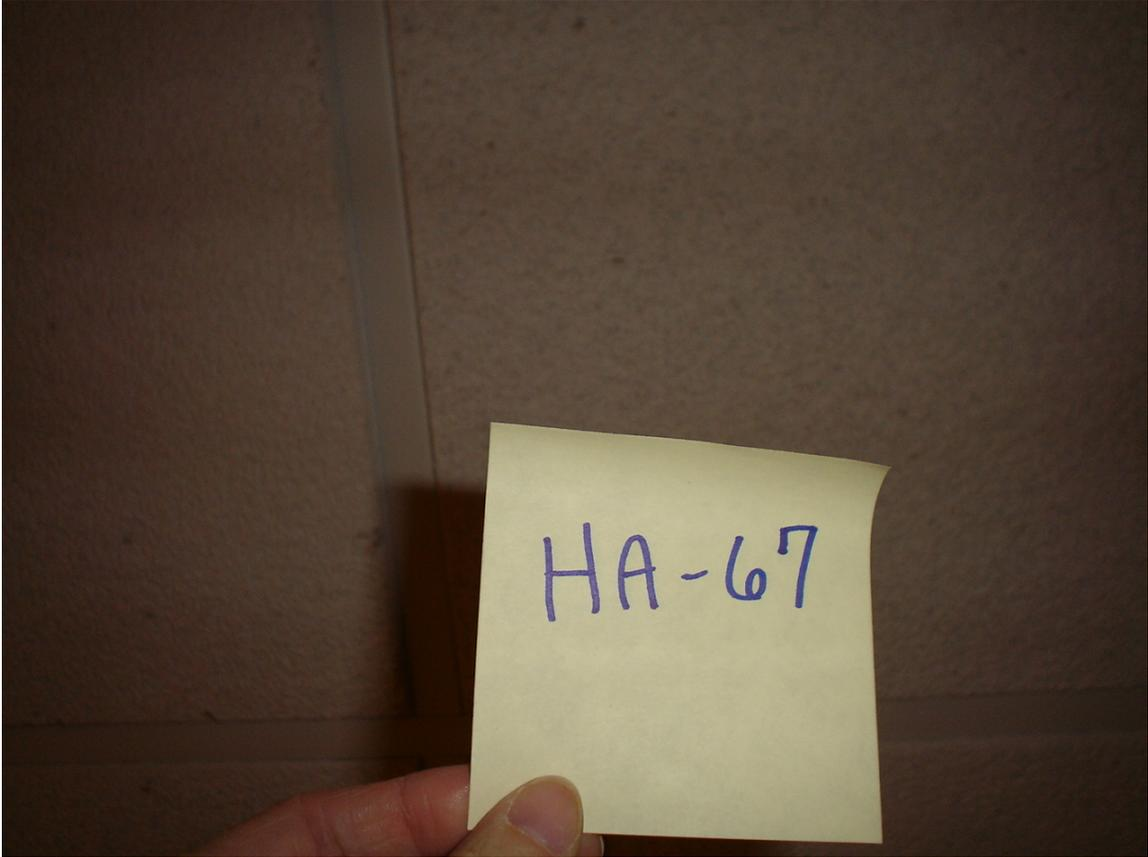
HA #67 – Non asbestos containing 2' x 2' white small textured drop ceiling tile
