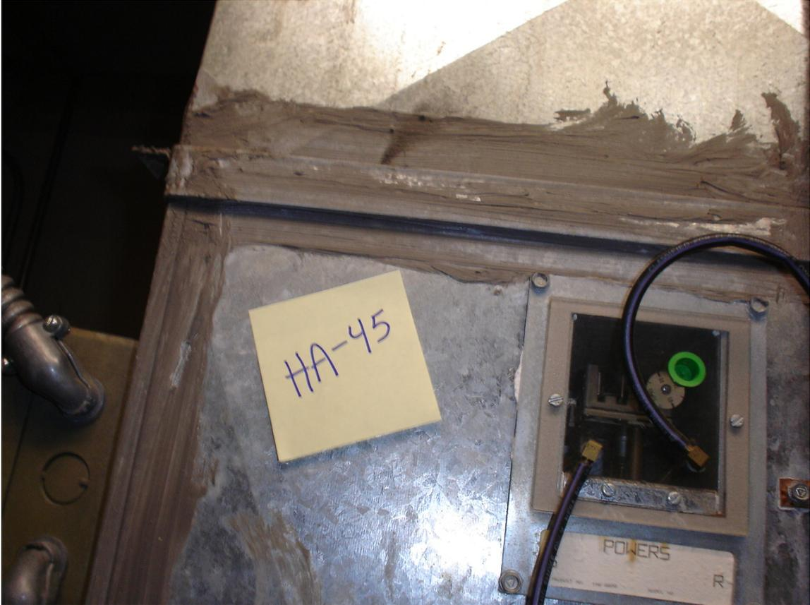
HA #45 – Non asbestos containing gray duct caulk
