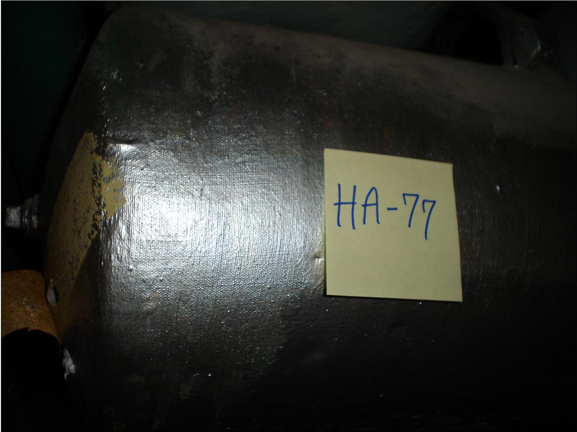
HA #77 – Asbestos containing tank insulation
