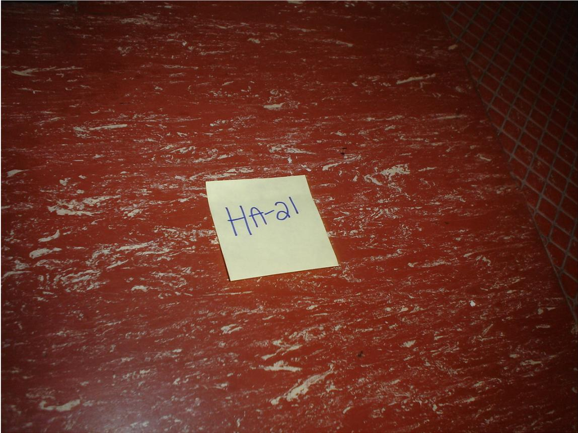
HA #21 – Non asbestos containing red linoleum with white streaks
