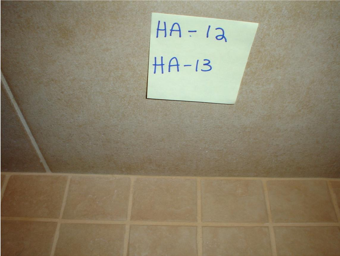
HA #12 – Non asbestos containing 2” x 2” light brown ceramic floor tile bedding compound
