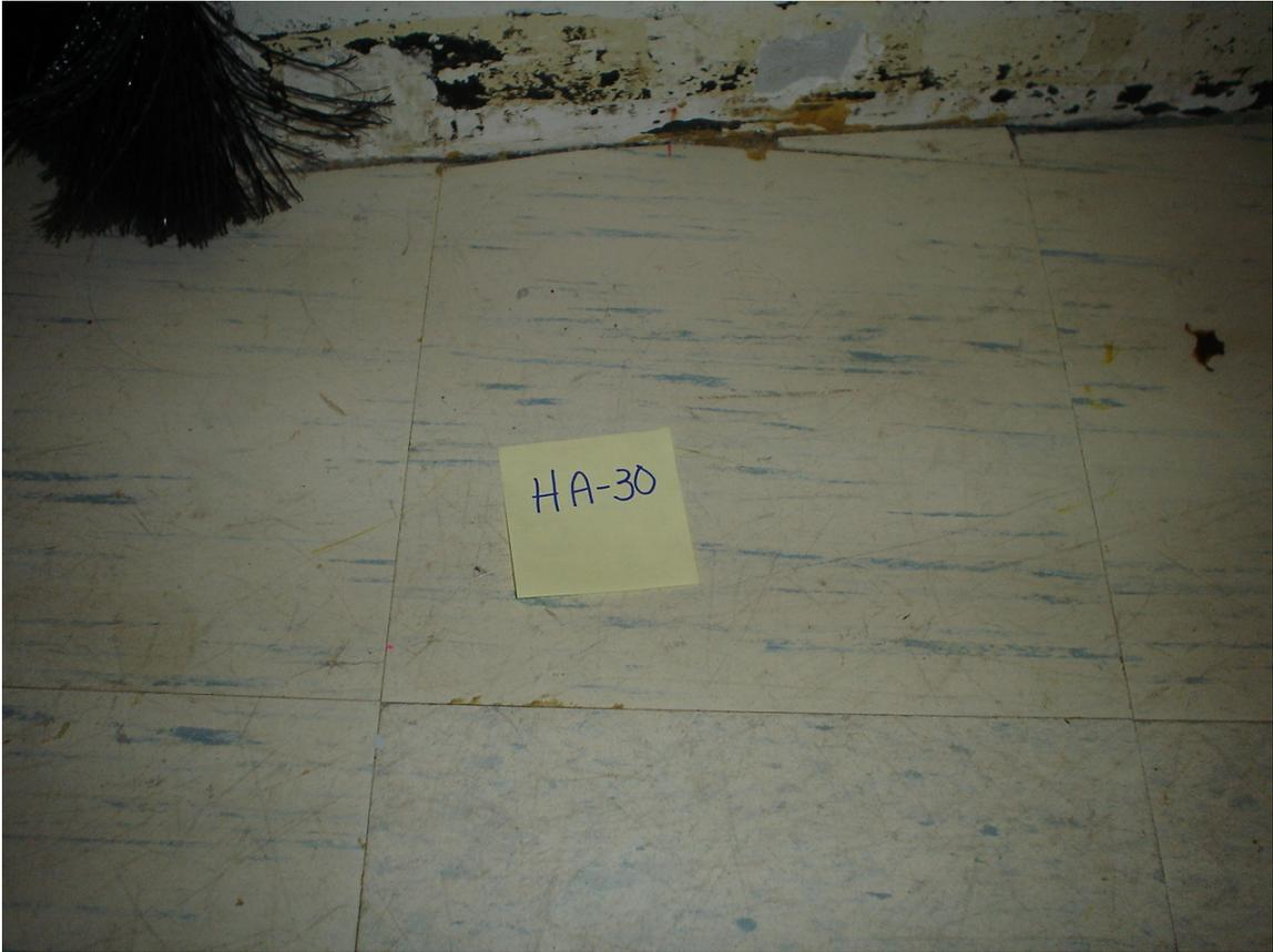
HA #30 – Non asbestos containing white floor tile with blue streaks and associated mastic
