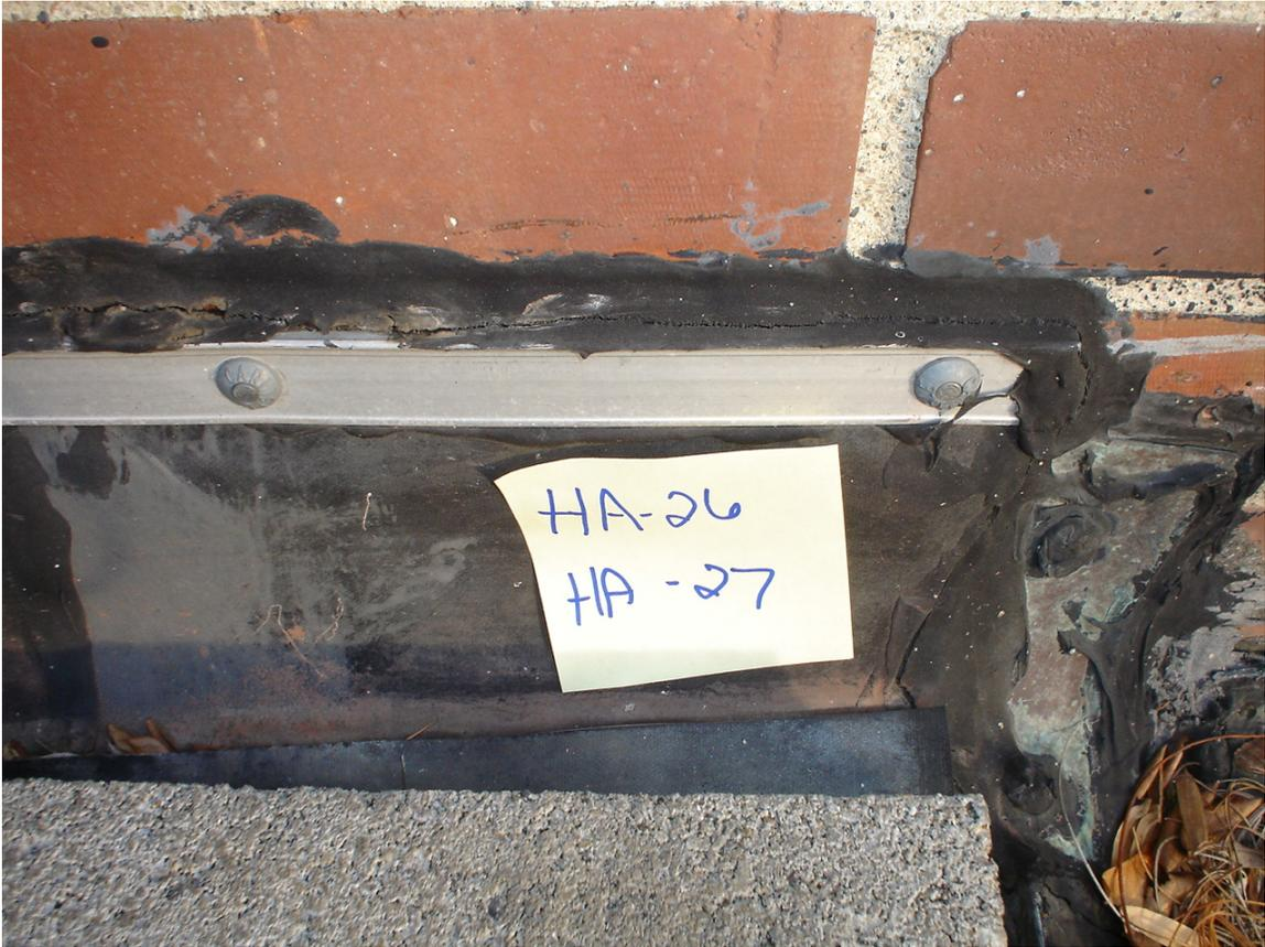
HA #26 – Assumed asbestos containing black roof flashing
