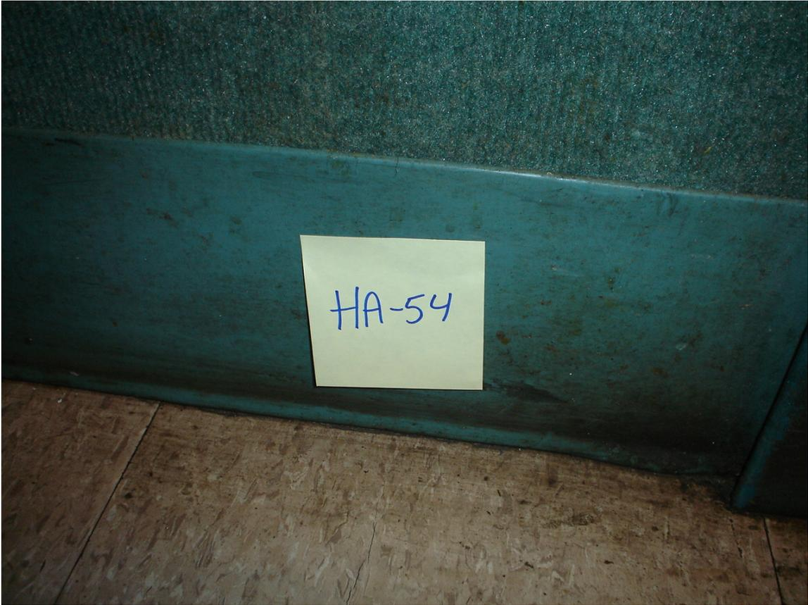
HA # 54 – Non asbestos containing 6” green cove molding and associated mastic
