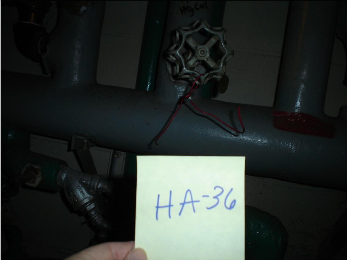
HA #36 – Asbestos containing steam pipe joint insulation
