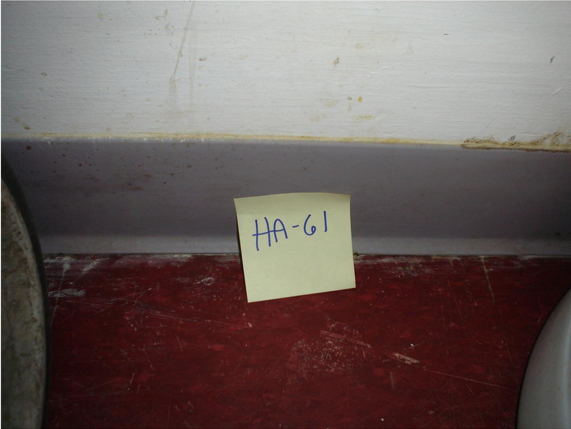
HA #61 – Non asbestos containing 4” gray cove molding and associated mastic
