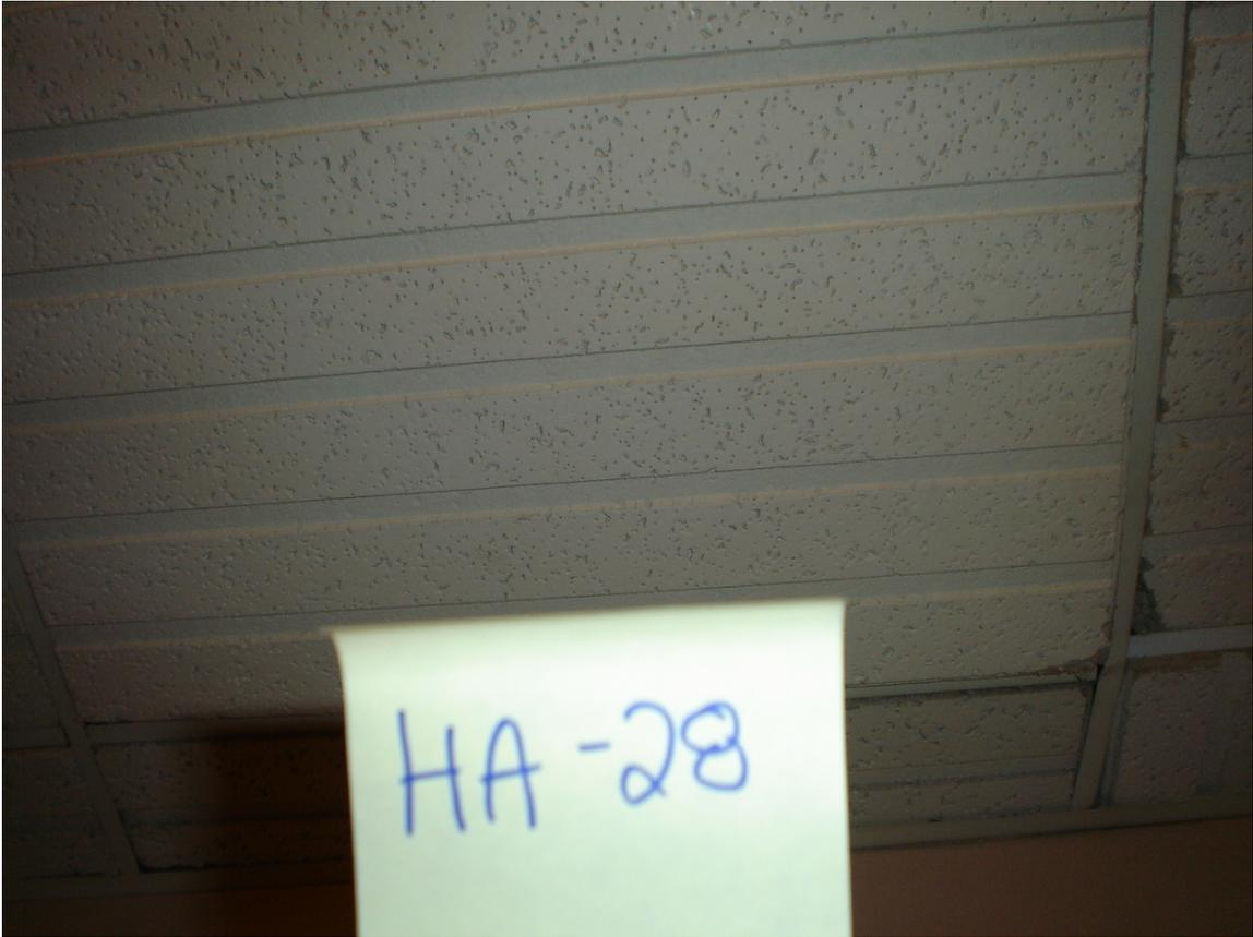
HA # 28 – Non asbestos containing 2' x 2' white lined drop ceiling tile
