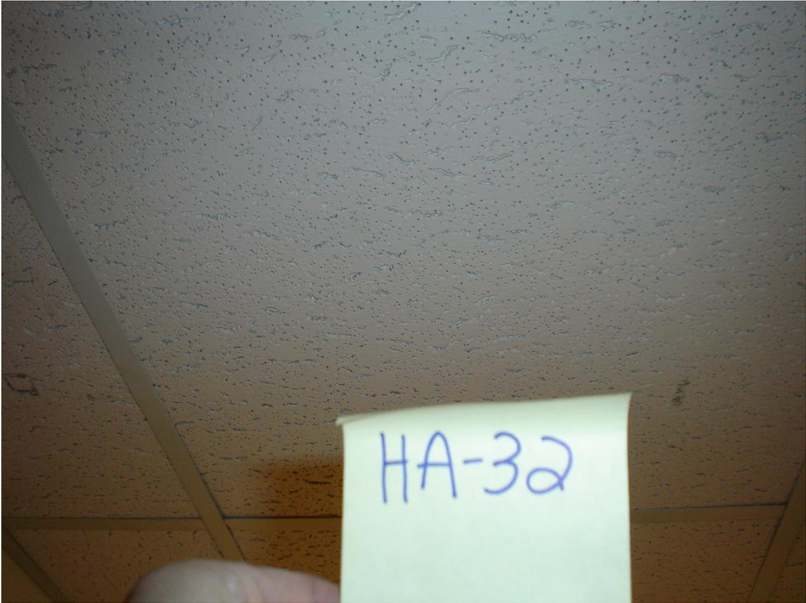
HA #32 – Non asbestos containing 2' x 2' white lay-in ceiling tile with pin holes and fissures
