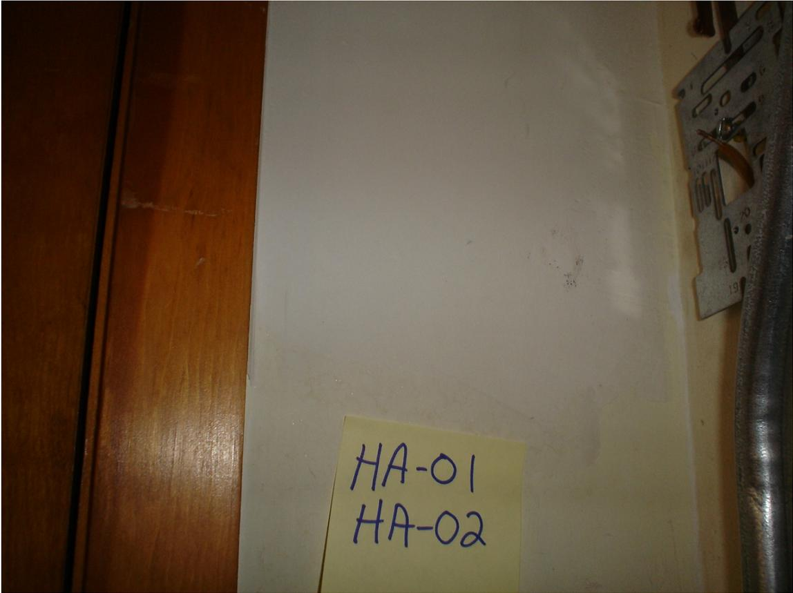
HA #1 – Non asbestos containing drywall
