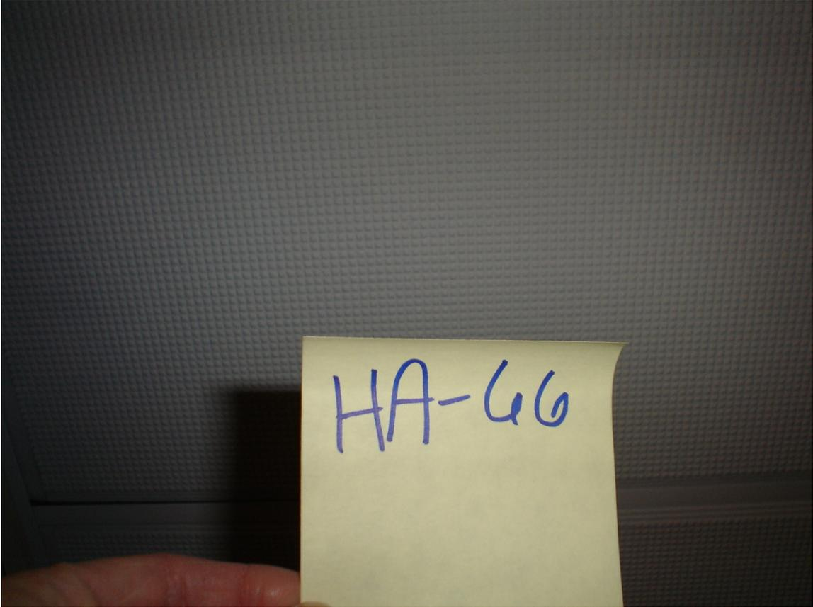
HA #66 – Non asbestos containing 2' x 2' white drop-in ceiling tile with tiny squares
