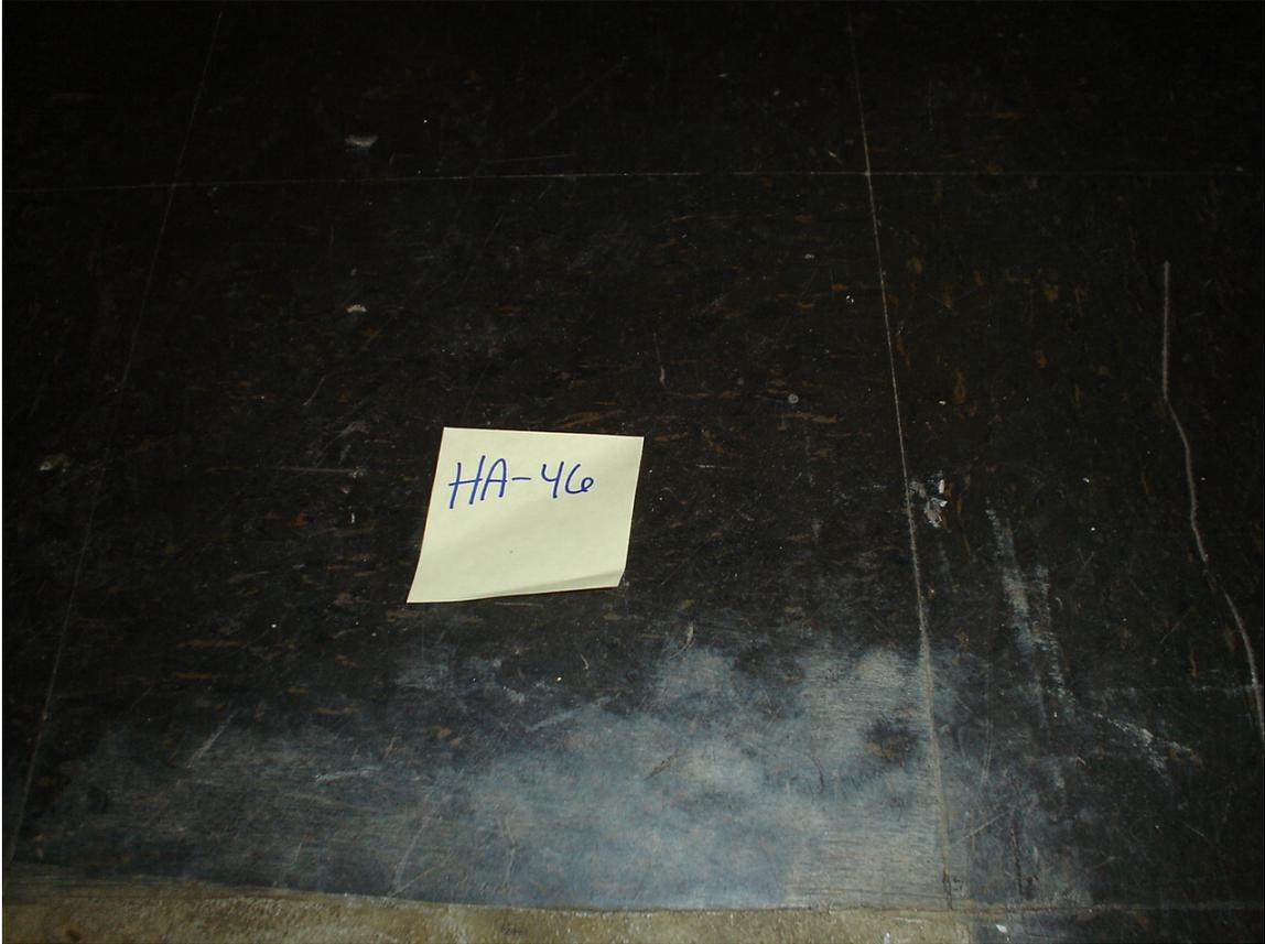
HA #46 – Asbestos containing 12” x 12” black floor tile with brown streaks and associated mastic
