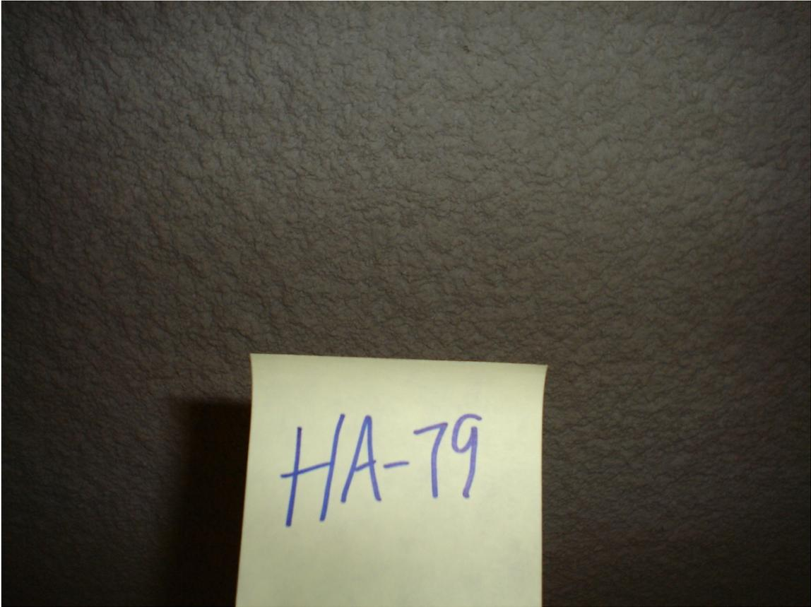
HA #79 – Non asbestos containing white acoustical ceiling
