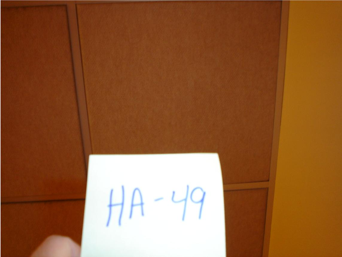
HA #49 – Non asbestos containing 2' x 2' off-white fuzzy drop-in ceiling tile
