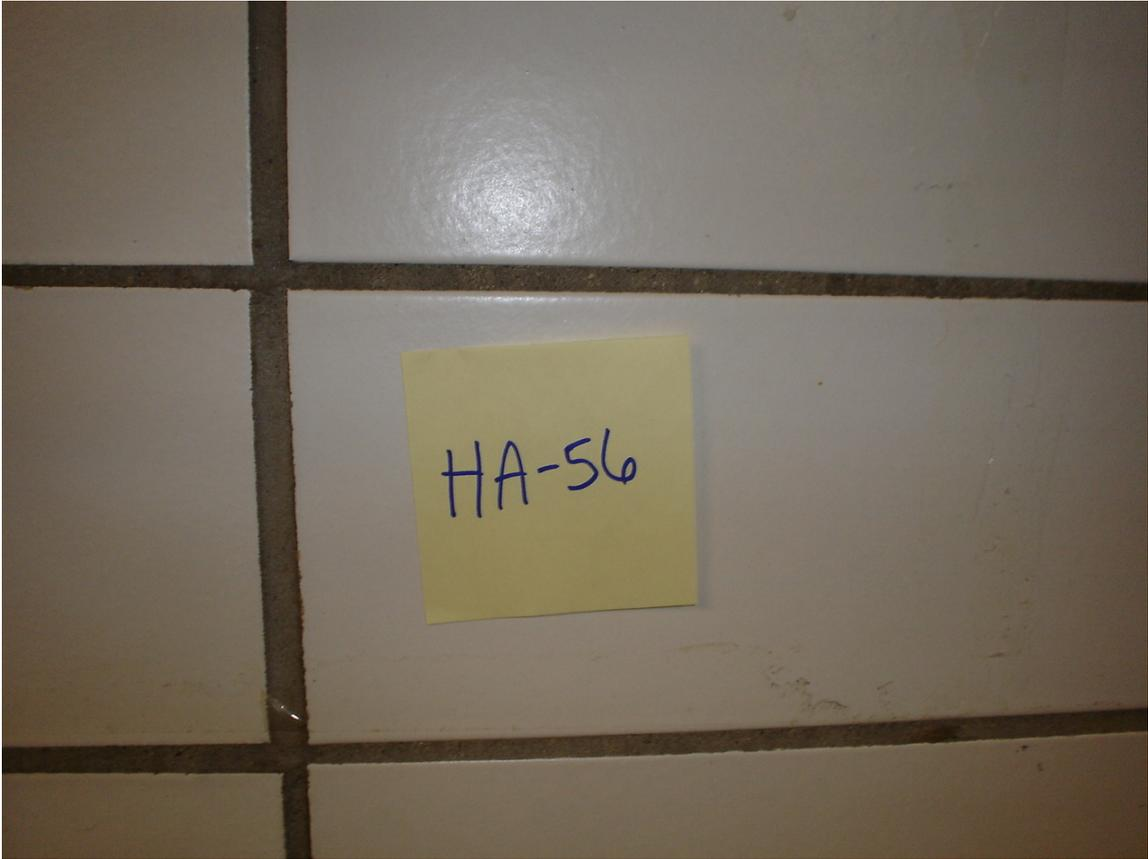
HA #56 – Non asbestos containing white ceramic wall tile
