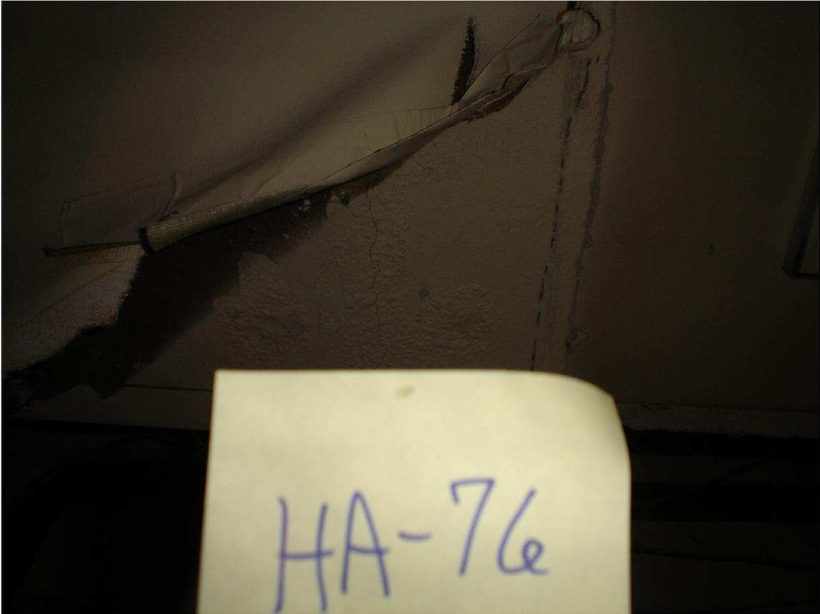
HA #76 – Non asbestos containing duct insulation
