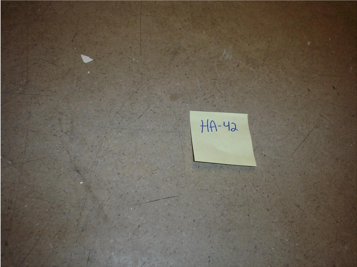
HA #42 – Non asbestos containing tan linoleum and associated mastic
