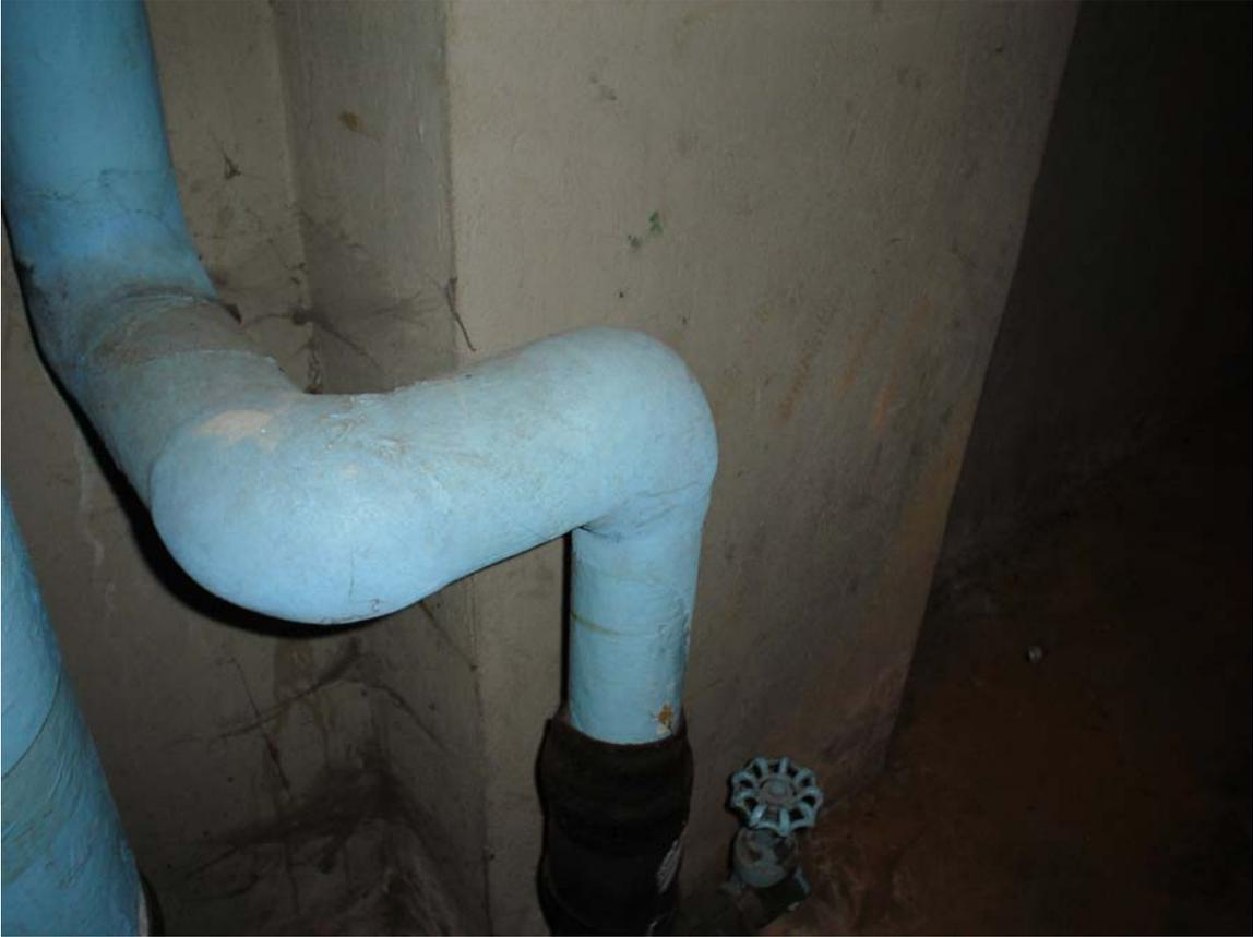
HA #4 – Asbestos containing domestic water supply pipe joint and hanger insulation
