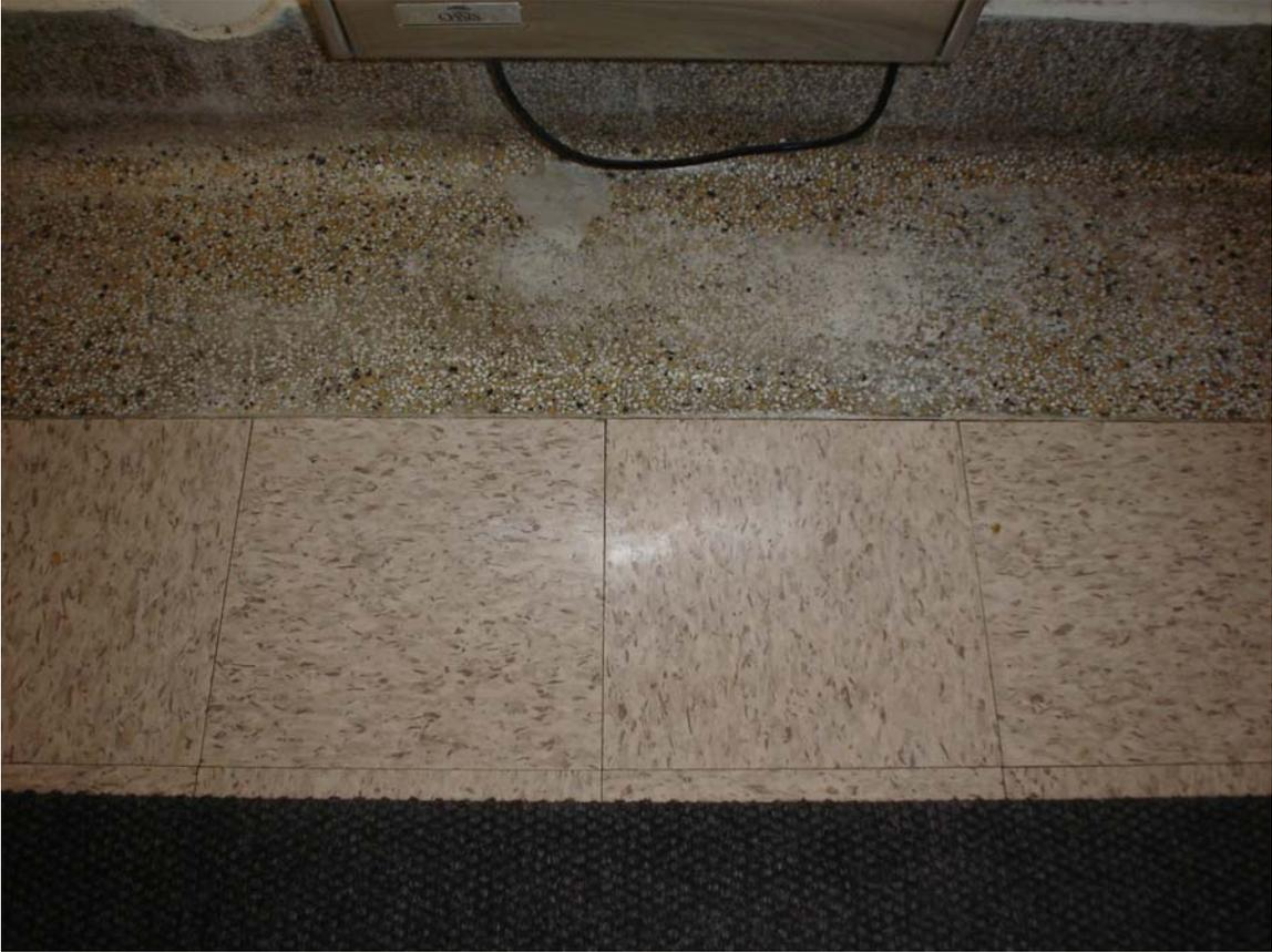
HA #2 – Non asbestos 12” x 12” tan marble pattern floor tile and associated asbestos containing mastic
