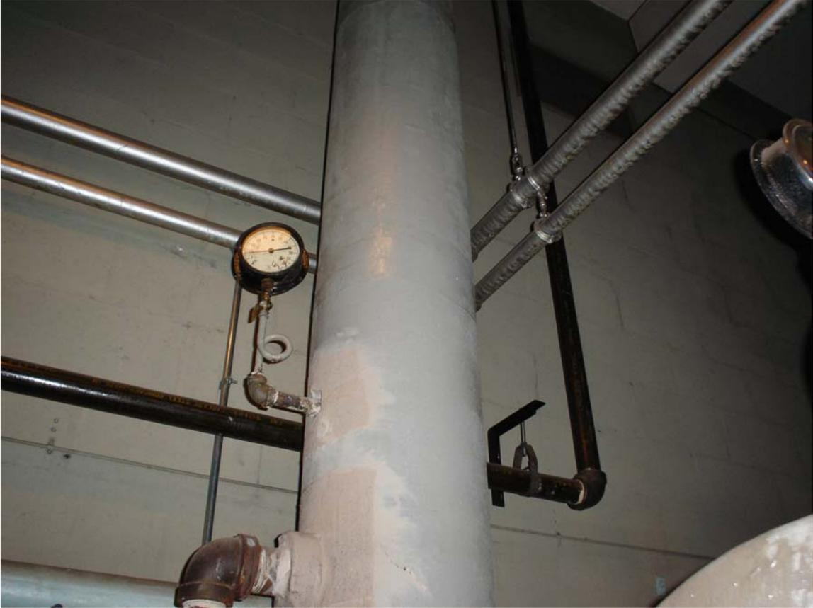
HA #5 – Asbestos containing steam/condensate supply and return pipe straight insulation
