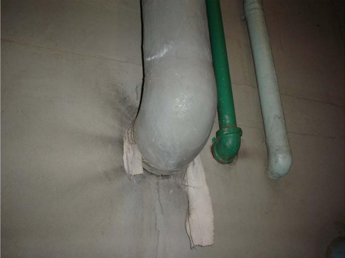
HA #6 – Asbestos containing steam/condensate supply
