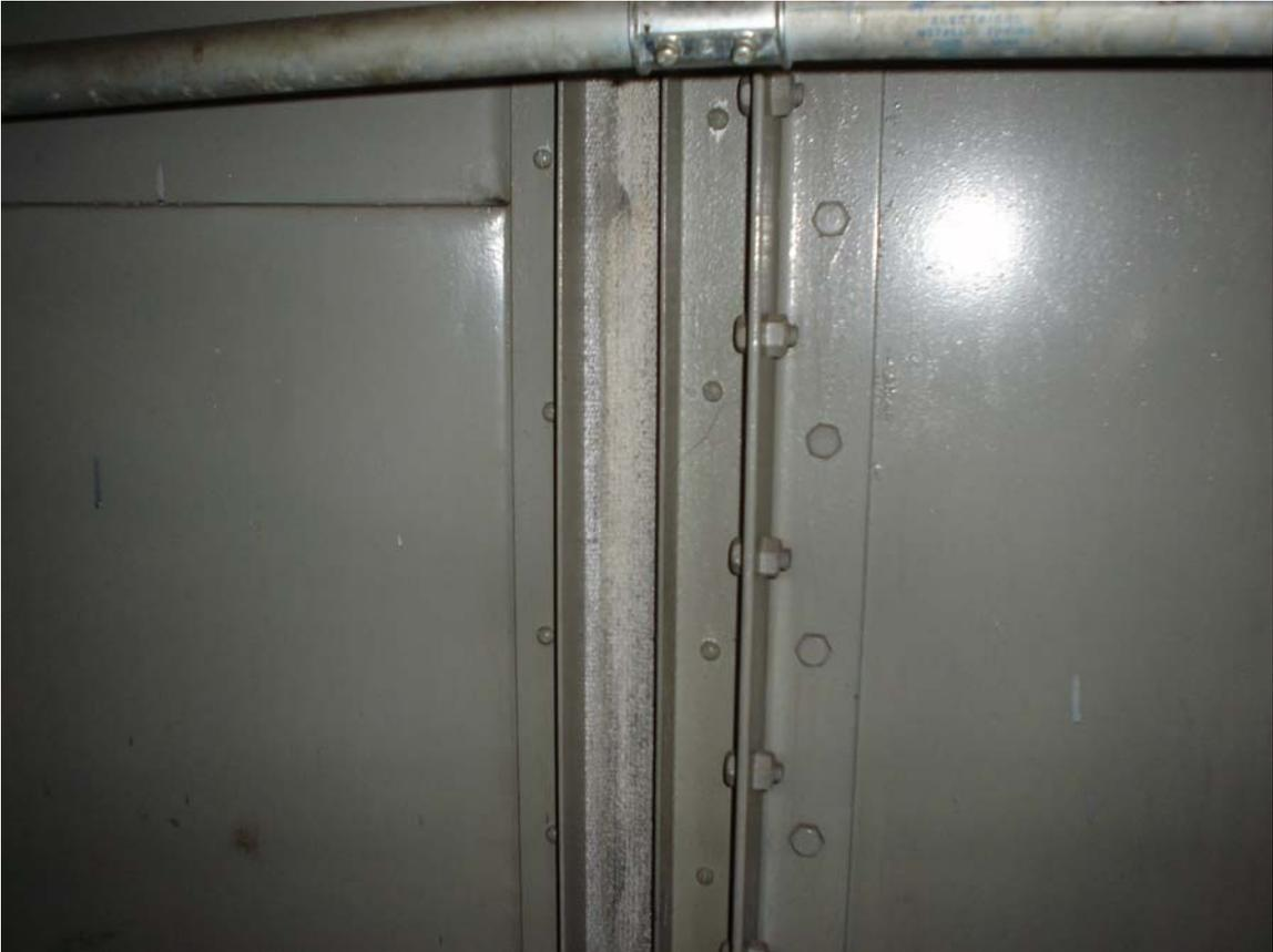
HA #8 – Asbestos containing ventilation duct expansion cloth
