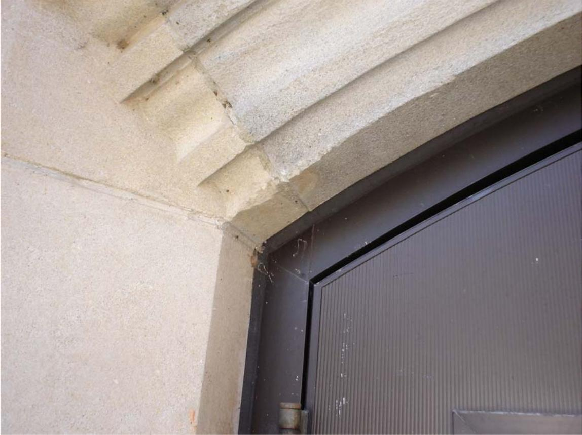
HA #46 – Assumed asbestos containing window and door frame caulk compound
