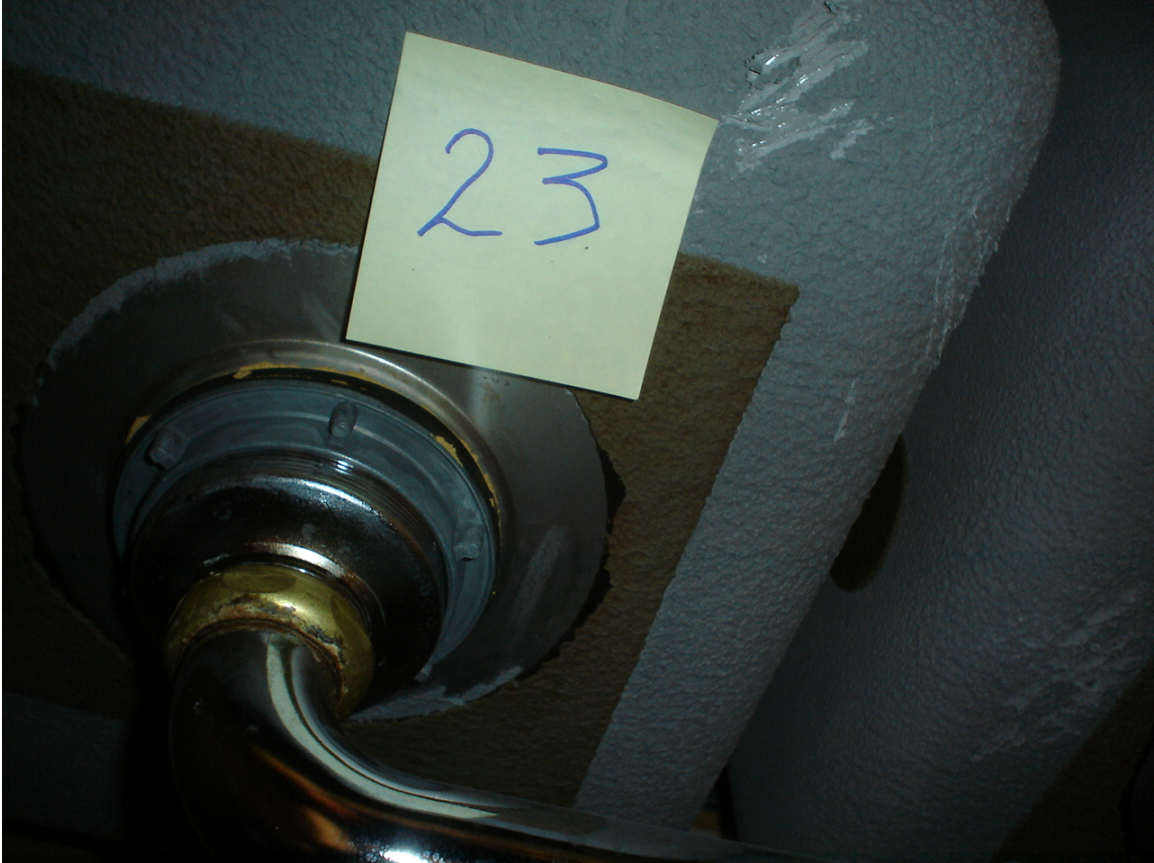
HA #23 – Non asbestos-containing gray sink undercoating
