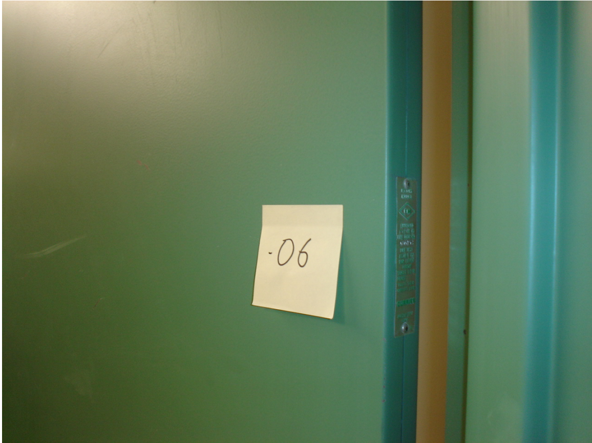
HA #6 – Assumed asbestos-containing fire door and frame
