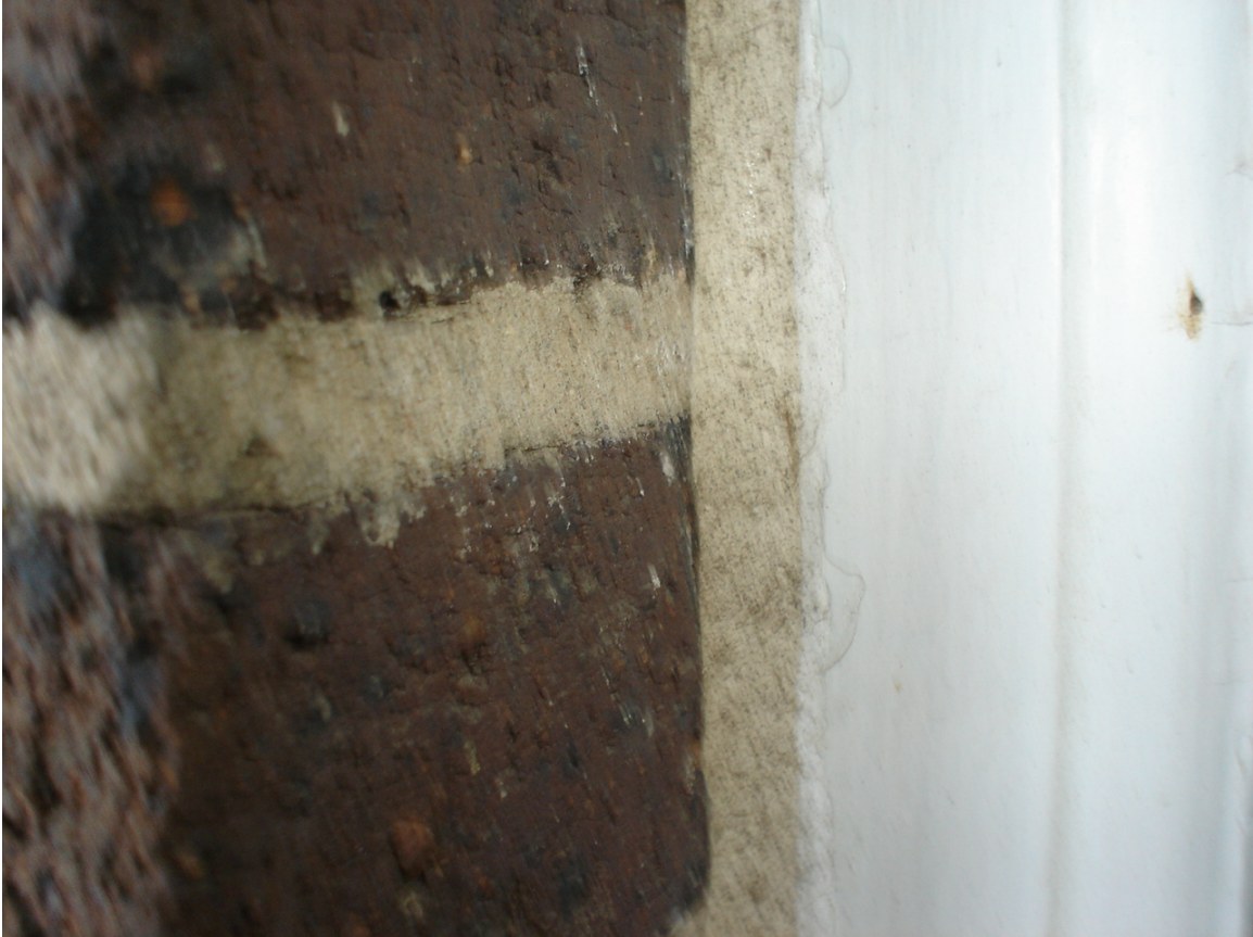
HA #8 – Assumed asbestos-containing window and door frame caulk compound
