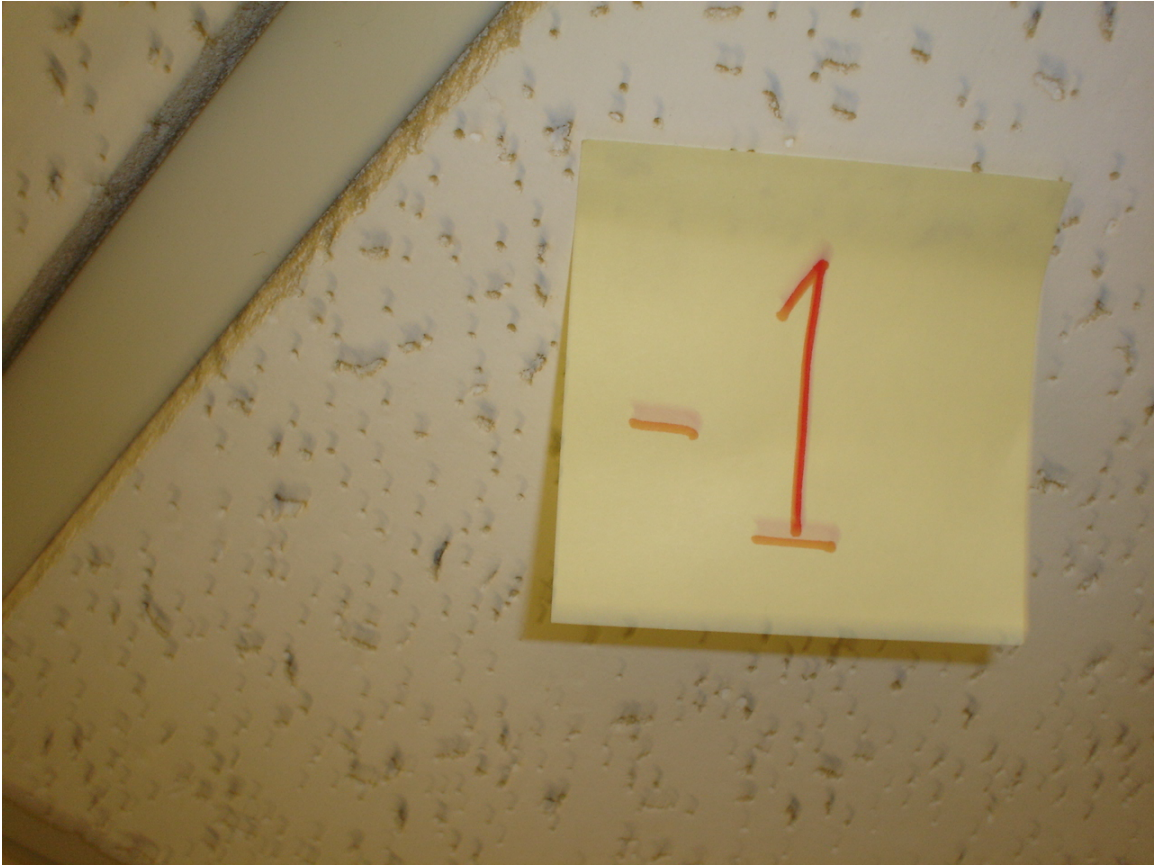
HA #1 – Non asbestos-containing 2' x 2' white drop-in ceiling tile with pin holes and fissures
