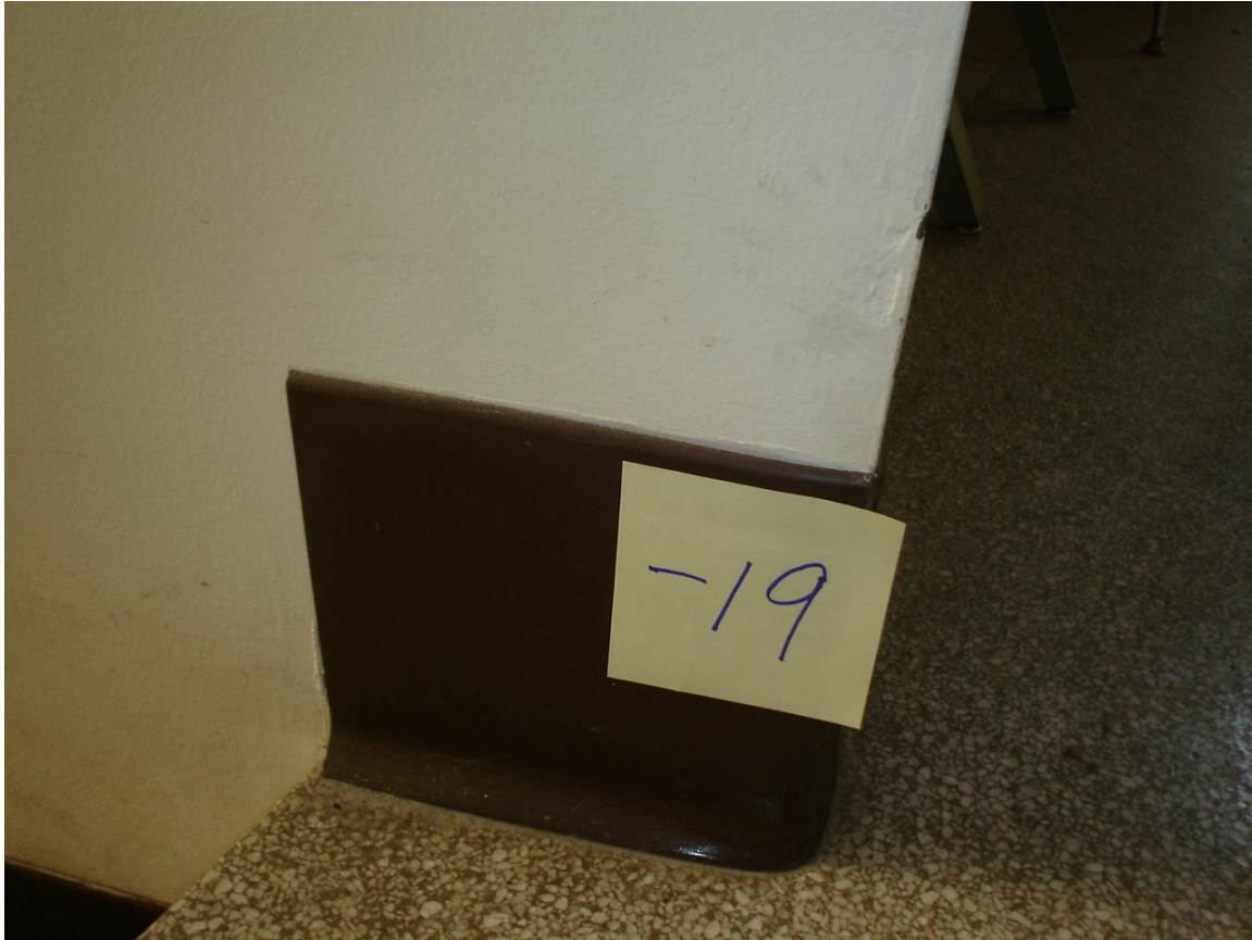
HA #19 – Non asbestos-containing 6" brown cove molding and associated mastic
