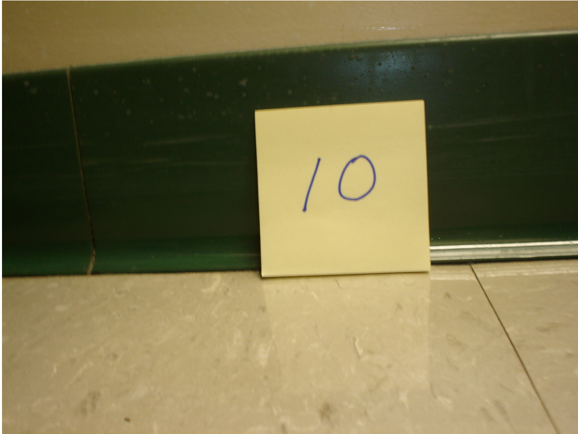
HA #10 – Non asbestos-containing 4" green cove molding and associated mastic
