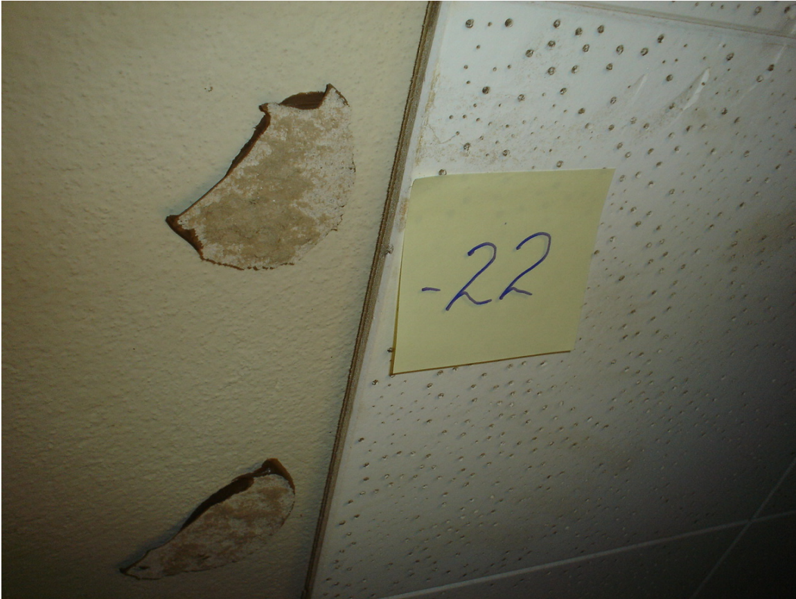
HA #22 – Non asbestos-containing 12" x 12" white ceiling tile with pin holes and associated glue pods
