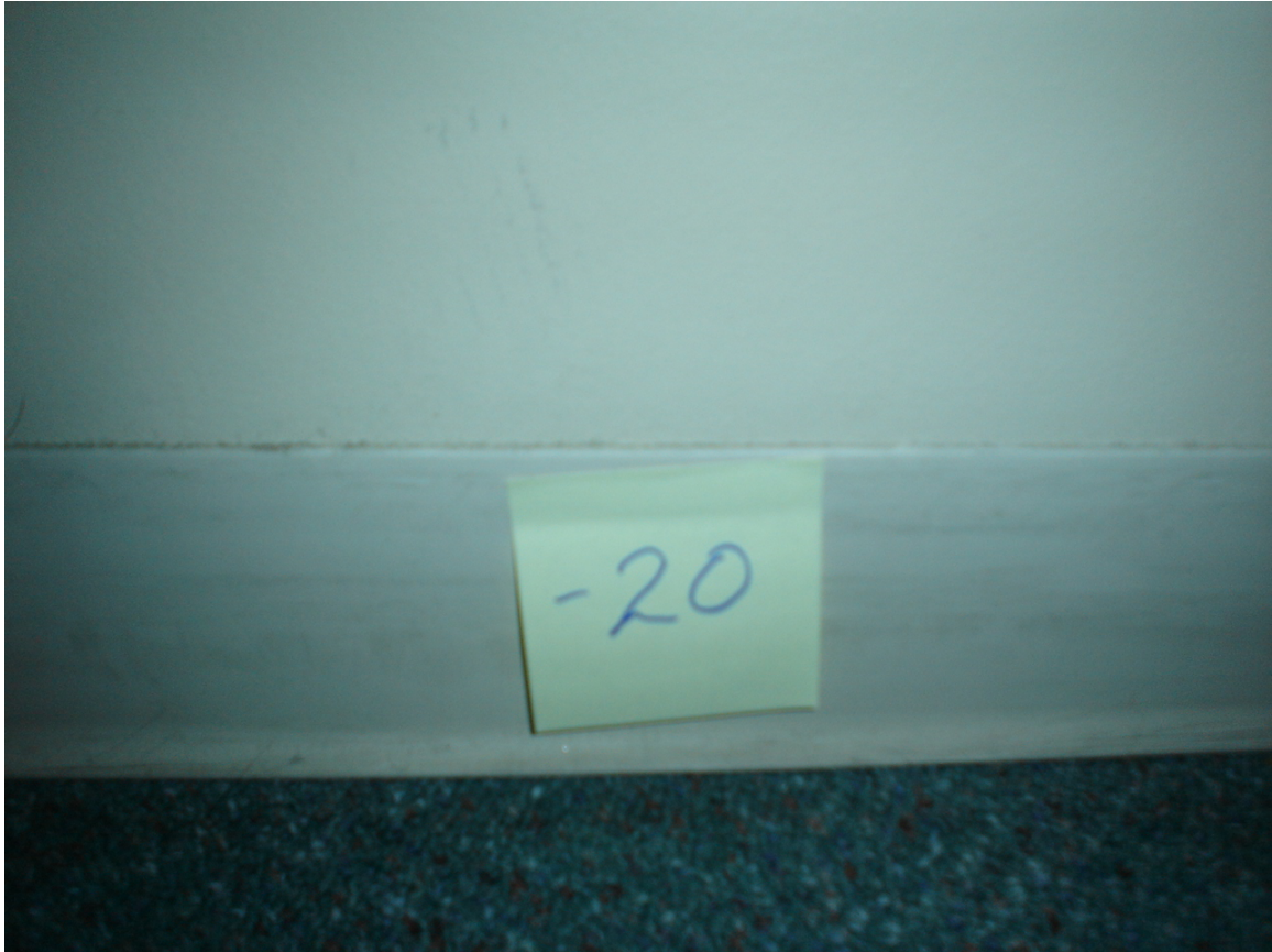
HA #20 – Non asbestos-containing 4" white cove molding and associated mastic
