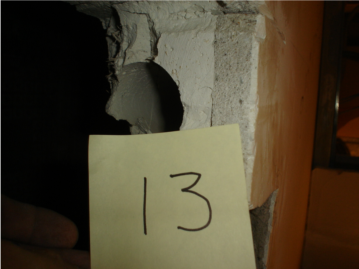
HA #13 – Non asbestos-containing pyrobar fire block
