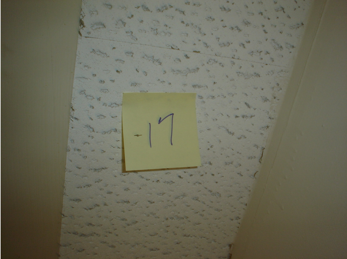
HA #17 – Non asbestos-containing 12" x 12" white ceiling tile with pin holes and fissures and associated glue pods
