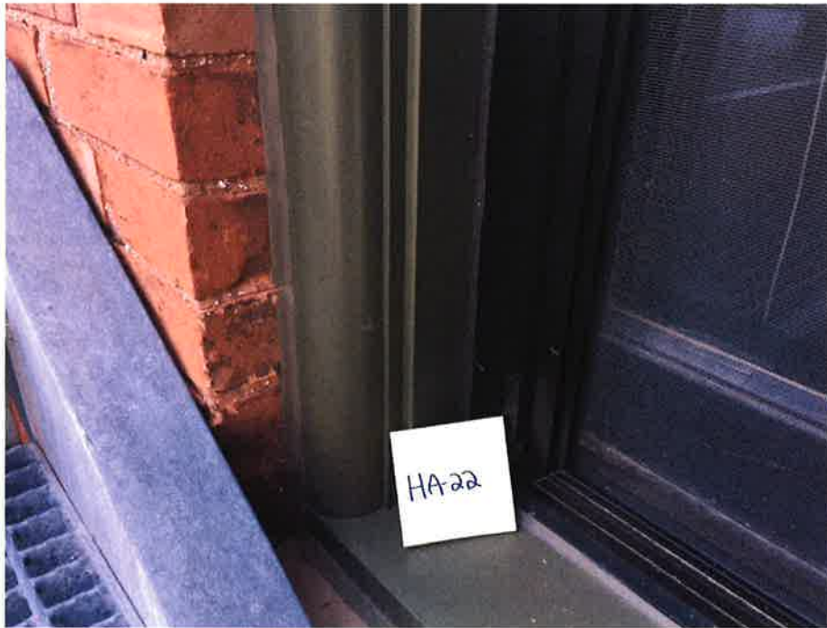
HA-22 Non-asbestos containing exterior black window caulk
