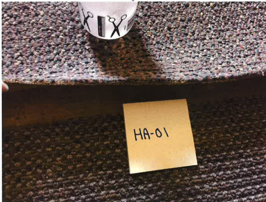
HA-01 Non-asbestos containing yellow carpet mastic
