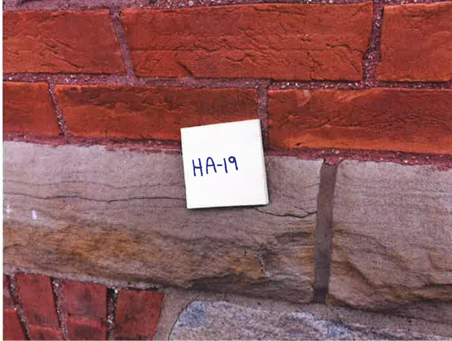
HA-19 Non-asbestos containing exterior brown building caulk
