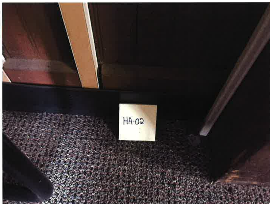
HA-02 Non-asbestos containing 4" black cove molding and associated mastic
