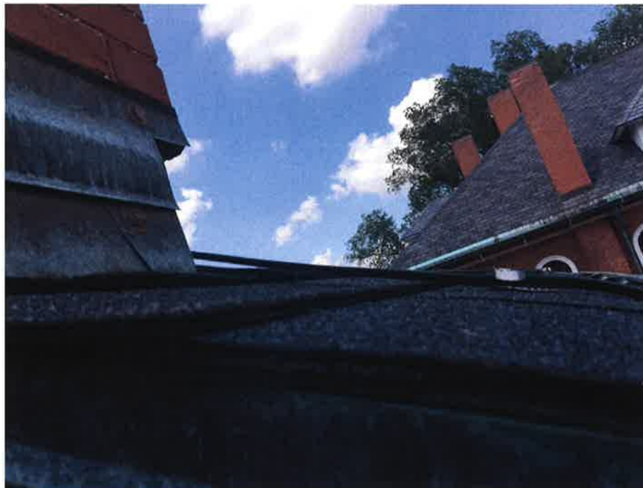
HA-16 Assumed asbestos-containing black roof shingles and tar paper
