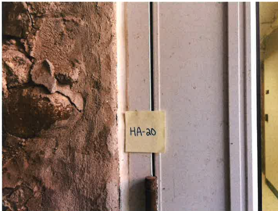
HA-20 Non-asbestos containing exterior white rubber door frame caulk
