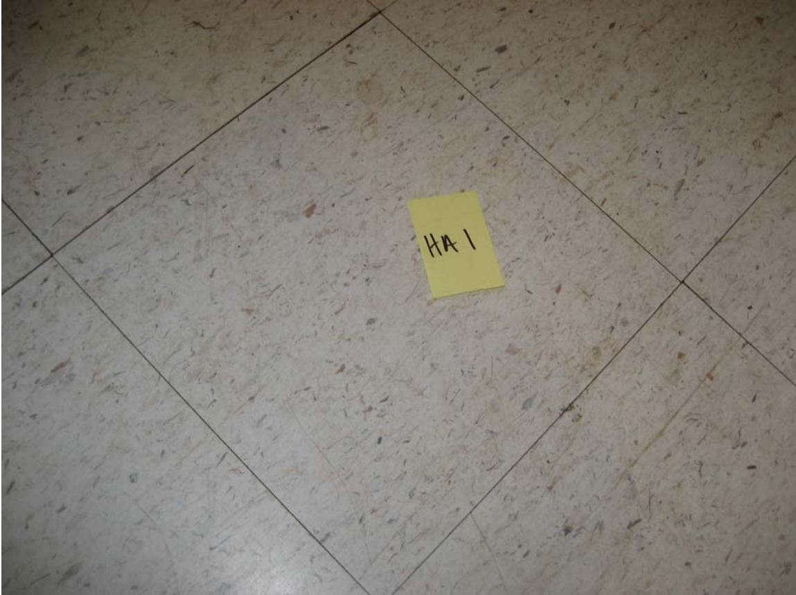
HA #1 – Non asbestos containing 12”x 12” White floor tile with gray and red streaks and associated mastic
