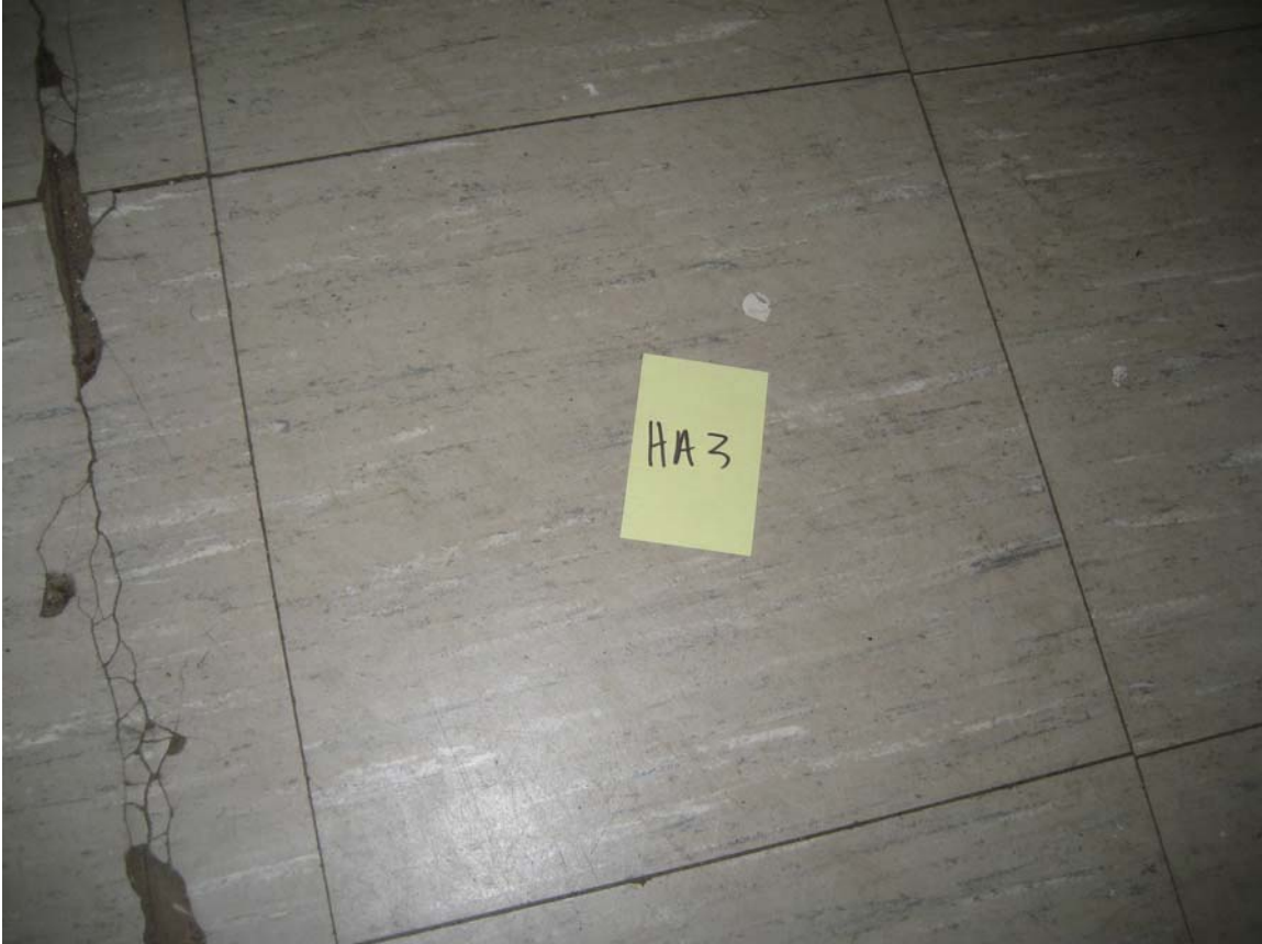
HA #3 – Non asbestos containing 12”x 12” Gray floor tile with dark gray and white streaks and associated mastic
