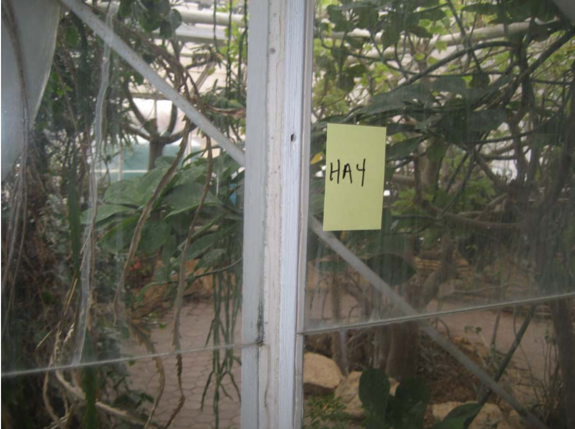
HA #4 – Non asbestos containing white window glazing
