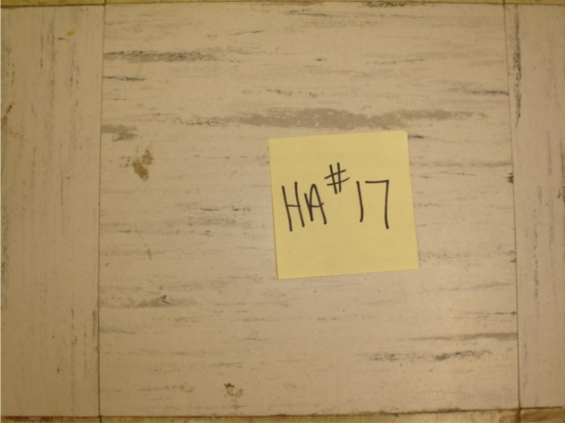
HA #17 – Non asbestos-containing 9” x 9” white floor tile with black streaks and associated asbestos containing mastic
