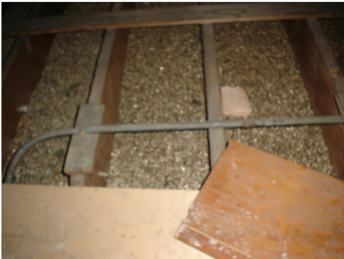
HA #30 – Non asbestos-containing attic insulation
