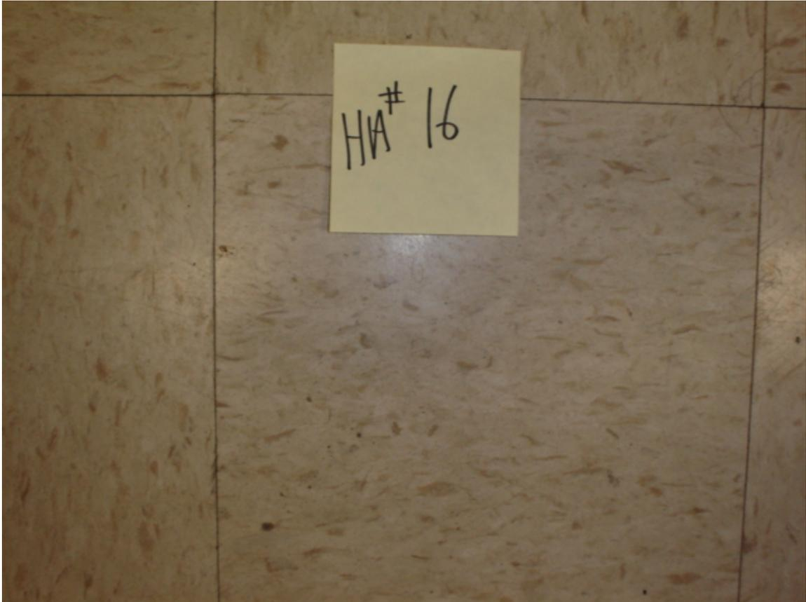
HA #16 – Non asbestos-containing 9” x 9” white floor tile with tan marble pattern and associated asbestos containing mastic
