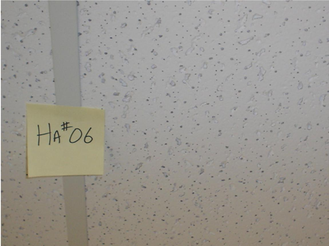
HA #6 – Non asbestos-containing 2' x 2' white lay-in ceiling tile
