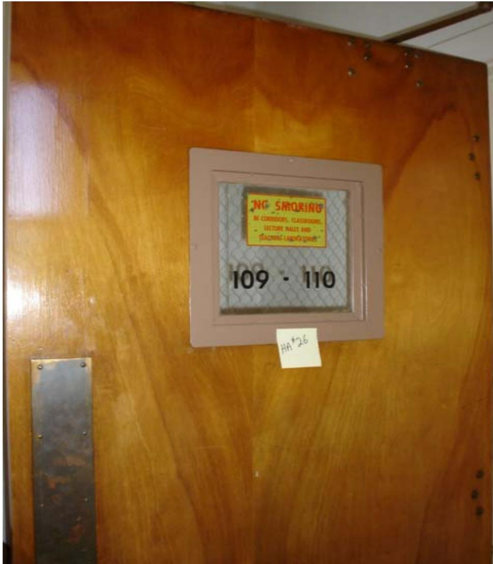
HA #26 – Assumed asbestos-containing fire door and frame
