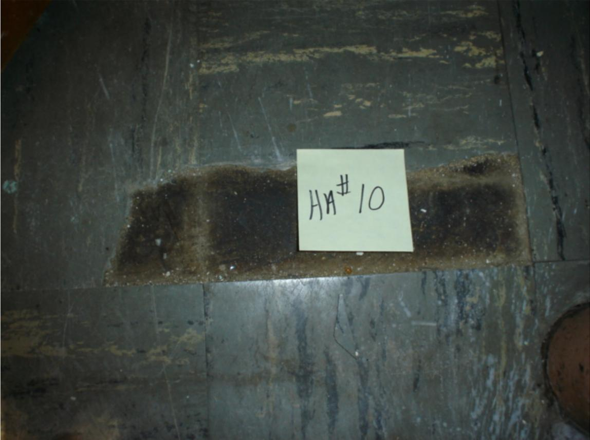
HA #10 – Asbestos-containing 9” x 9” gray floor tile with black and white streaks and associated non asbestos-containing mastic
