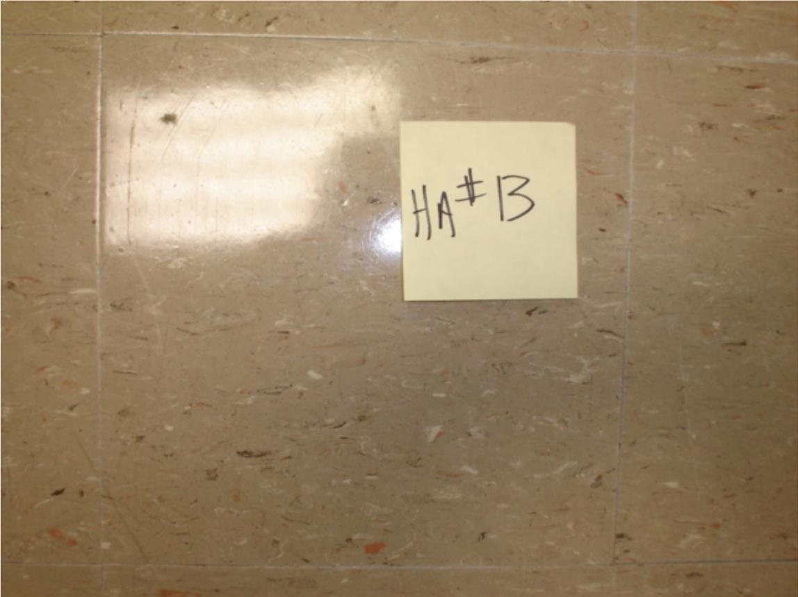
HA #13 – Asbestos-containing 9” x 9” beige floor tile with pink, white and brown streaks and associated non asbestos-containing mastic
