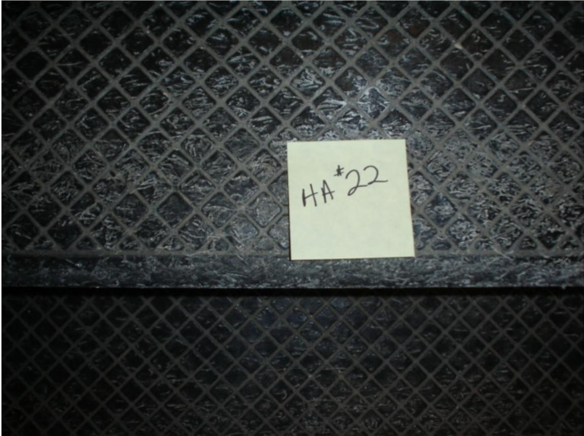
HA #22 – Non asbestos-containing black stair tread and associated mastic
