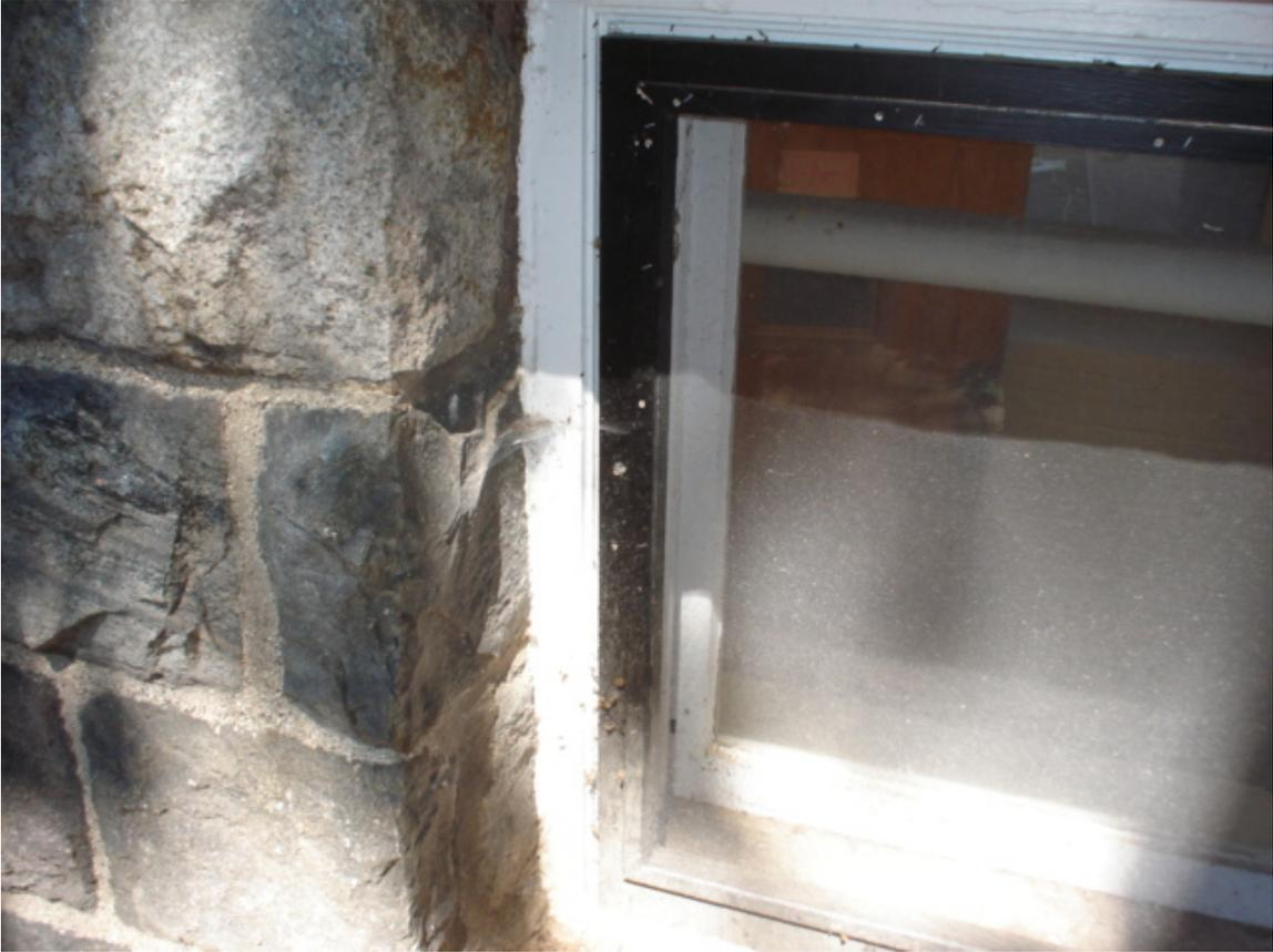
HA #27 – Assumed asbestos-containing window and door frame caulk compound
