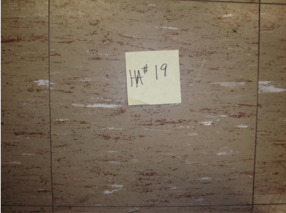
HA #19 – Asbestos-containing 12” x 12” tan floor tile with white and rust streaks and associated non asbestos-containing mastic
