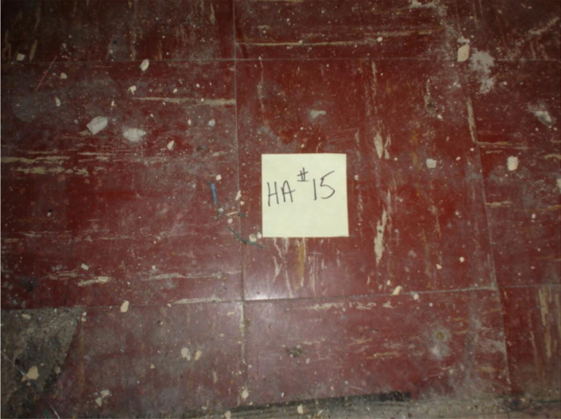
HA #15 – Asbestos-containing 9” x 9” red floor tile with cream streaks and associated non asbestos-containing mastic
