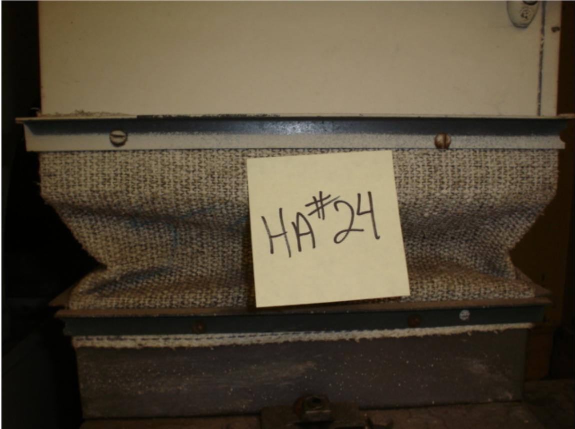
HA #24 – Asbestos-containing ventilation duct expansion cloth
