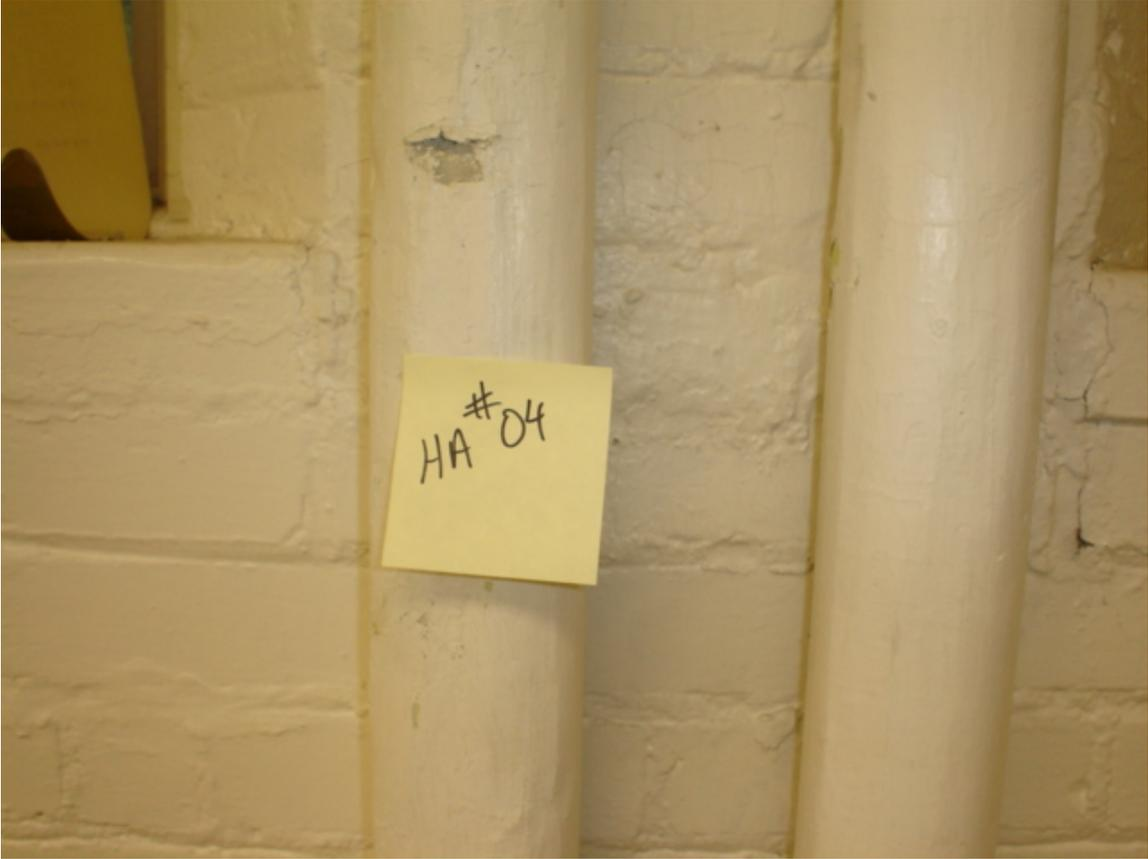
HA #4 – Asbestos-containing steam/condensate supply and return pipe straight insulation
