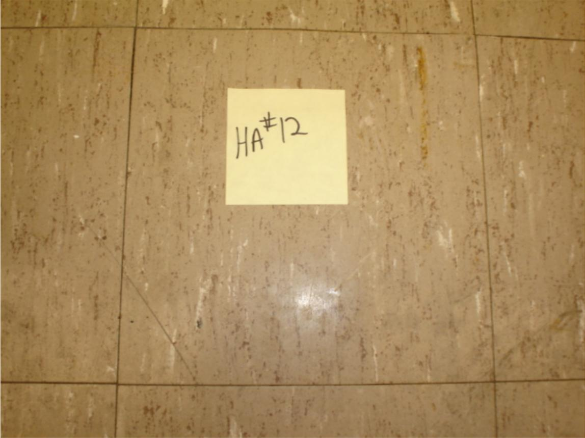
HA #12 – Asbestos-containing 9” x 9” tan floor tile with white and rust streaks and associated non asbestos-containing mastic
