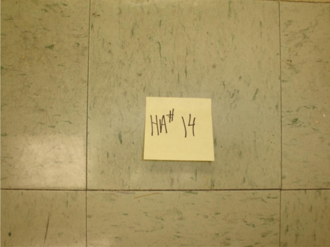
HA #14 – Non asbestos-containing 9” x 9” green floor tile with green streaks and associated asbestos-containing mastic
