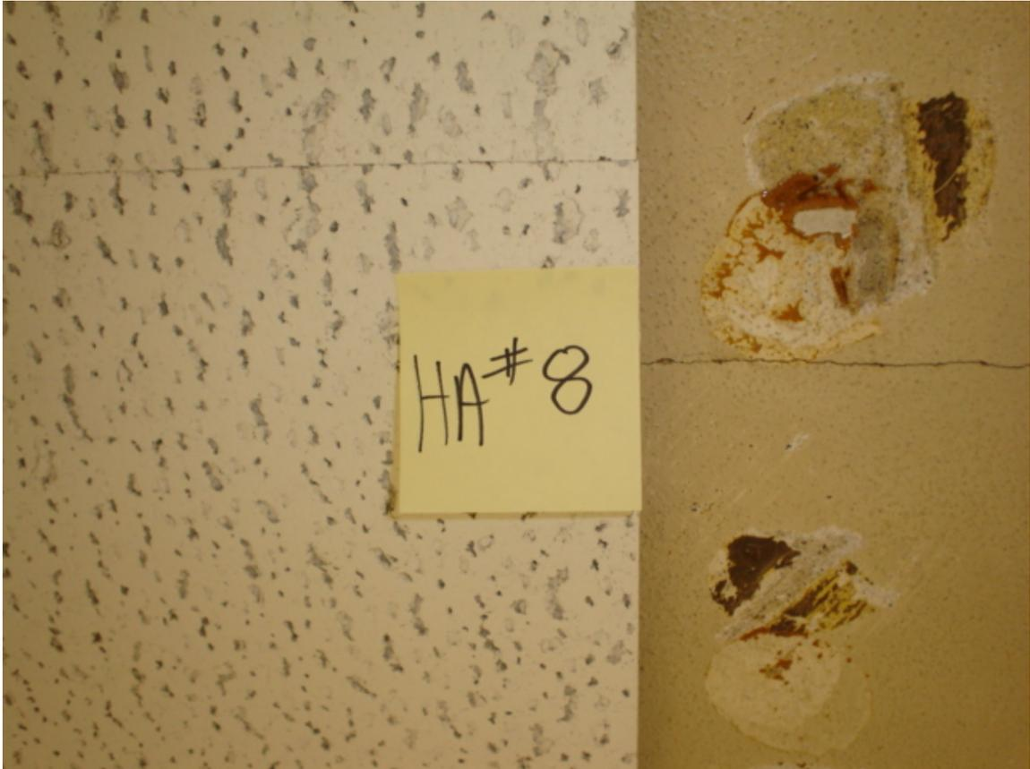
HA #8 – Non asbestos-containing 12” x 12” white ceiling tile with gouges and associated glue pods
