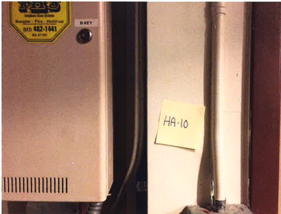
HA-10 Non-asbestos containing drywall
