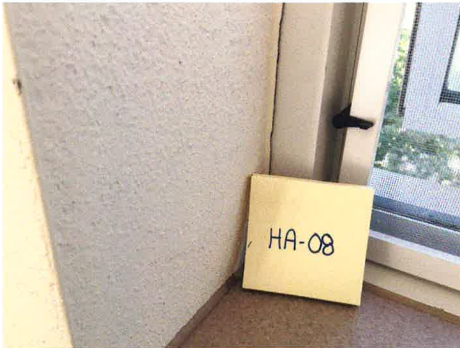
HA-08 Non-asbestos containing interior white window caulk
