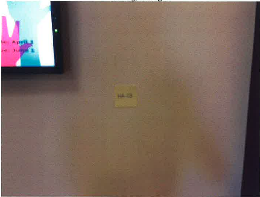
HA-03 Non-asbestos containing white textured wall plaster
