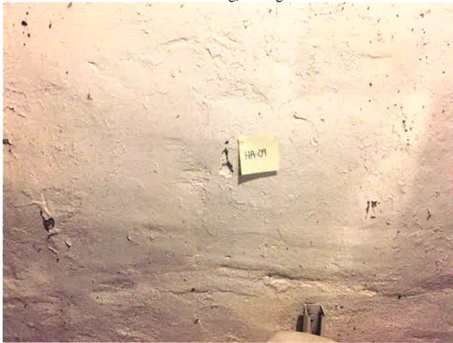
HA-09 Non-asbestos containing white rough texture plaster
