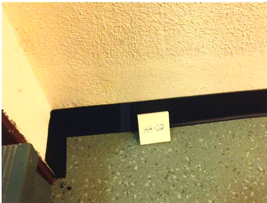
HA-02 Non-asbestos containing 4" black cove molding and associated mastic.
