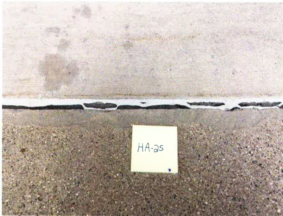
HA-25 Non-asbestos containing exterior gray front steps caulk
