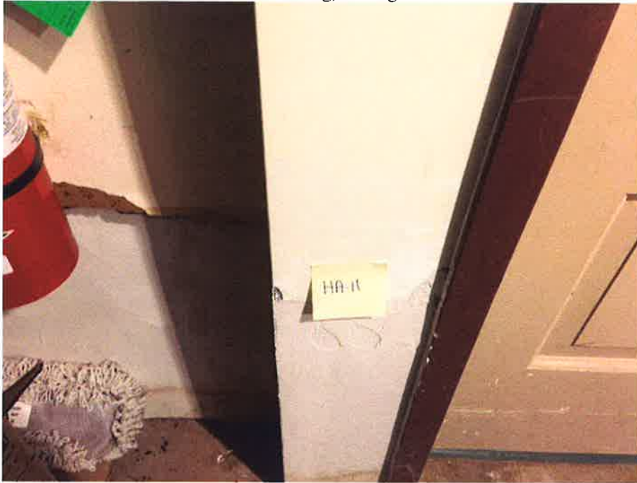
HA-11 Non-asbestos containing drywall joint compound
