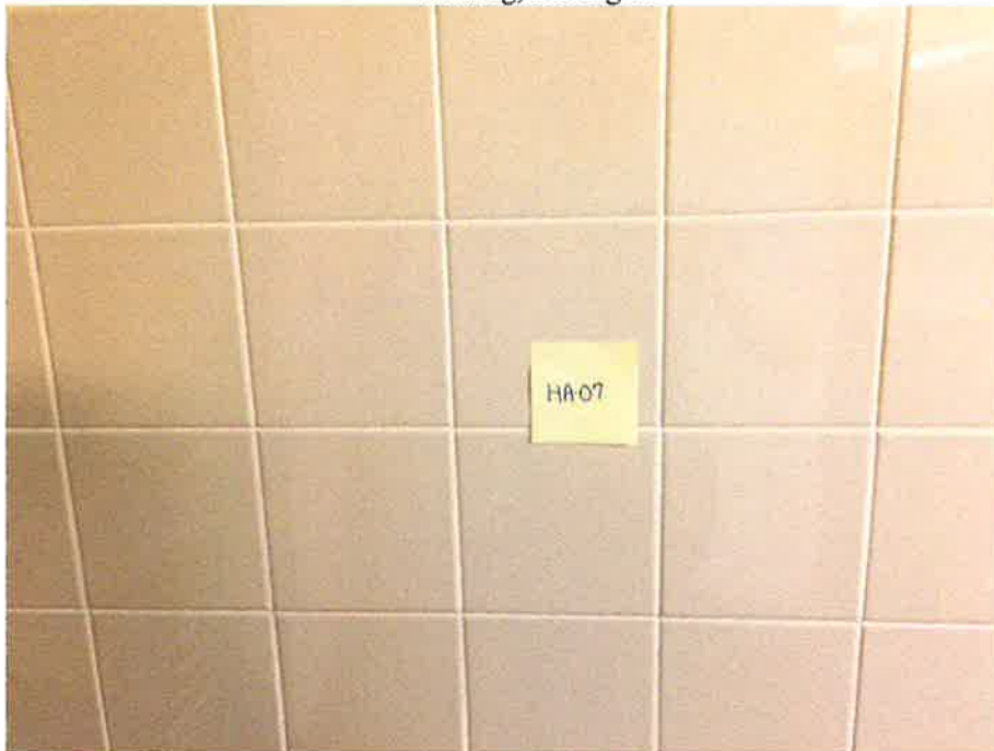
HA-07 Assumed asbestos-containing ceramic wall tile bedding compound and grout
