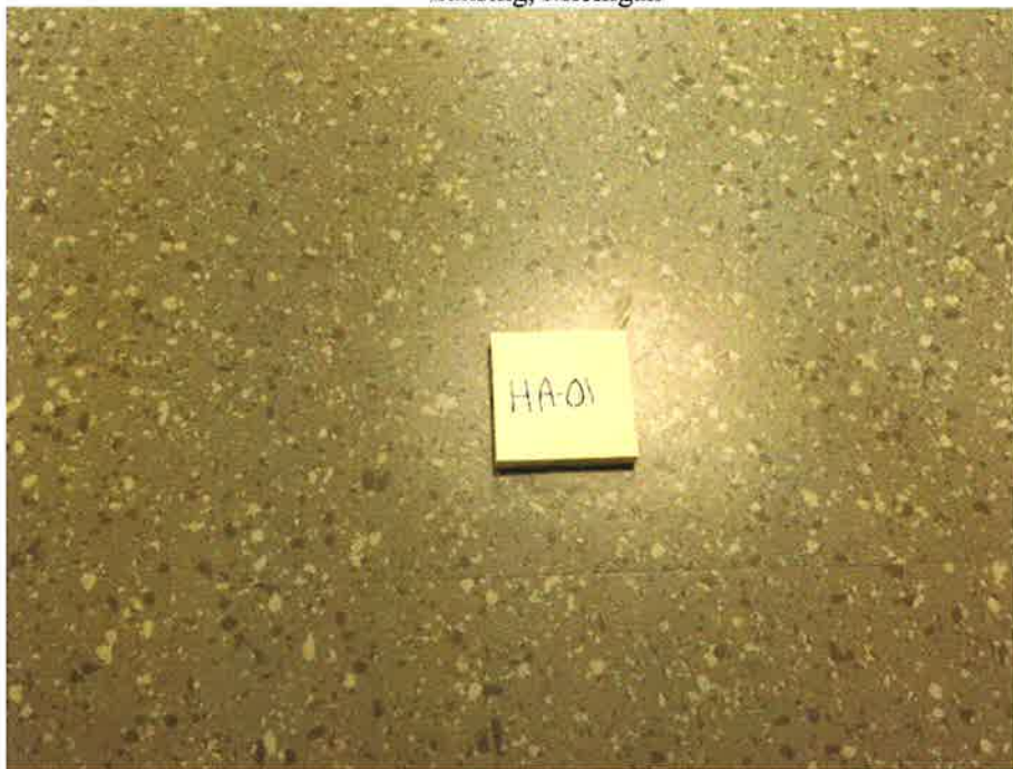
HA-01 Non-asbestos containing green linoleum with marble pattern and associated mastic
