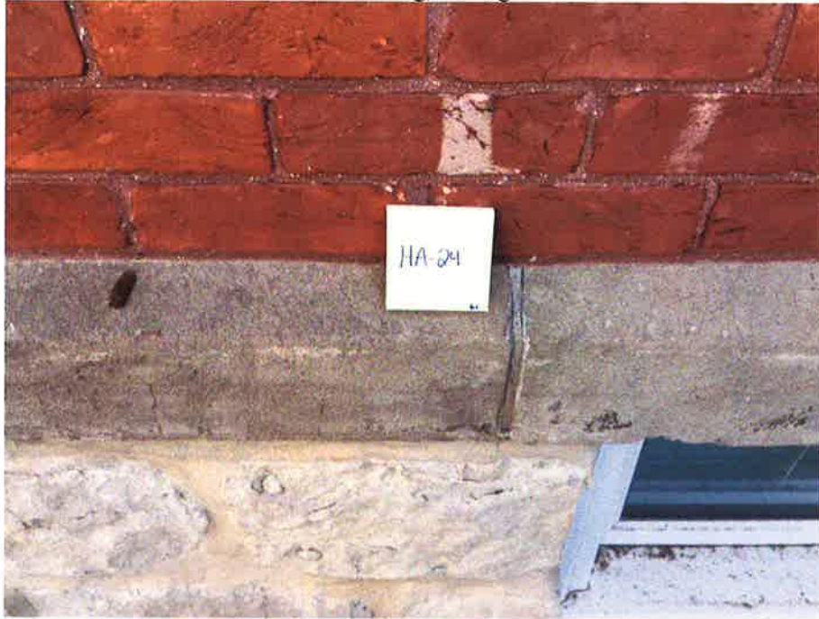
HA-24 Non-asbestos containing exterior brown building caulk
