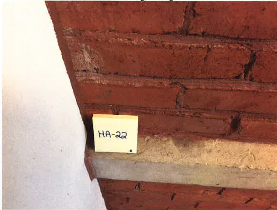
HA-22 Non-asbestos containing interior red brick caulk
