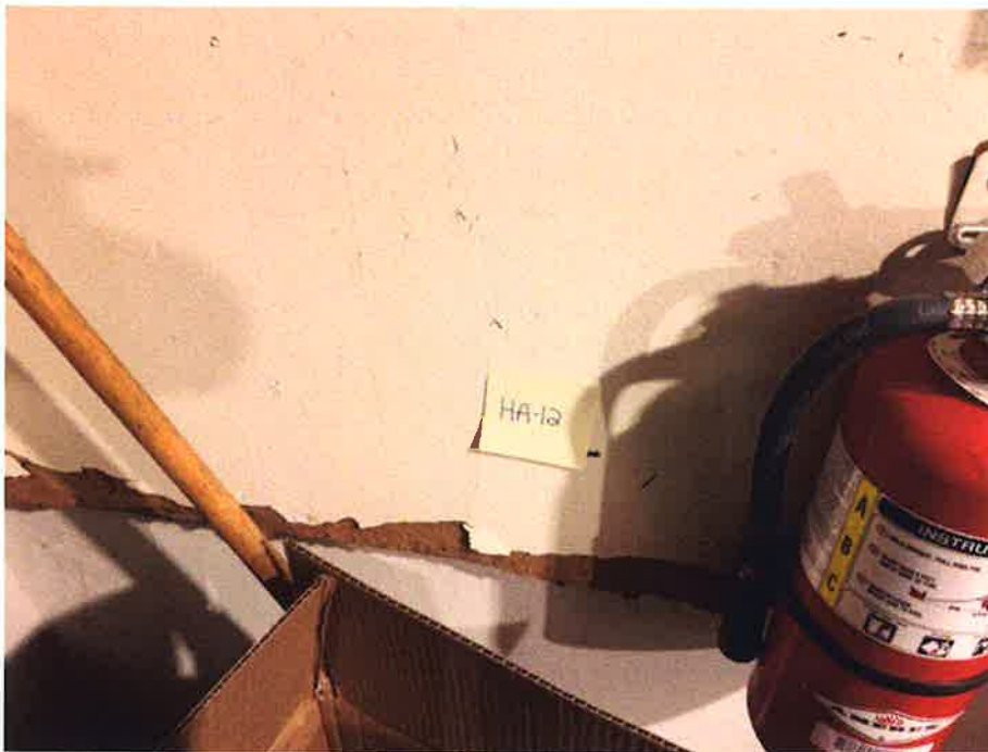
HA-12 Non-asbestos containing fiberboard wall panels and associated mastic
