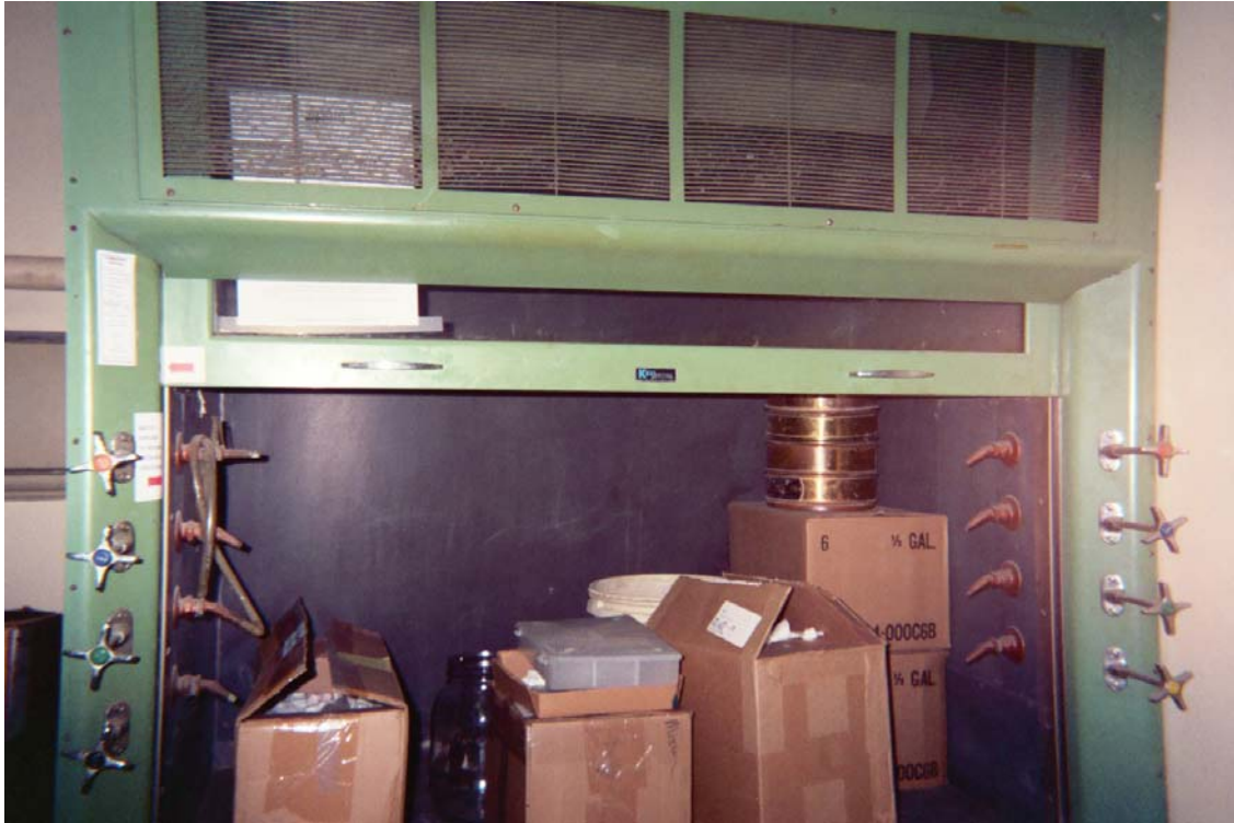
Photo 17 – Assumed asbestos-containing transite vent hood
