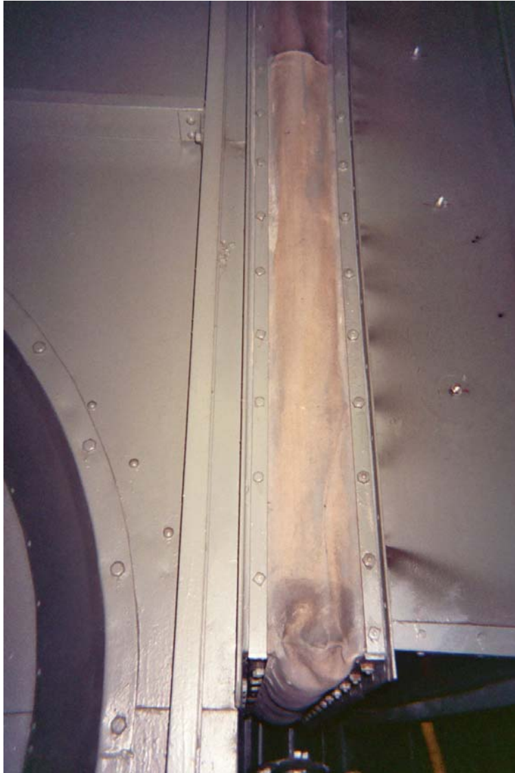
Photo 6 – Non asbestos-containing ventilation duct expansion cloth
