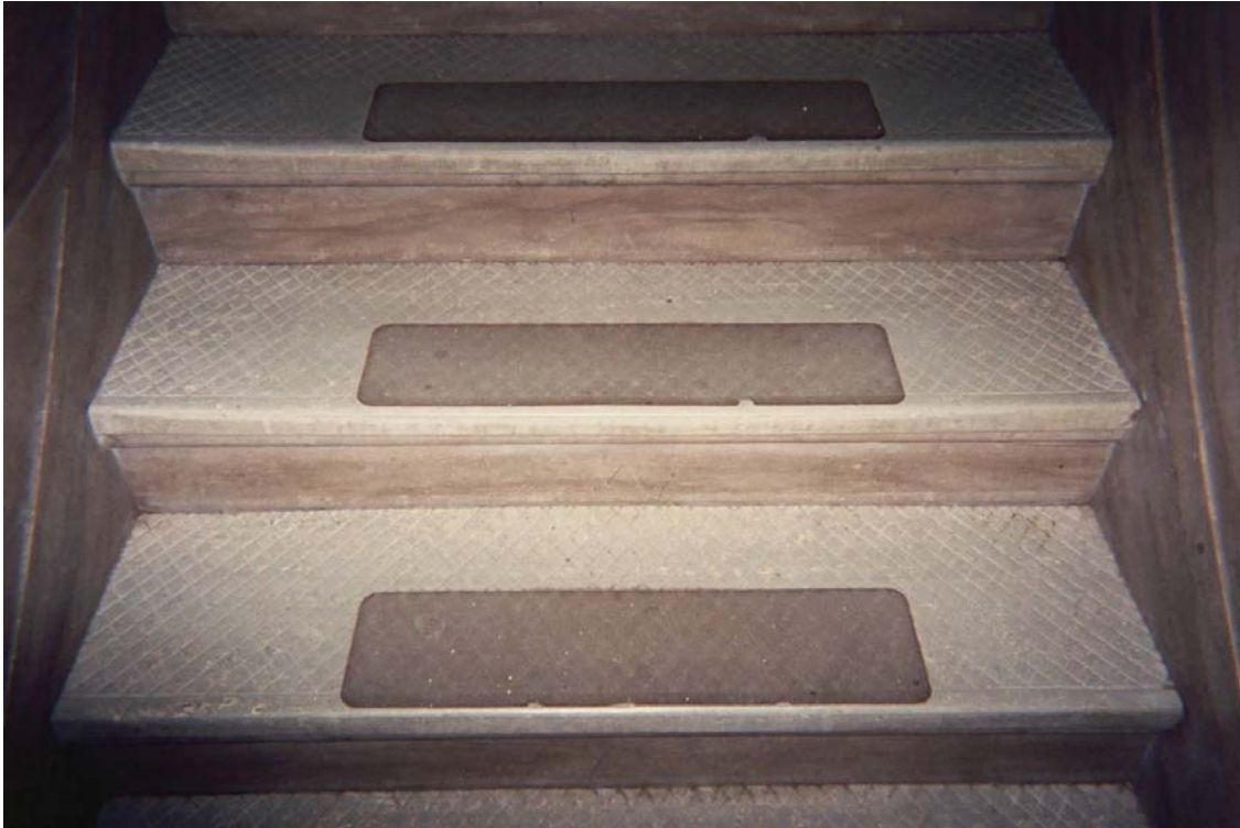
Photo 14 – Non asbestos-containing gray stair tread (associated mastic is asbestos-containing)
