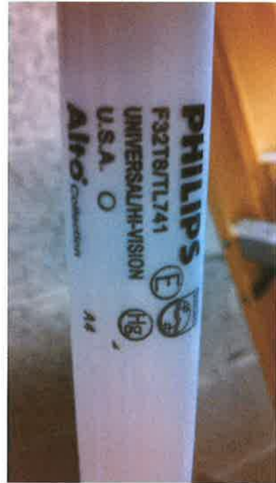
Energy efficient mercury containing fluorescent bulb used throughout
